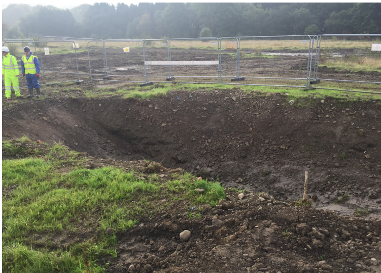
Early stages of excavation work for channel
