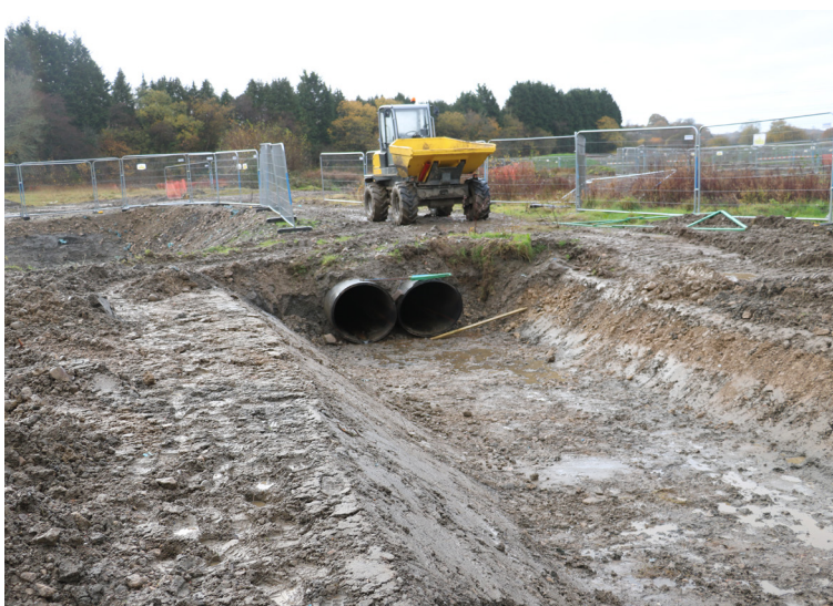
Pipework outflow leading into the new channel
