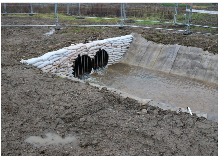
Bagwork headwall termination
