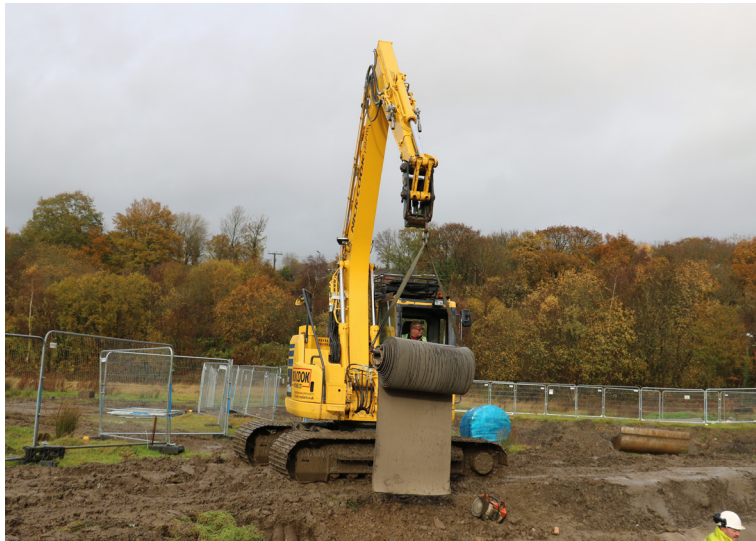
CC bulk rolls mounted to a spreader beam for easy deployment
