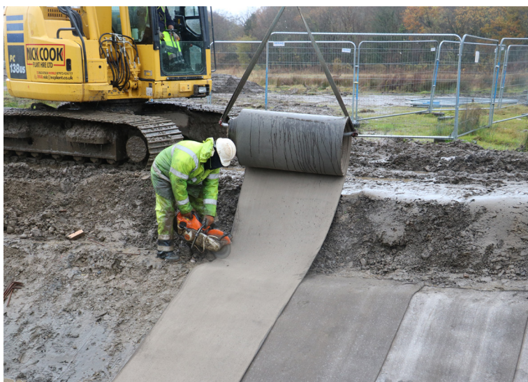
CC laid transversely and cut with a disc cutter
