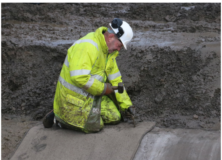
Material edges fixed within anchor trenches using ground pegs
