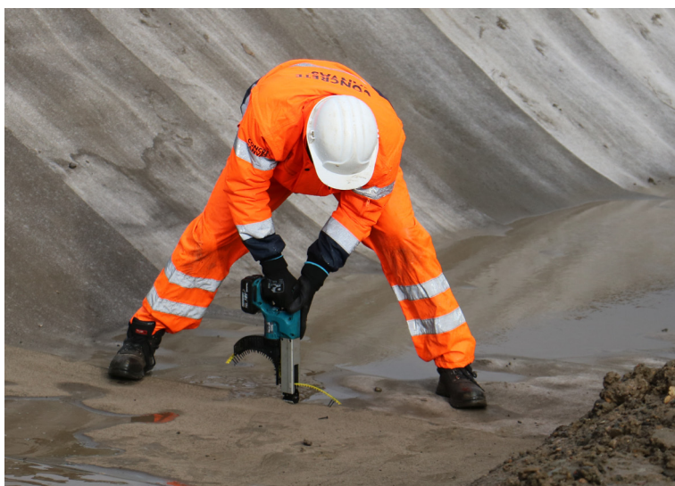
Overlaps were jointed using screws and an auto-fed screwdriver
