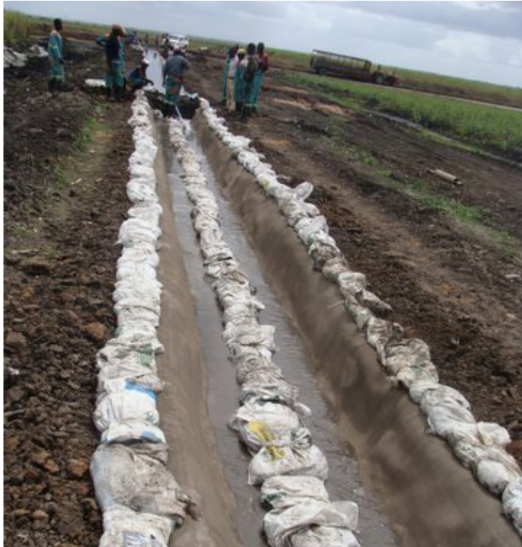
Sandbags were used to ensure flat edges and intimate contact with substrate
