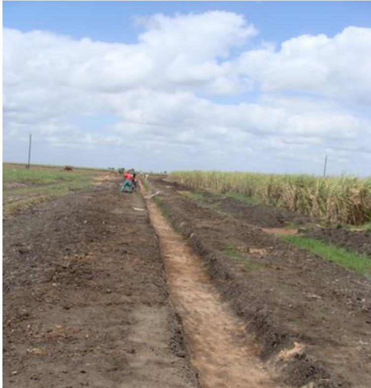
Original dirt canal
