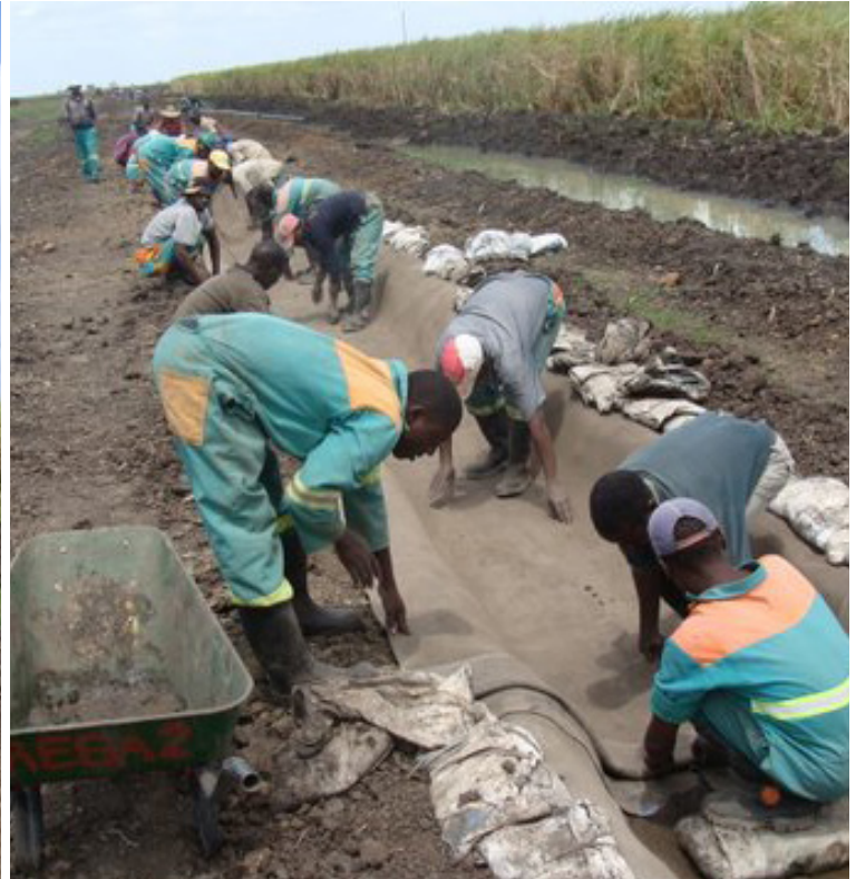
Installation of CC
