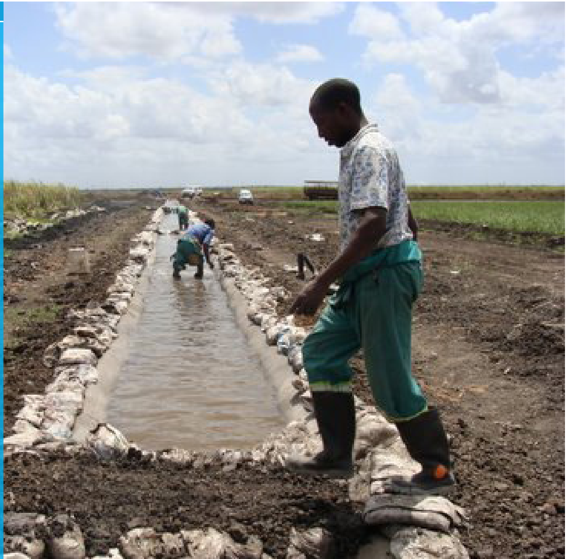
CC lined canal section with sandbags used to ensure flat edges.
