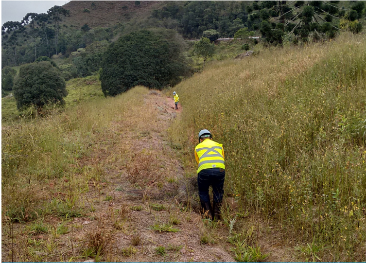
Removing vegetation from invert
