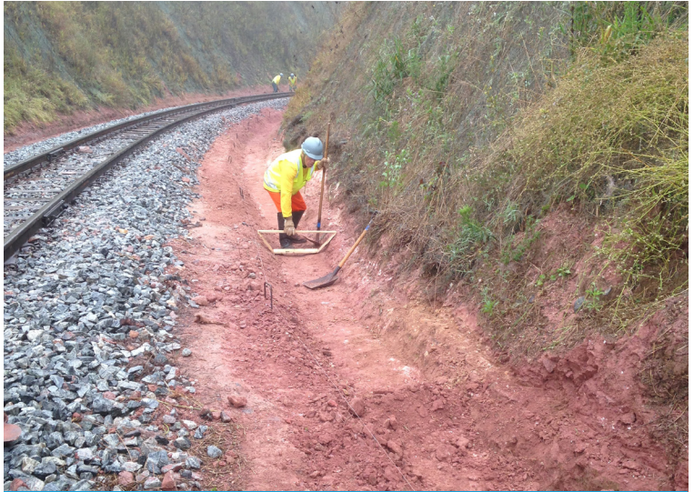
Grading channels
