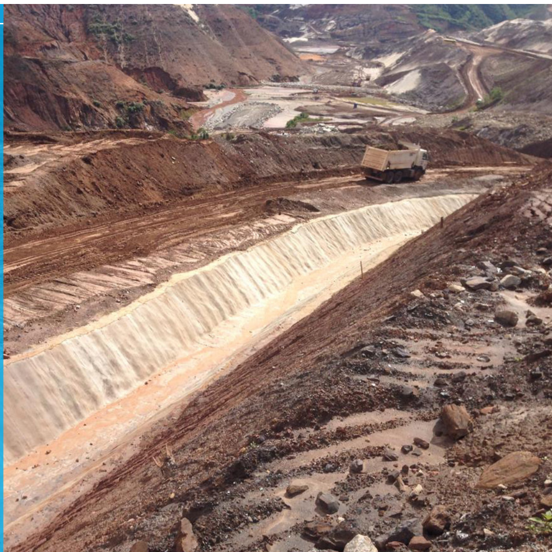
Completed channel section at a mine site in Mariana, Brazil
