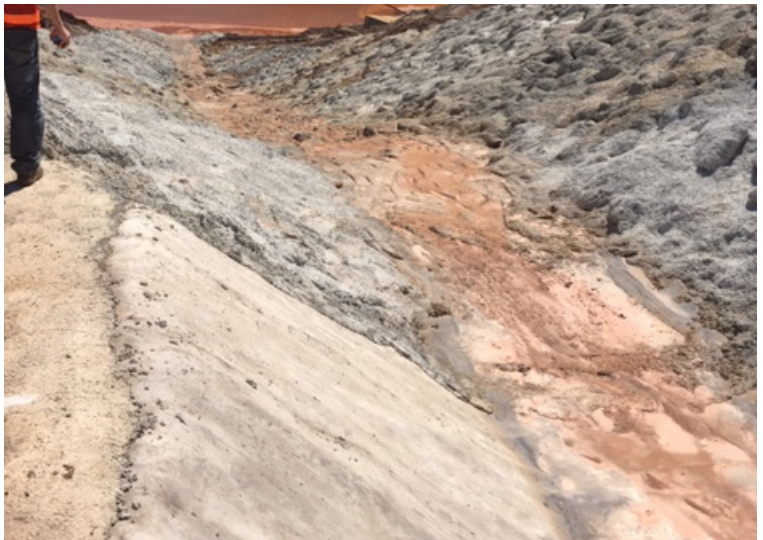
CC termination at rocky section of channel
