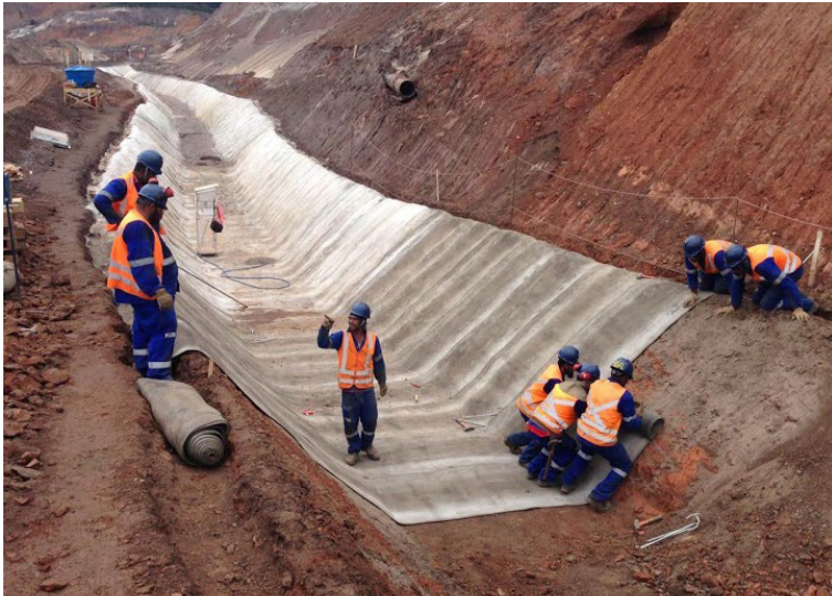
CC deployed transversely
