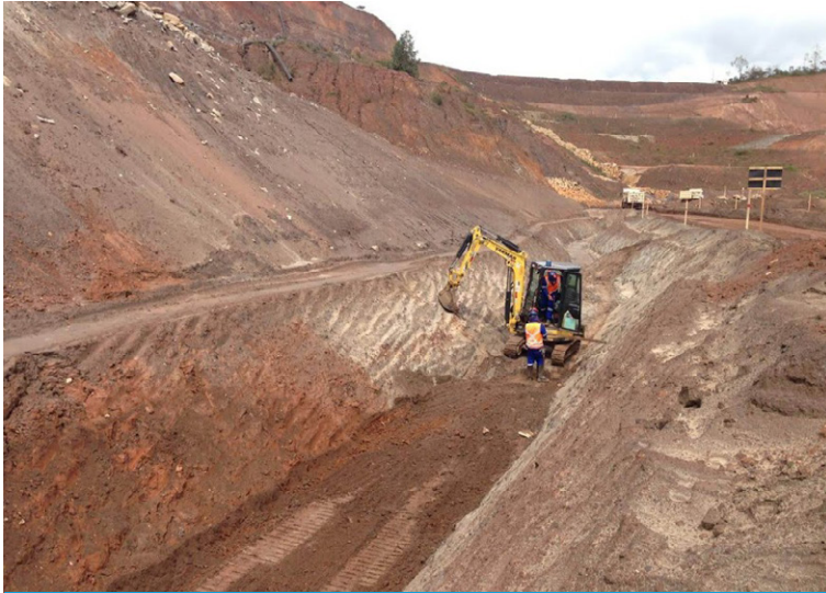
Excavation of 3m deep channel
