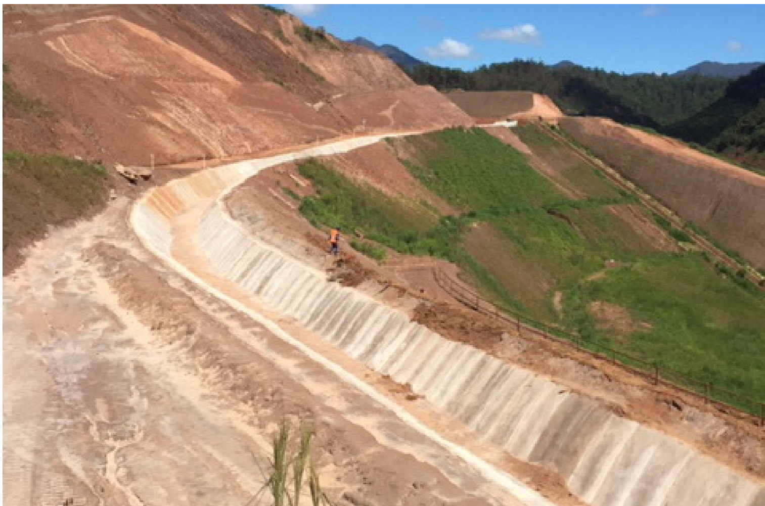
Completed channel and backfilling of anchor trenches using mortar
