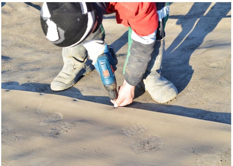
Joining overlaps with stainless steel screws
