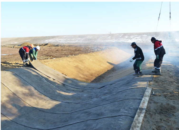
CC layers overlapped by 100mm
