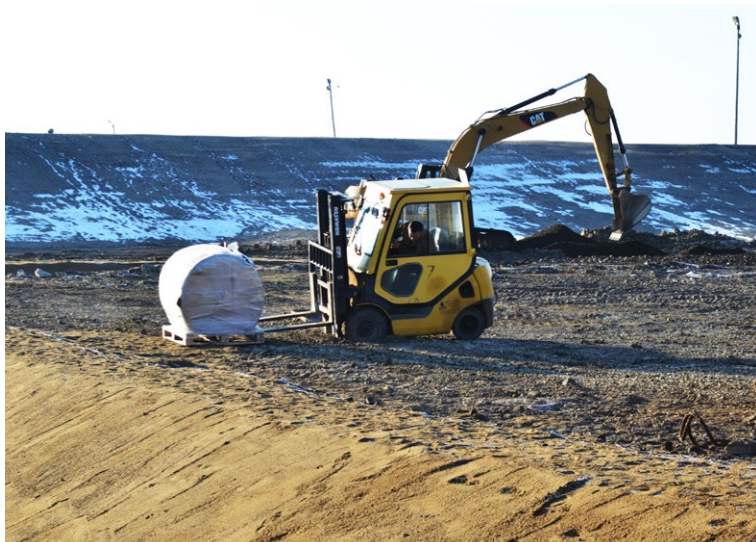
Bulk rolls of CC13™ were transported on site by forklift
