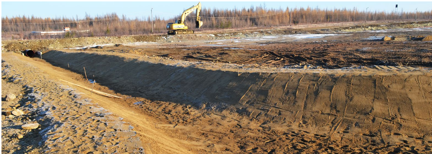
Channel following excavation
