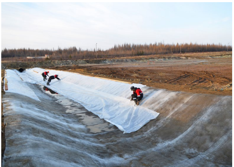
Covering CC with plastic sheeting to protect from frost
