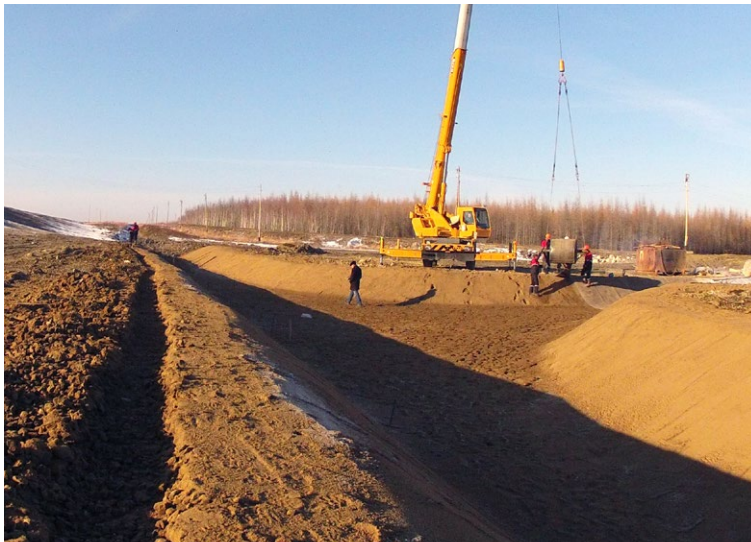
CC mounted onto a spreader beam and hung from a crane for deployment
