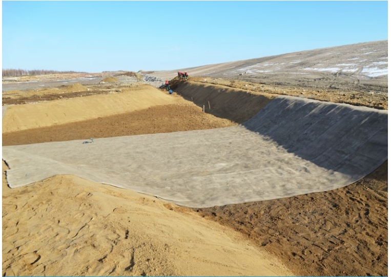
CC laid transversely across the channel
