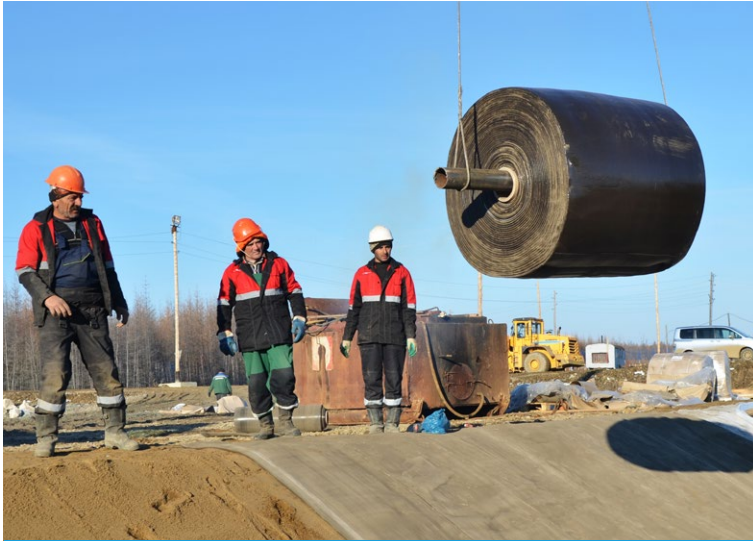
Bulk roll of CC13™ lowered into position for deployment
