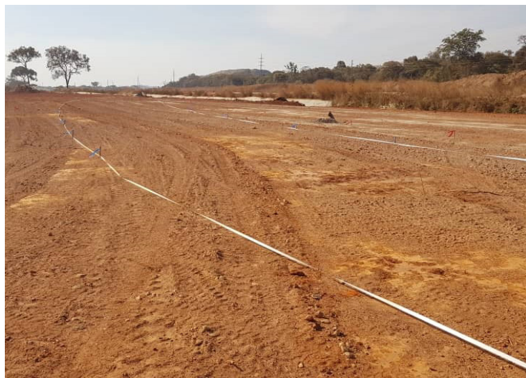
Channel marked out prior to ground works
