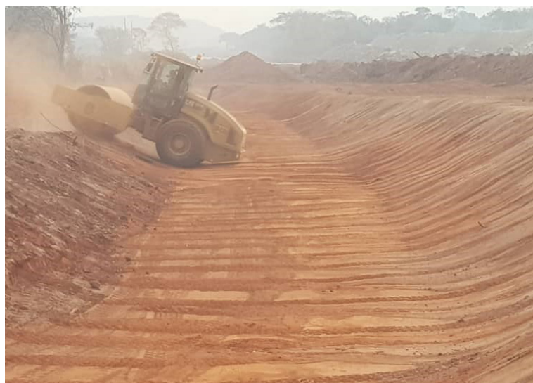
Compacting substrate following excavation of side slopes
