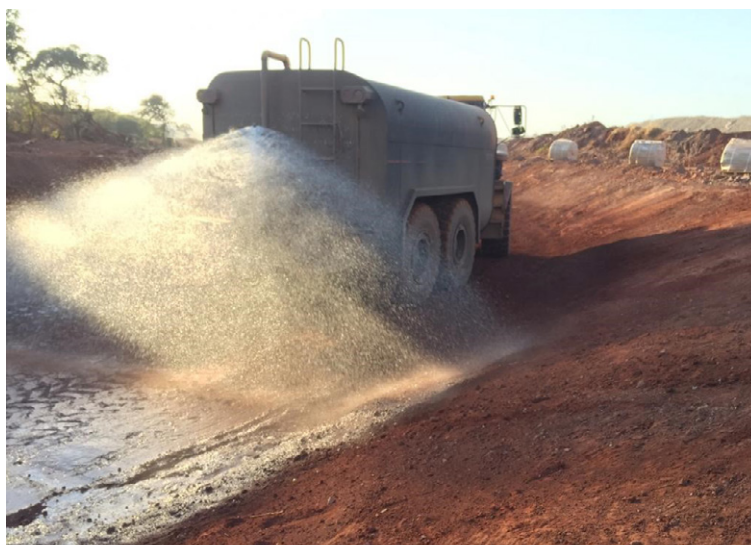
Moistening substrate prior to installation
