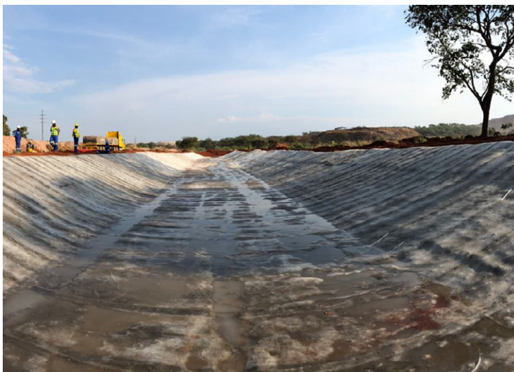
Completed channel section following hydration
