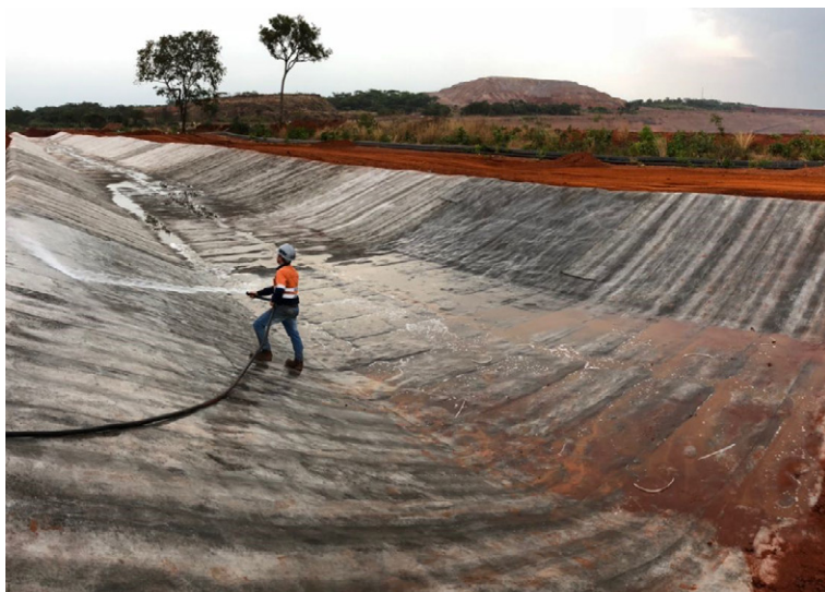
Hydration of material at end of work day
