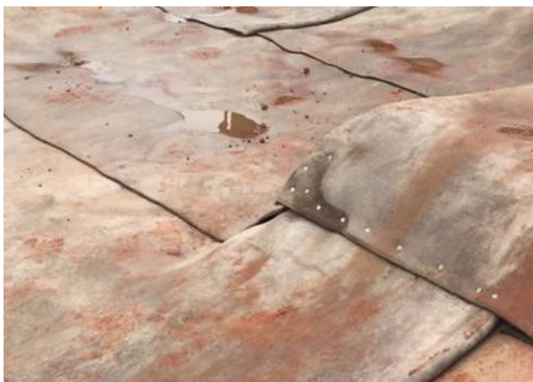
CC layers jointed using screws at corner section
