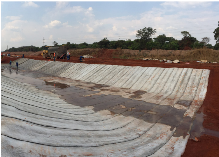
CC was laid transversely, using an excavator and spreader beam
