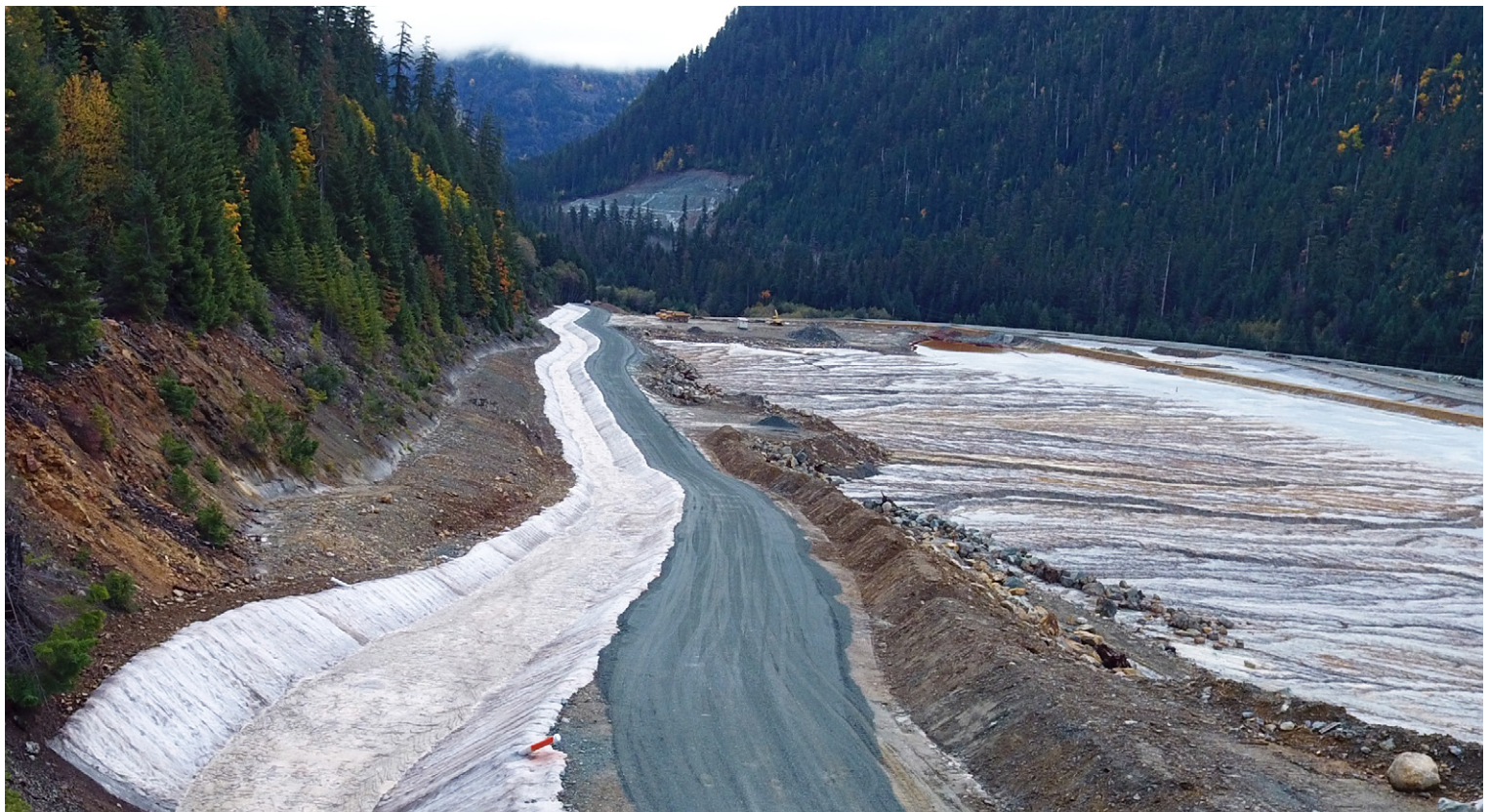
Aerial view of the mouth of the channel showing transition anchor trench
