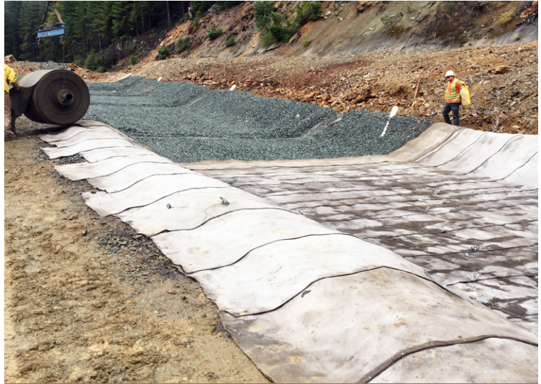
Anchor trench prior to backfilling
