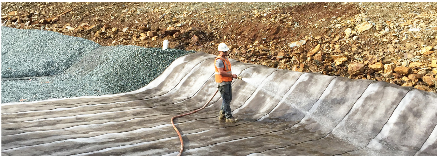
Hydration of the CC layers. CC run-off did not require treatment prior to discharge into the local water course
