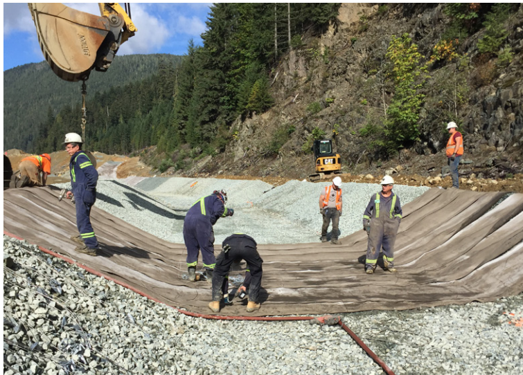
Screwing overlapped joints at 150mm centres
