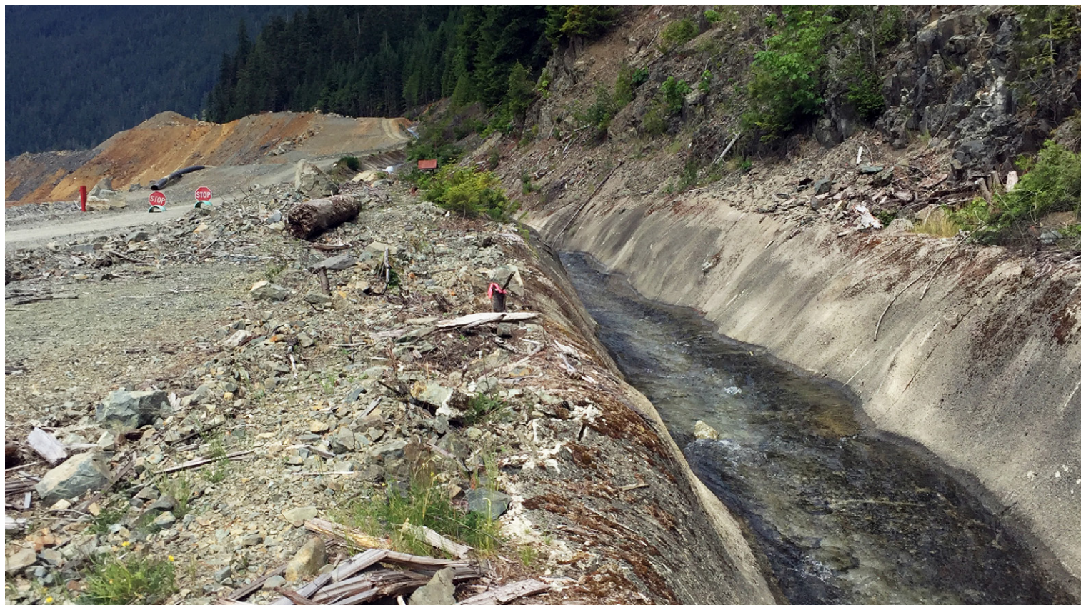
Previous channel section originally lined with shotcrete and showing signs of degradation
