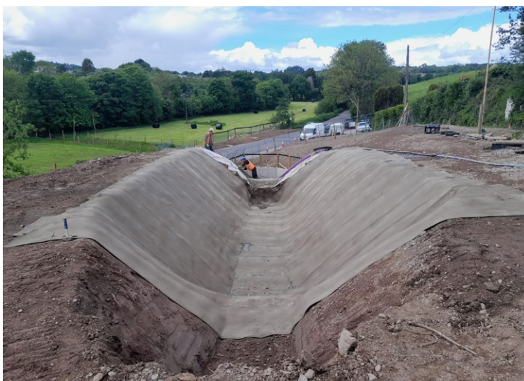
CCT2™ material laid transversely
