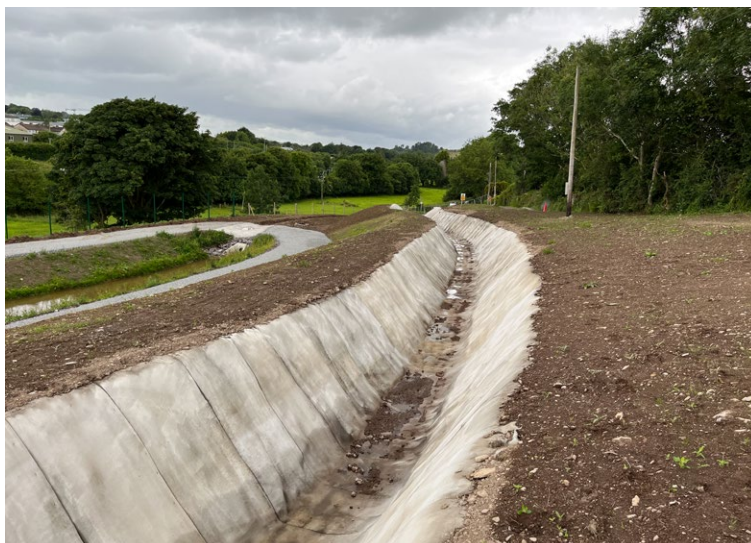
Anchor trenches backfilled
