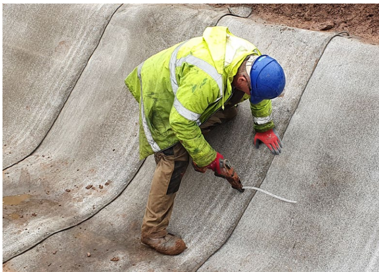
CC layers secured together at 200mm intervals
