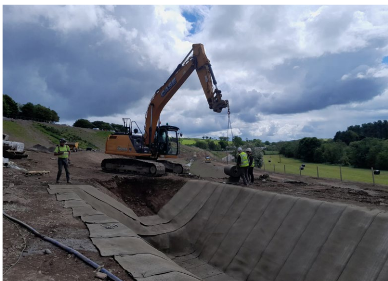
CCT2™ Bulk Rolls deployed using spreader beam
