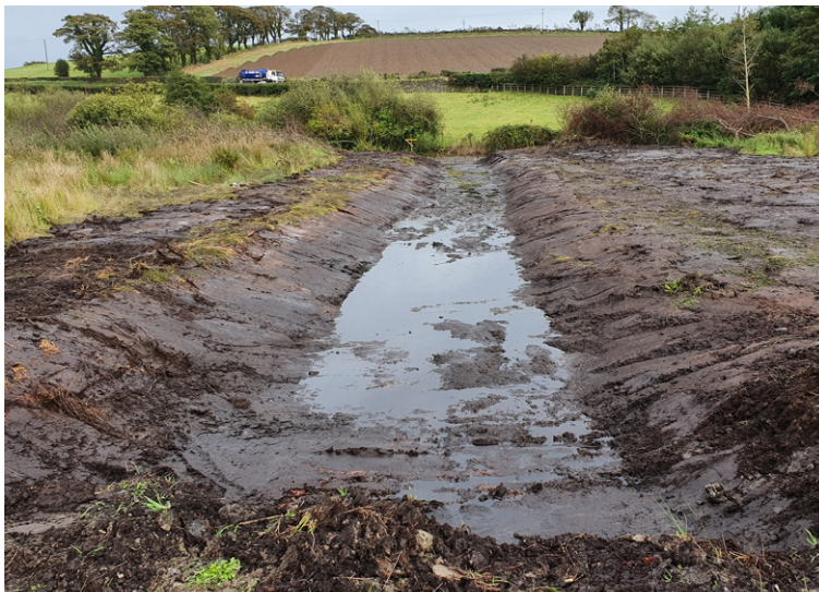
Saturated ground following excavation
