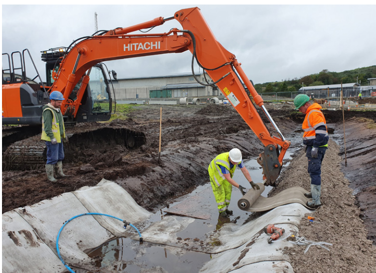
Deploying CC transversely across channel
