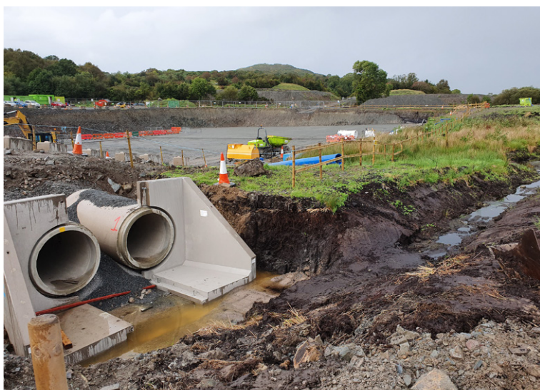
Precast headwall with 1200mm twin pipes on upstream side
