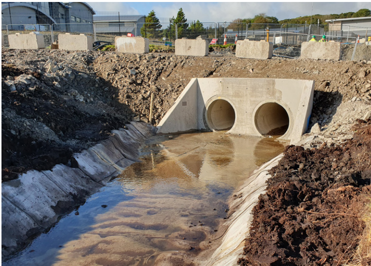
Headwall section completed
