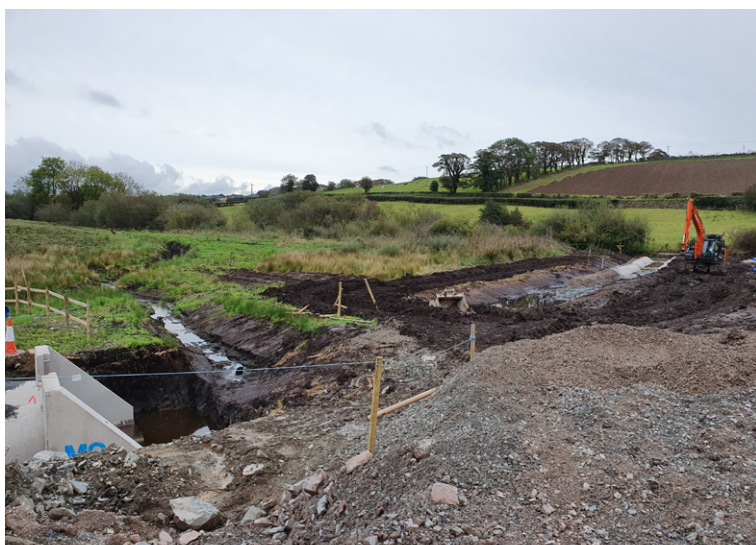
Temporary diversion channel excavated to divert water
