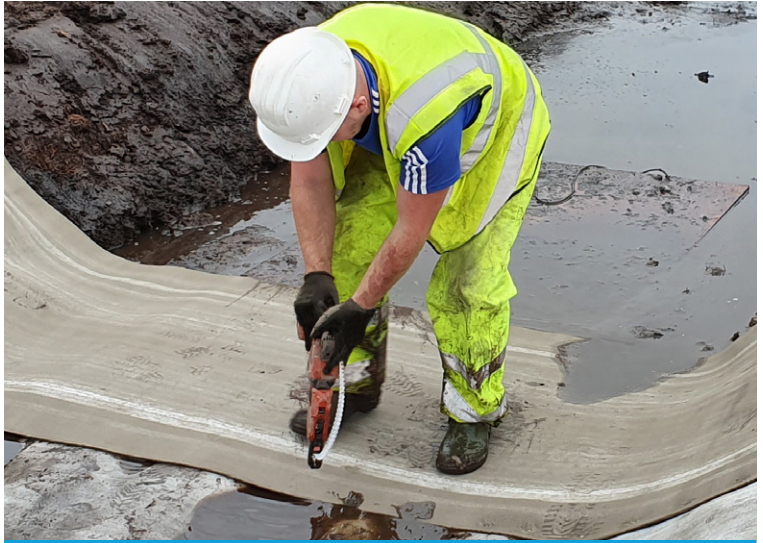
Screwing joints & pinning CC into anchor trench
