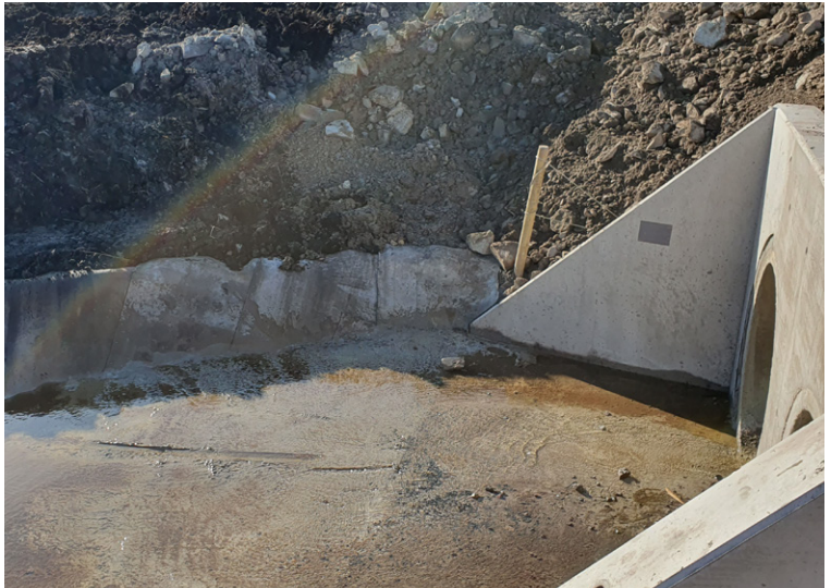
Precast headwall & CC interface
