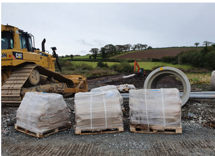
CC8 batched rolls delivered to site
