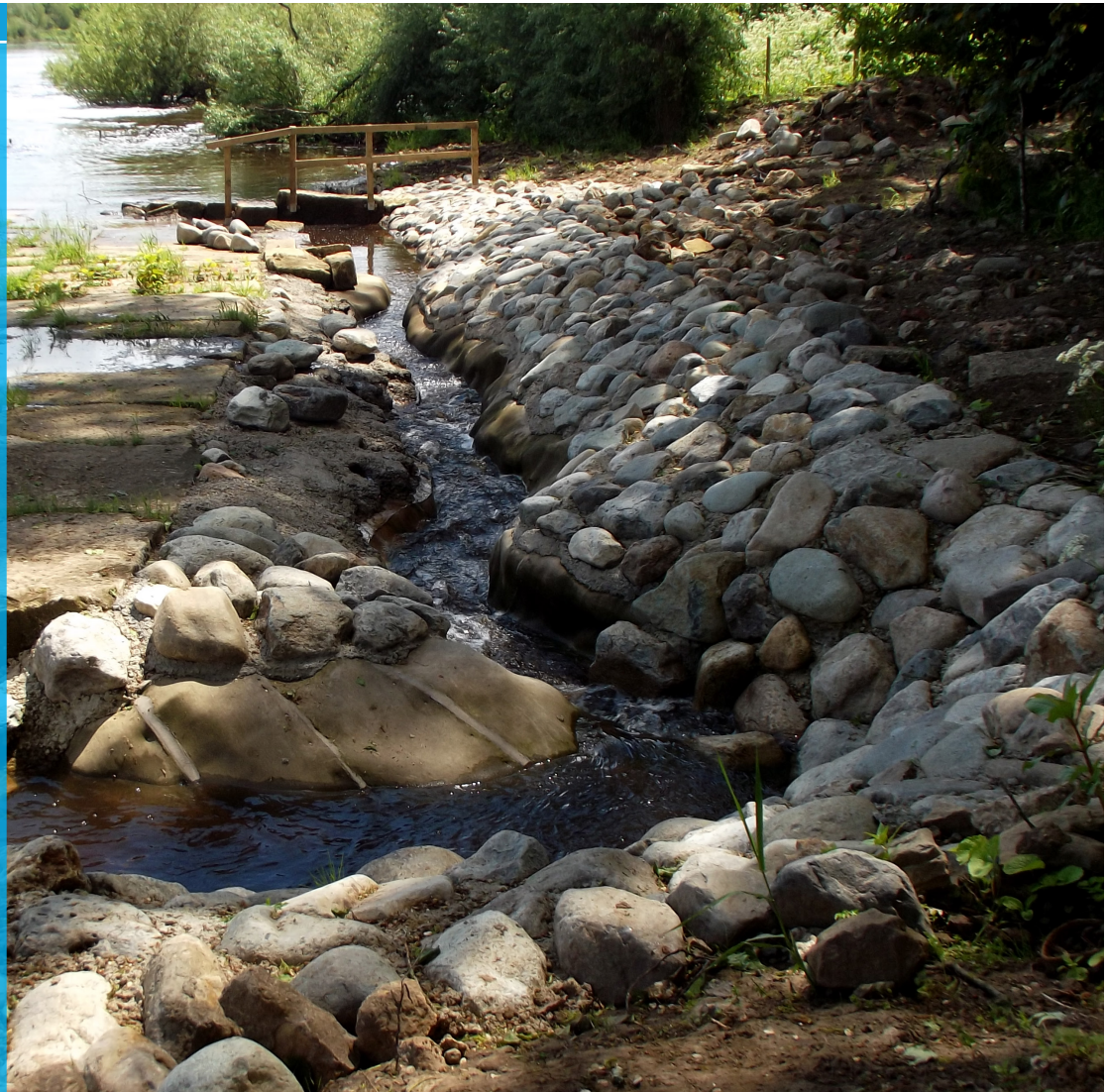
Section of completed installation at the Naburn Weir eel and lamprey pass
