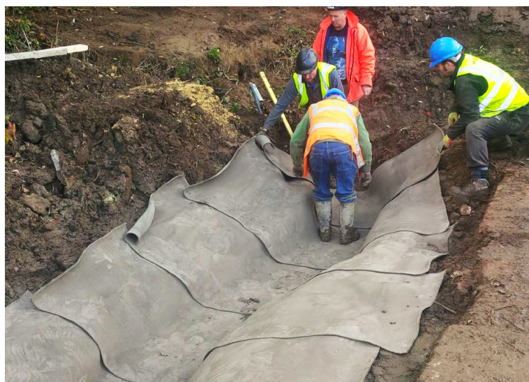
Installation of transverse CC layers
