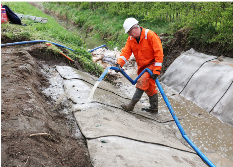
Hydration of the upper sections of CC
