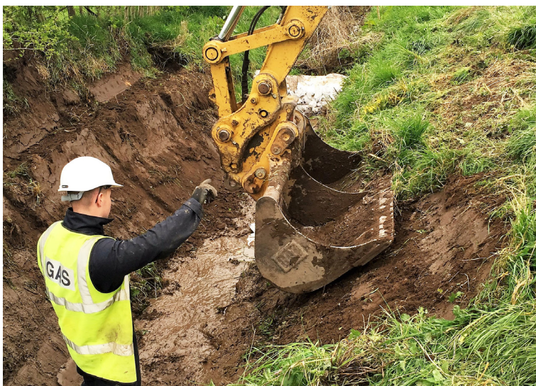
Grading of the profile
