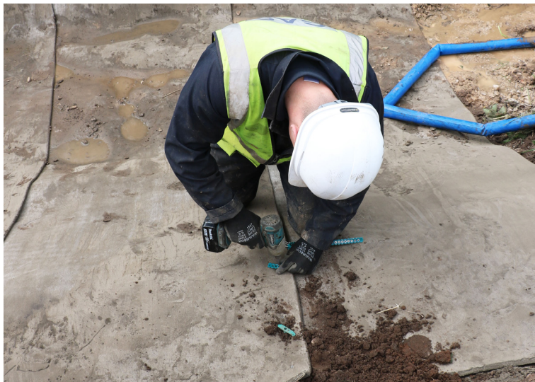
Screwing of the overlapped layers of CC
