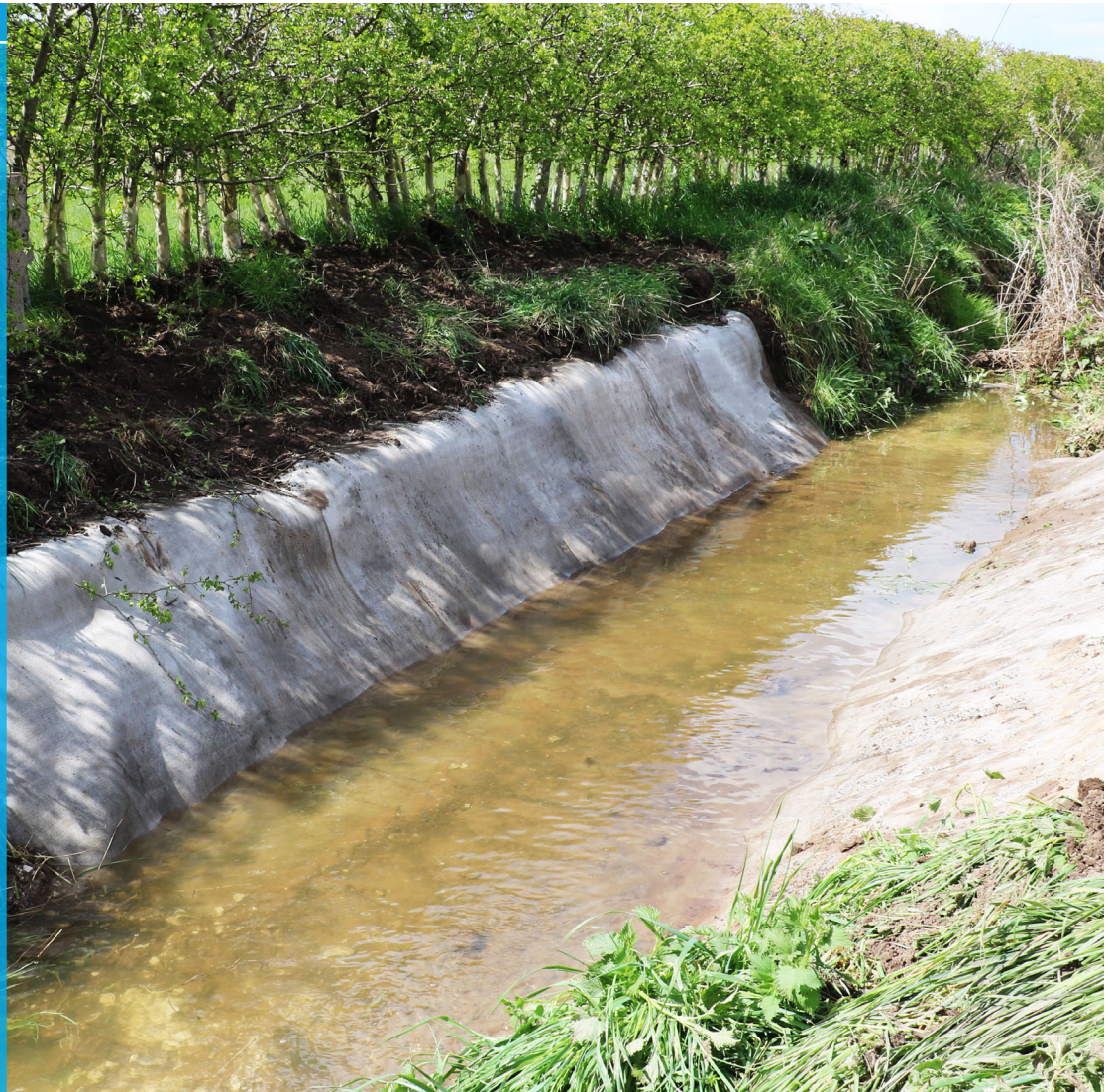
Completed CC lined drainage channel above pipe crossing
