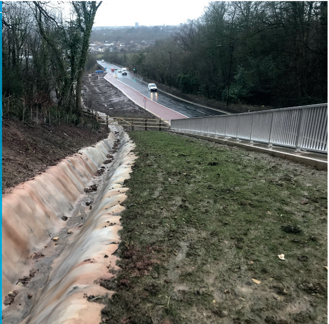
CC8™ used to line a crest drainage channel along a newly constructed retaining wall
