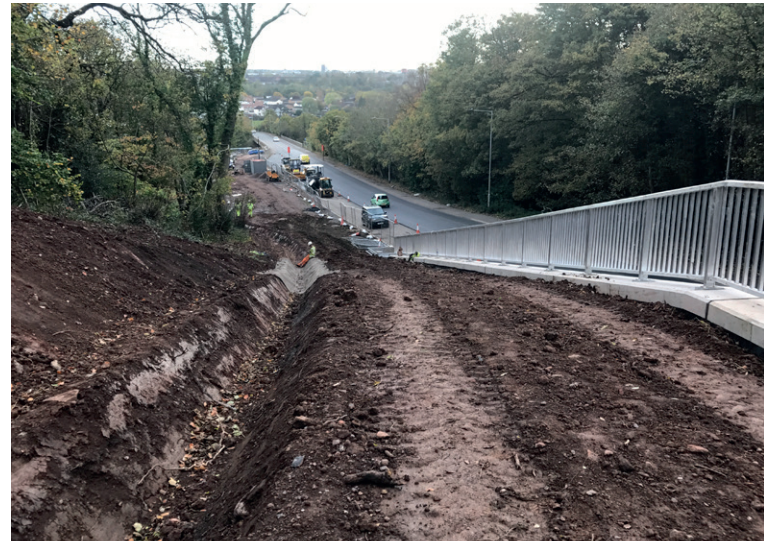
Ditching bucket used to create channel profile
