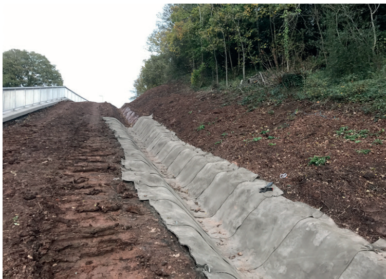
CC installed behind retaining wall working upstream
