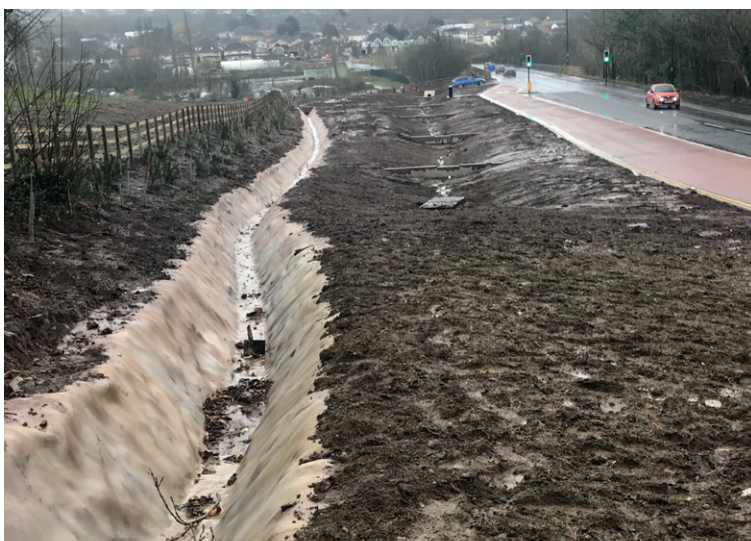
Swale constructed in front of CC channel to collect highway surface water
