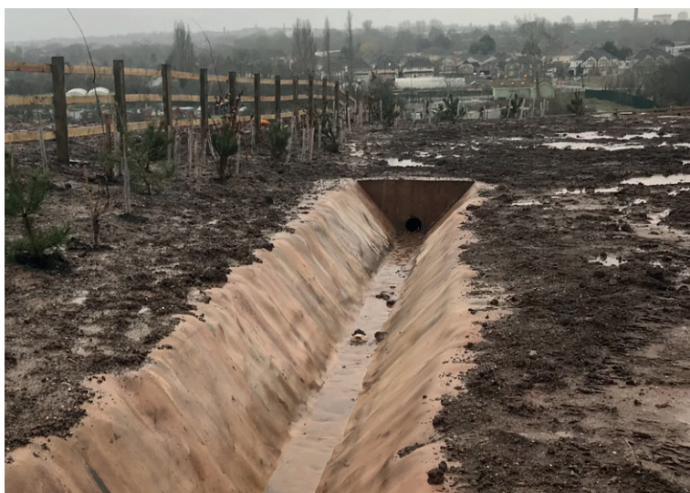
CC terminated into concrete headwall
