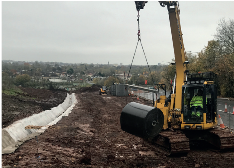
Bulk rolls of CC8™ were deployed from a spreader beam and excavator
