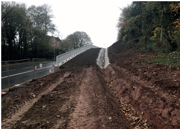
Completed CC channel behind retaining wall
