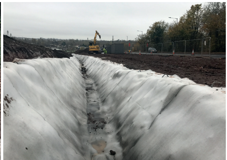
CC was hydrated at the end of each installation stage
