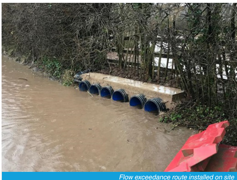
Super gullies were installed to help channel excessive water during flood events
