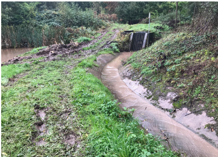
Existing concrete lined section of channel
