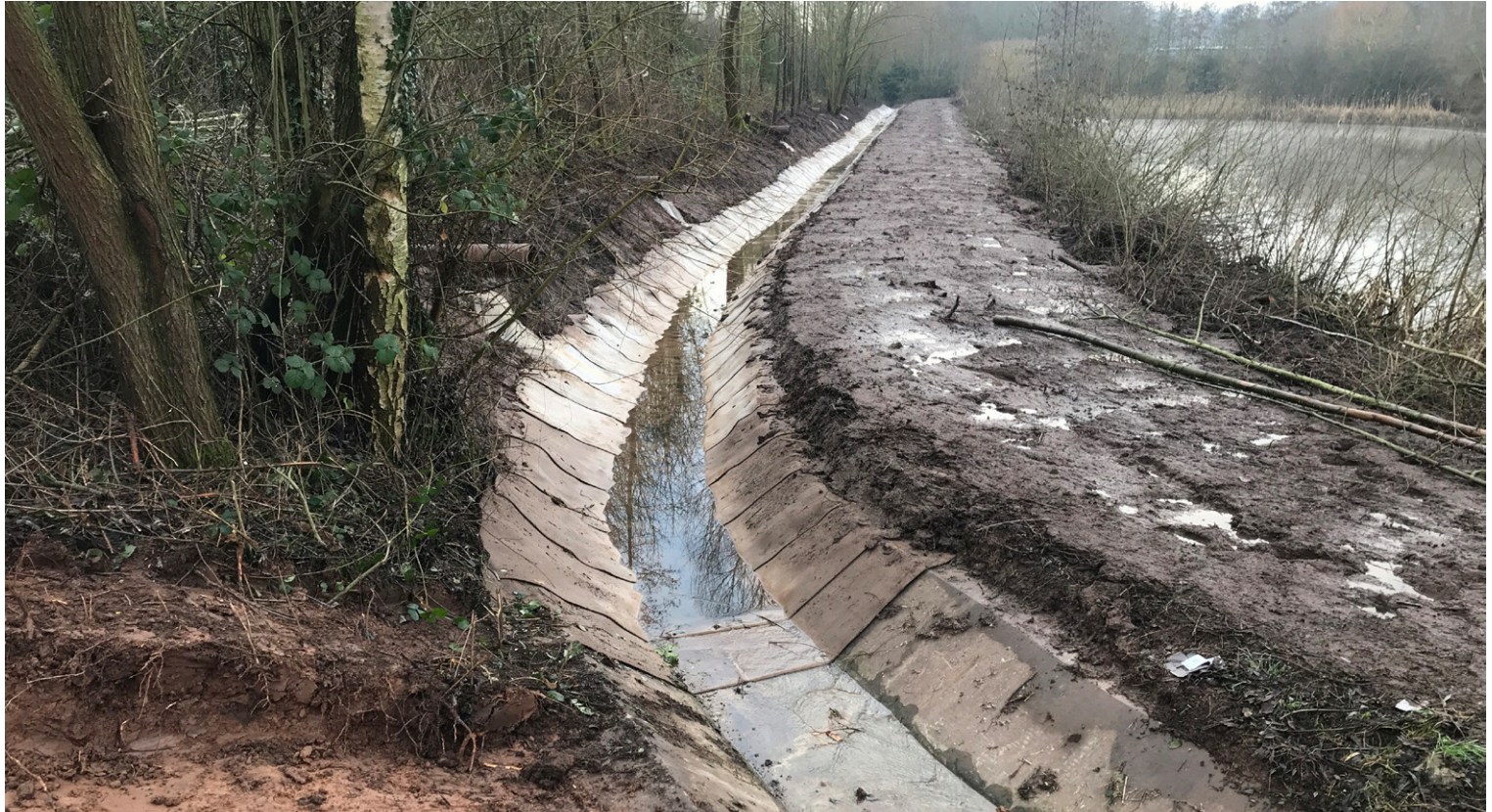
CC terminating against existing concrete channel section
