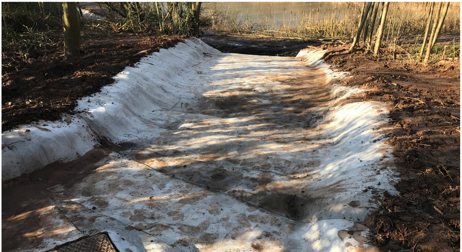
CC lined spillway area leading from newly installed flow exceedance pipes
