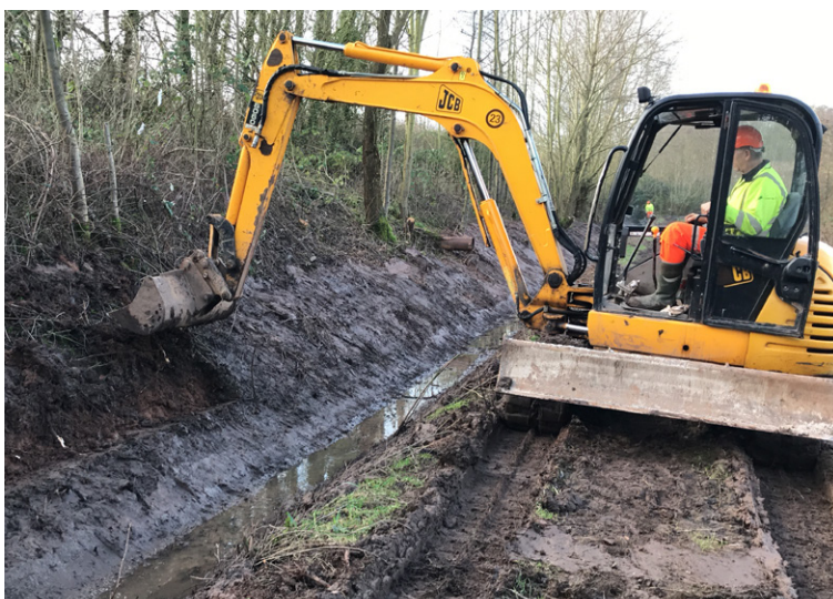
Reprofiling of the existing channel prior to installation
