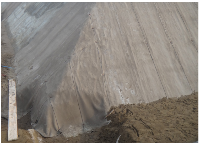
CC edges buried at the toe
