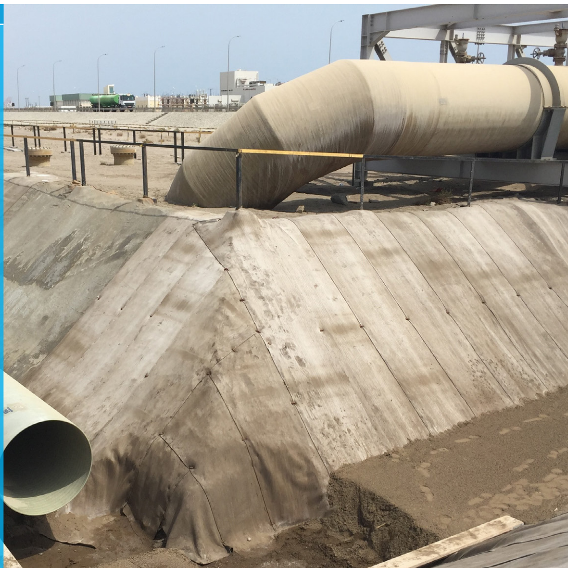
Completed section of CC lined channel wall
