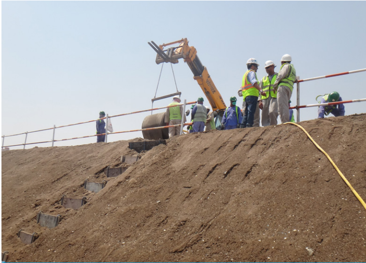
Channel wall prior to lining
