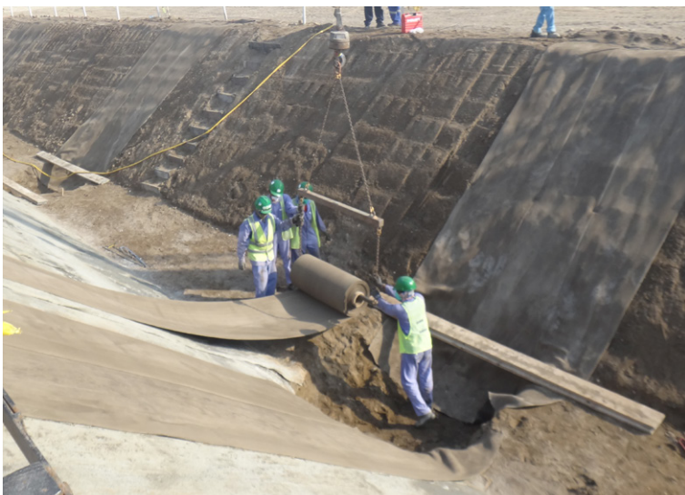
CC depoyed from spreader beam
