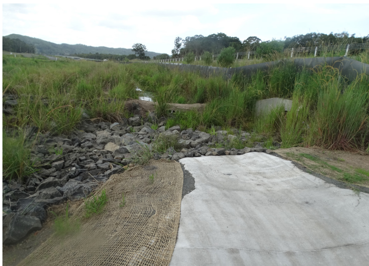
CC edges were captured within anchor trenches and backfilled
