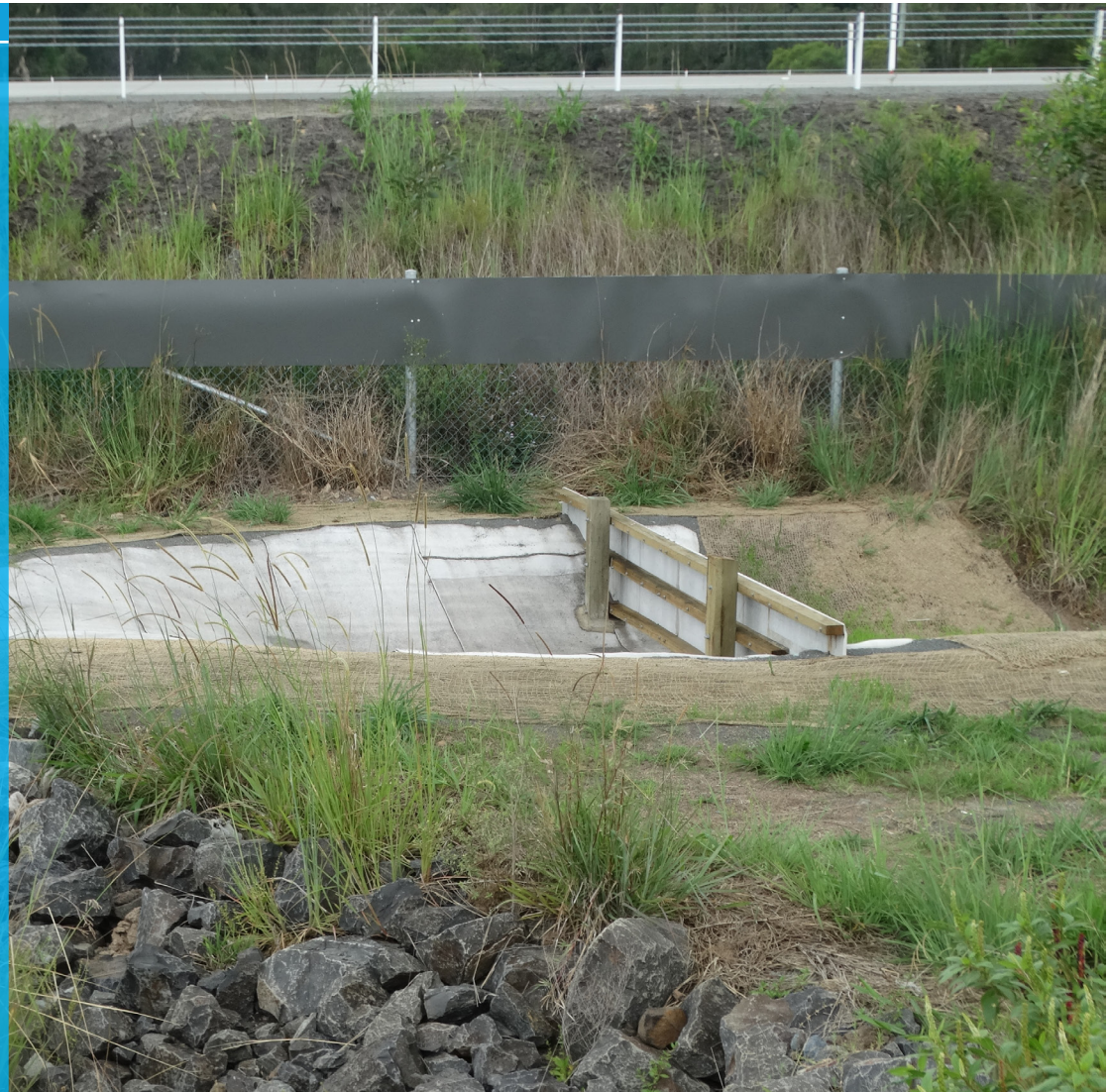
Completed channel lining installation alongside Pacific Highway
