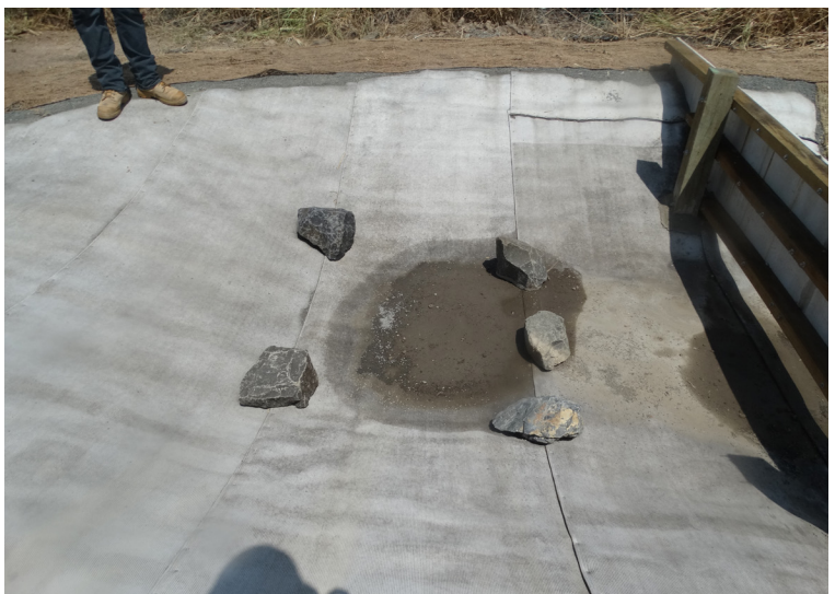
CC was laid transversely across channel
