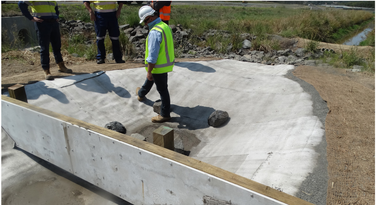
The CC will prevent erosion that would otherwise be caused by concentrated flows
