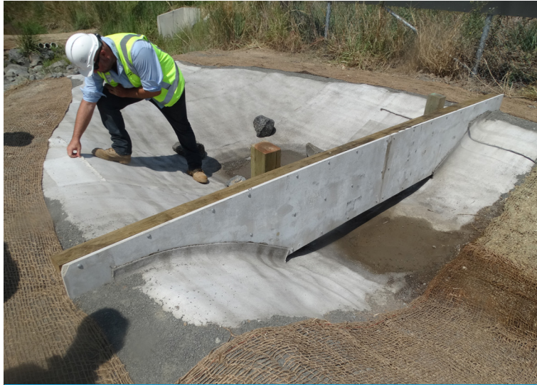
CC was installed either side of the baffle
