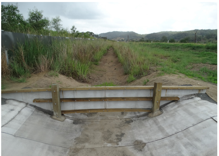
CC lined channel section feeds into an existing water course
