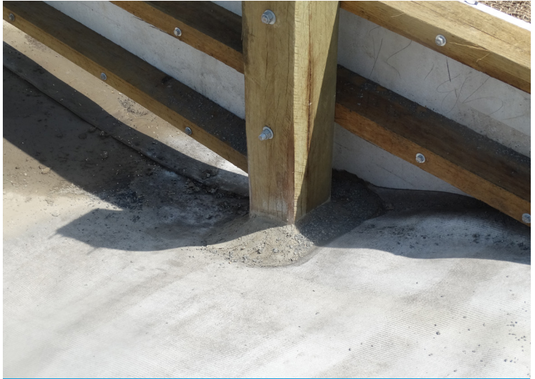
Grout was applied around baffle board posts
