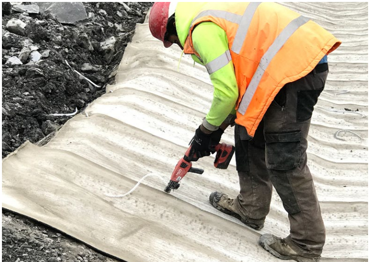
Overlapped sections were jointed using screws
