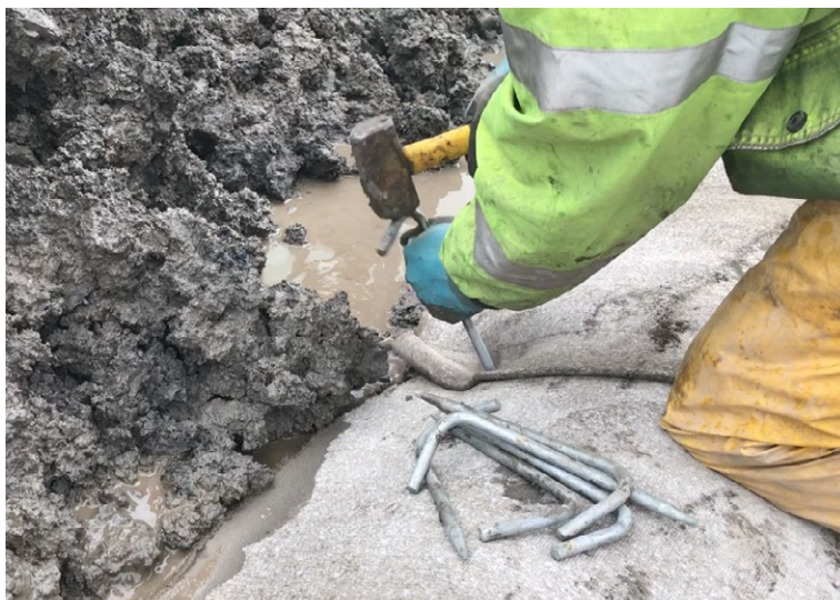
CC edges were secured with ground pegs in the anchor trenches
