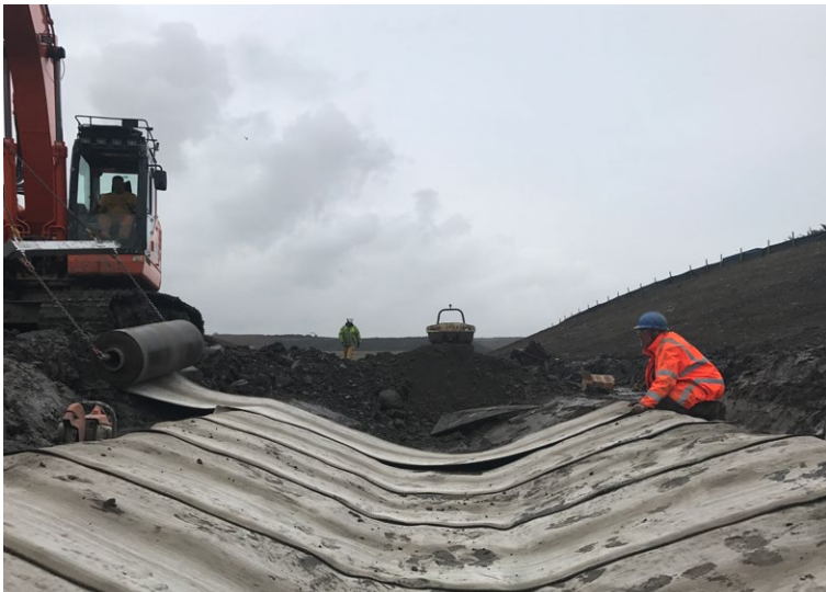
CC was laid transversely
