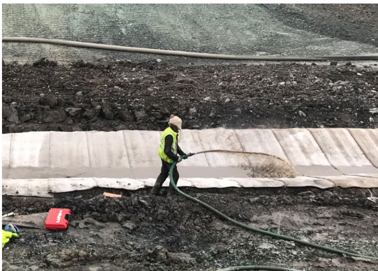
Following installation, the CC was hydrated
