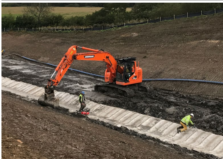
The anchor trenches were backfilled following pegging of the material
