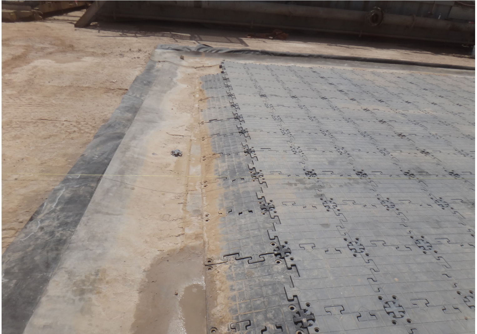
Completed channel lining installation
