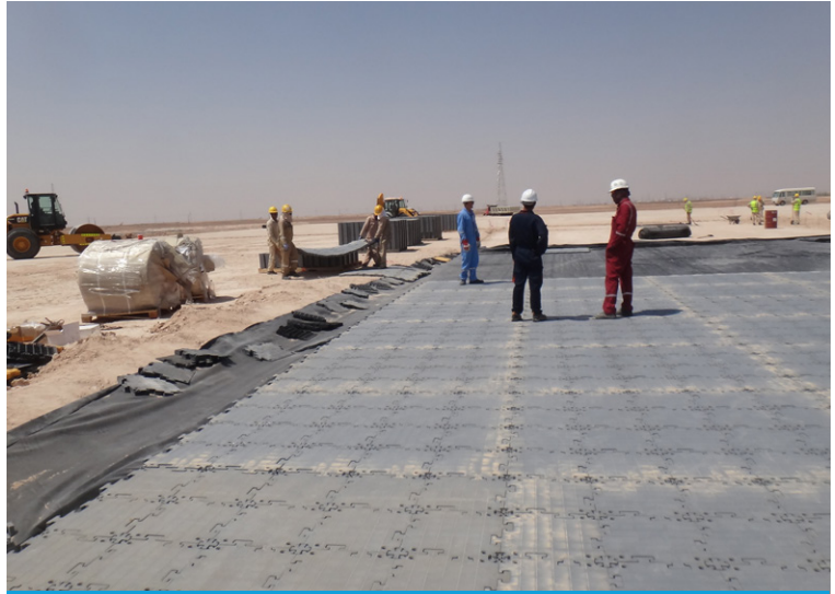
Liner laid in channels prior to deployment
