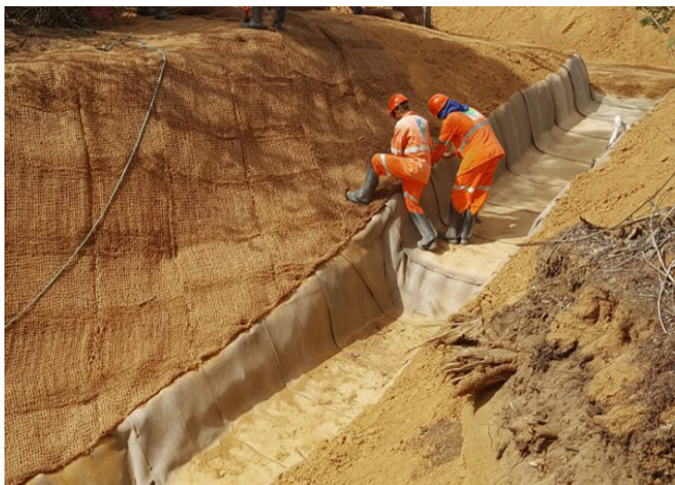
Coconut fibre was fixed to slopes around the channels after installation
