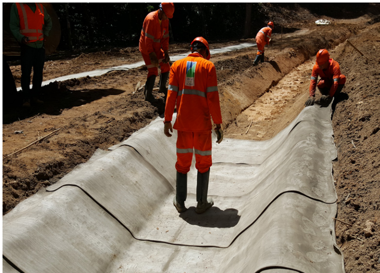
CC was laid transversely
