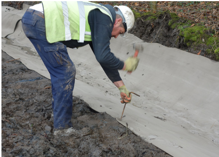
Galvanised ground pegs used to secure CC edges within anchor trenches
