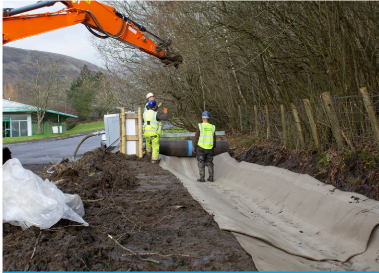
CC Wide Rolls deployed from excavator mounted spreader beam
