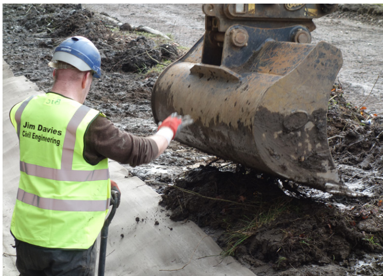
Excavator used to backfill and level anchor trenches
