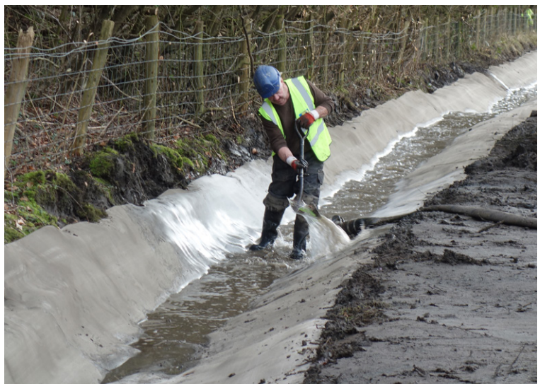
Water pumped from channel used to hydrate CC
