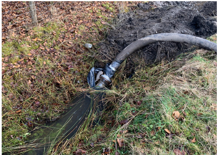
Water pumped from channel to allow ground works to be carried out
