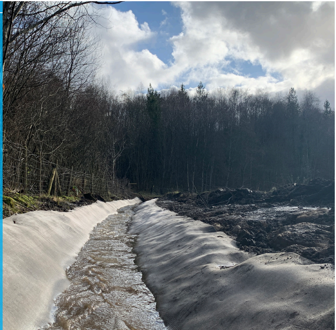
Completed channel on site of future recycling centre in Abertillery, Wales
