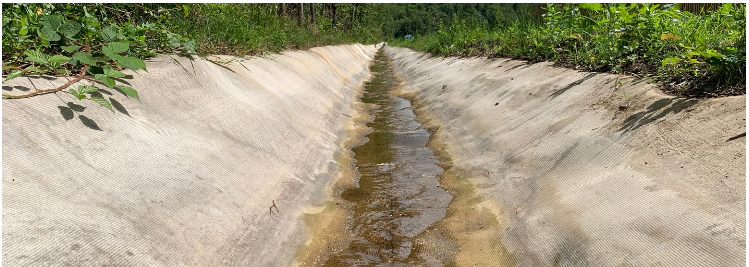
In service channel 3 months from installation
