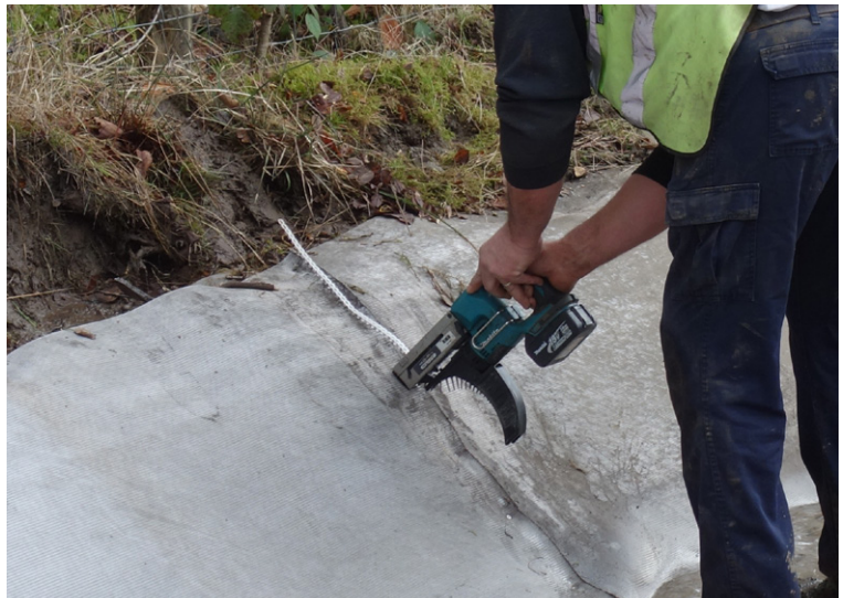
Stainless steel screws and autofed screwdriver used for jointing overlaps
