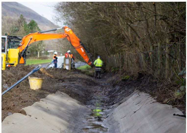
Final section of channel excavated prior to installation
