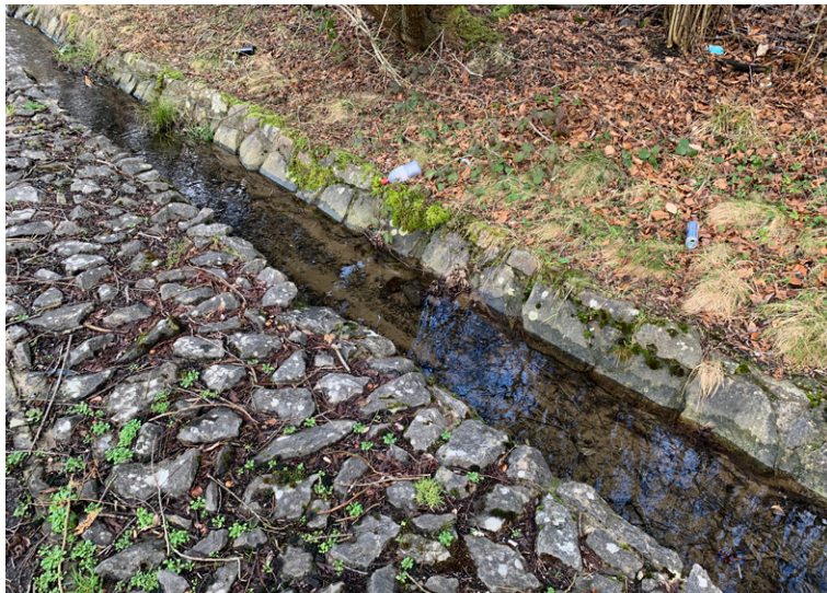
Existing concrete riprap lined channel section
