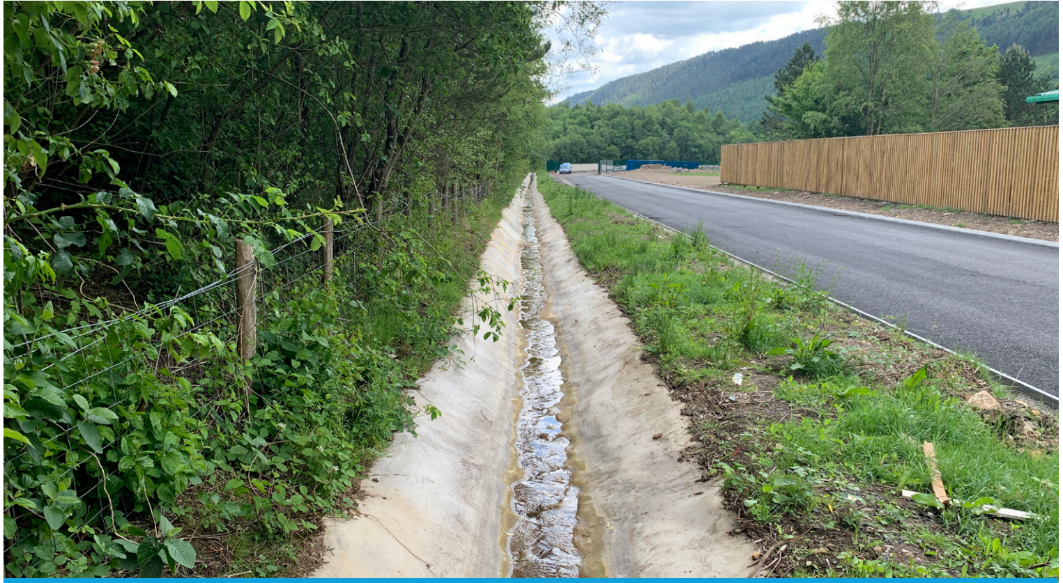
Completed channel section; hay bails used as baffling to control flow velocity following hydration
