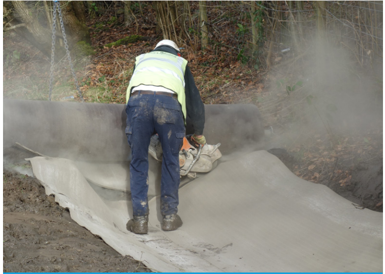
A disc cutter was used to cut the CC to required lengths
