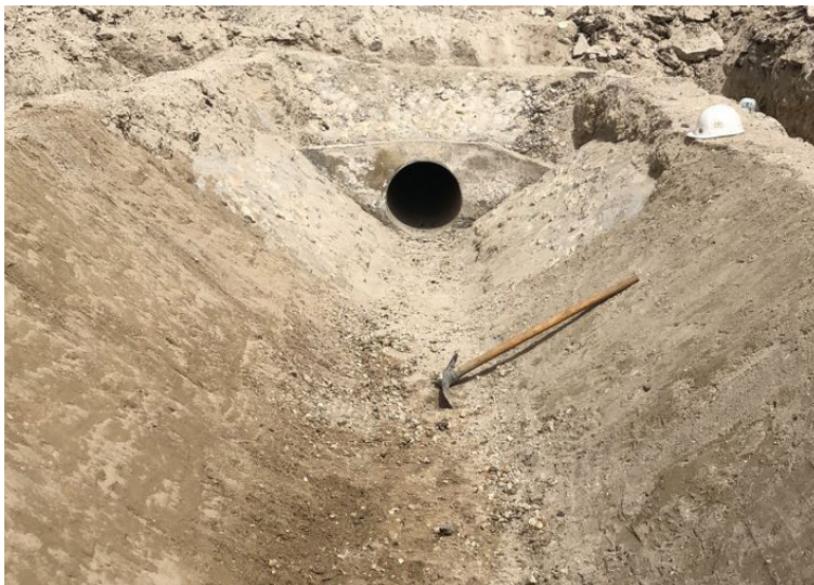
Excavated and compacted channel profile
