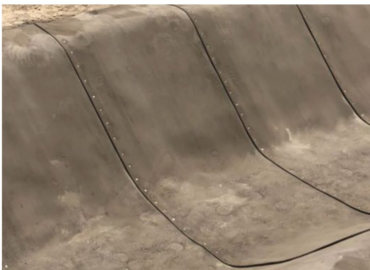
Overlaps jointed using stainless steel screws
