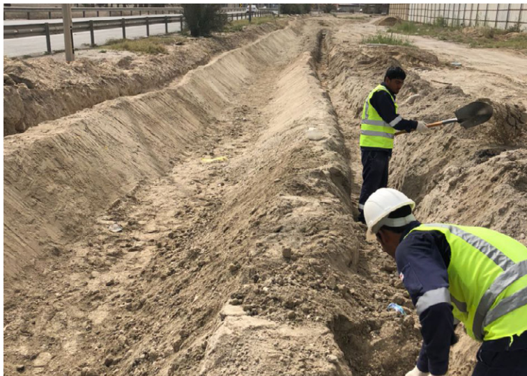
Ground preparation - anchor trenches being created on channel shoulders
