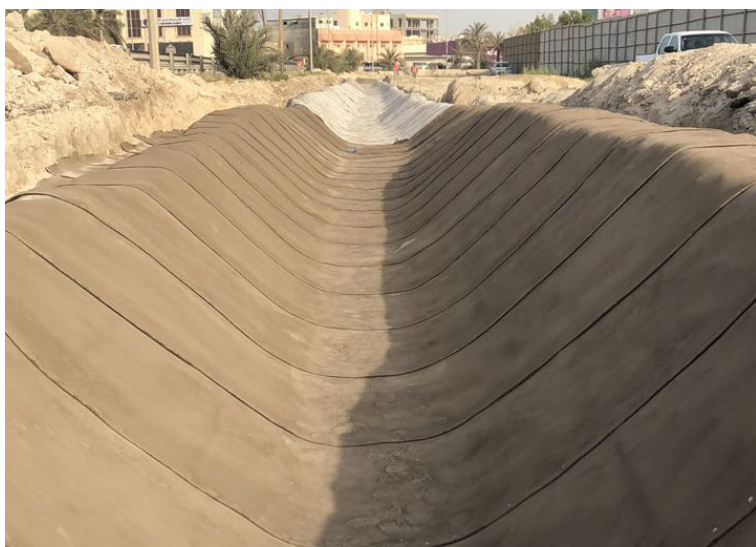
CC material laid transversely
