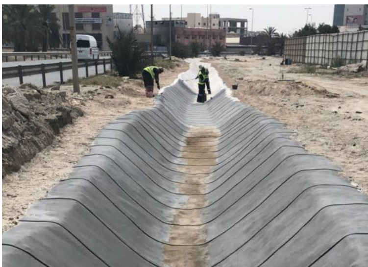
Painting of channel following material setting
