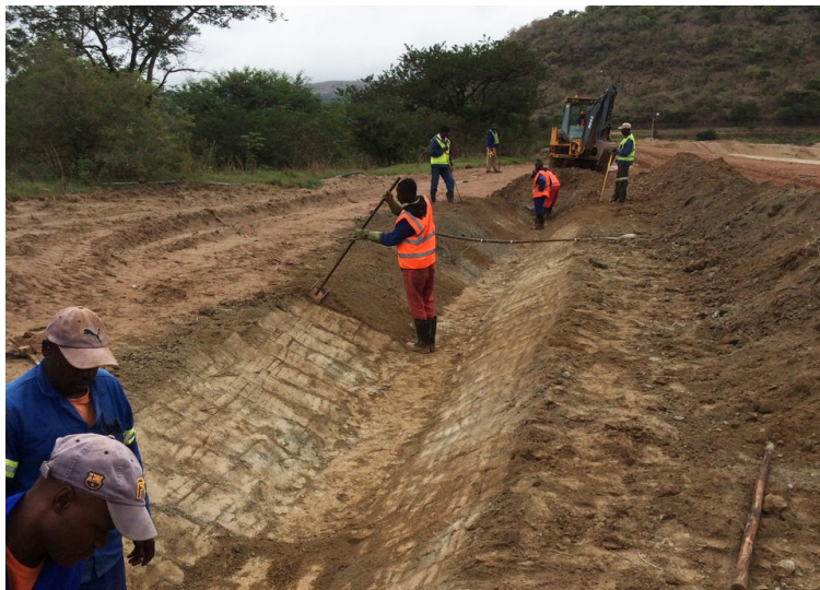
Compacting the substrate
