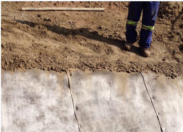
Backfilled anchor trench and jointed overlaps
