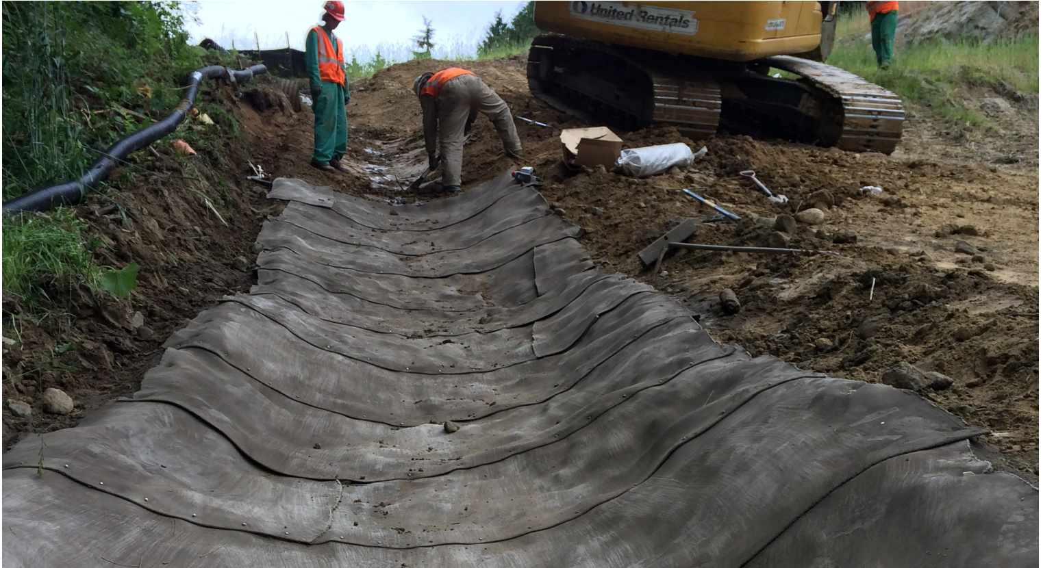
Ground preparation was carried out by digger and with hand tools
