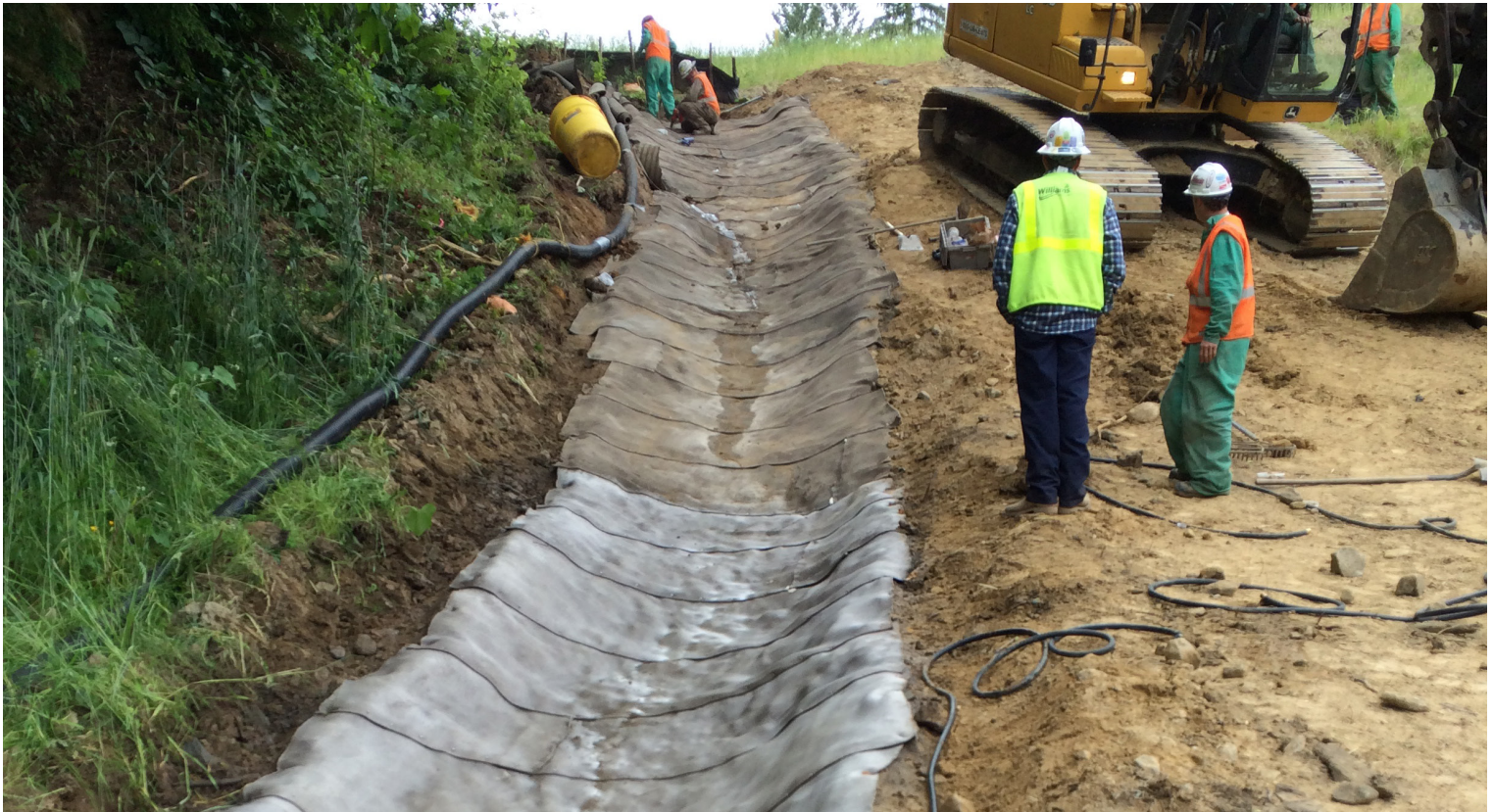
Completed section of hydrated channel
