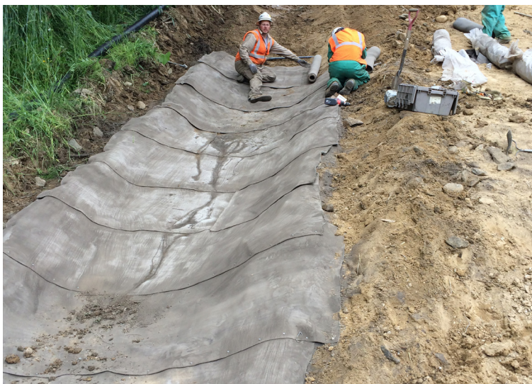
CC was laid transversely
