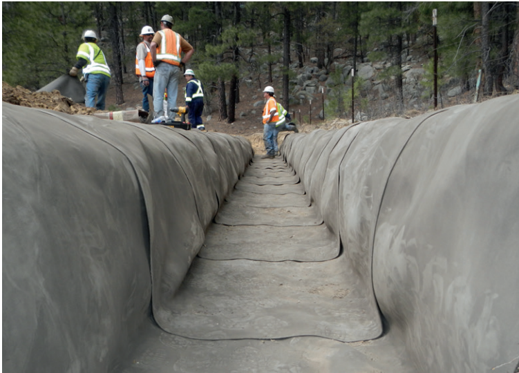
Completion of French drain
