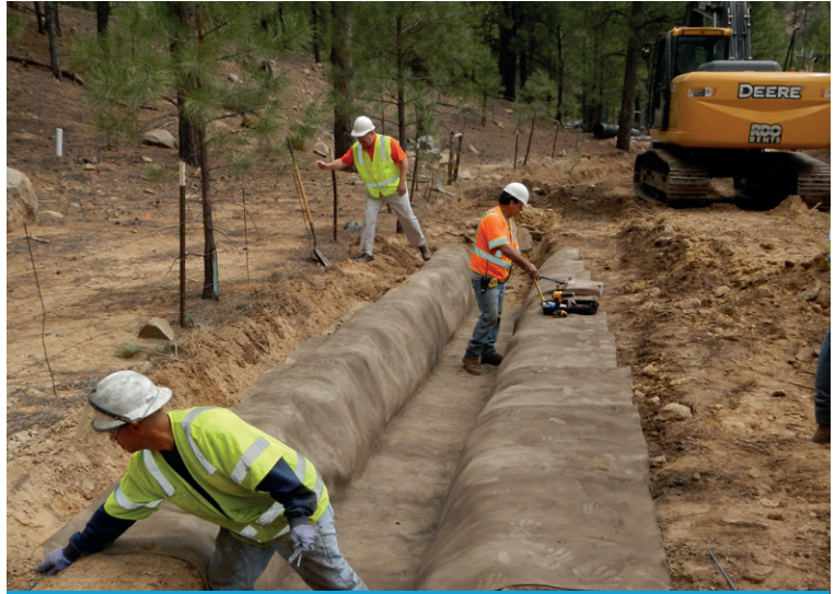
CC was laid transversely in both channel sections
