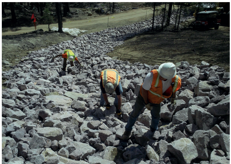
Placement of drain rock over and around perforated pipe
