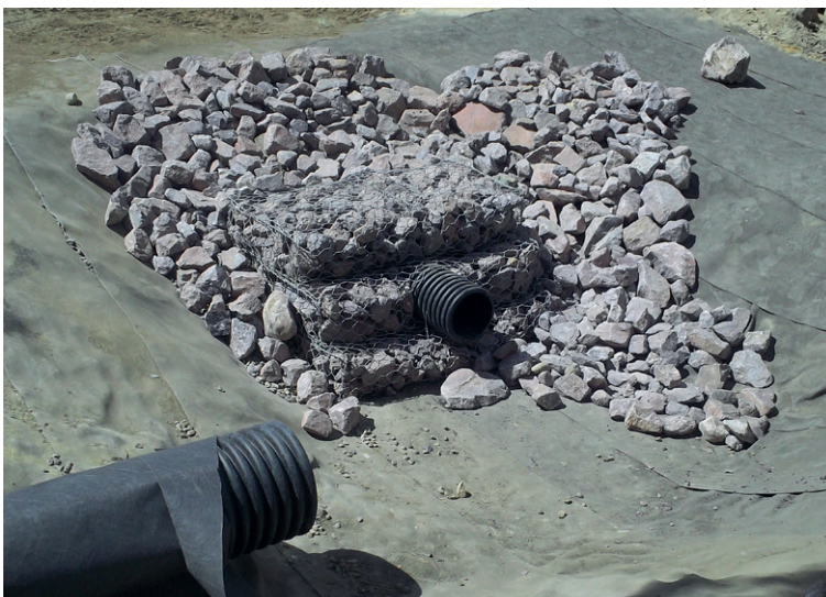
Pipe outflow covered with gabions and drain rock
