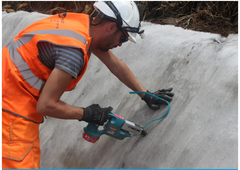
Screws were used to joint overlaps of CC
