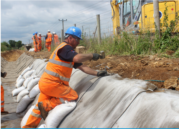
Ground pegs were used to fix the CC
