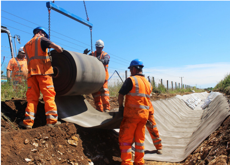
Over 2,000m² of CC was used for the installation
