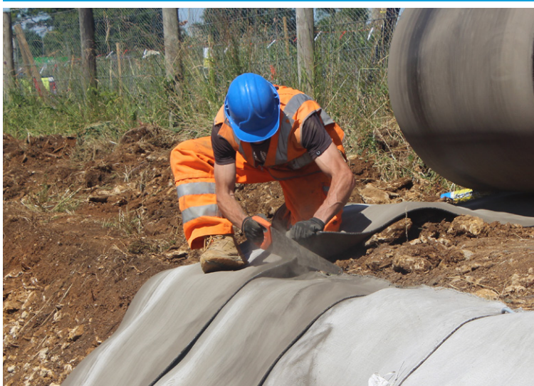
The CC was laid transversely and cut, once laid, using a hand saw
