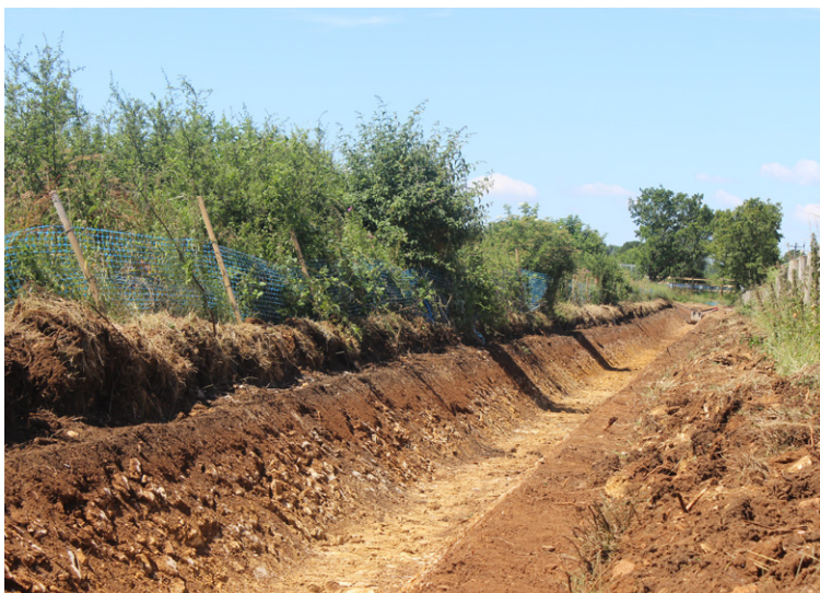
The channel was graded prior to installation
