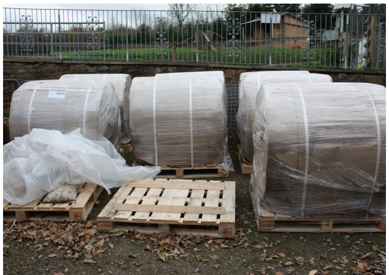
Bulk rolls of CC were delivered to site
