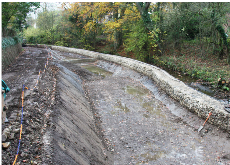
The substrate was then re-graded to provide a smooth surface for installation
