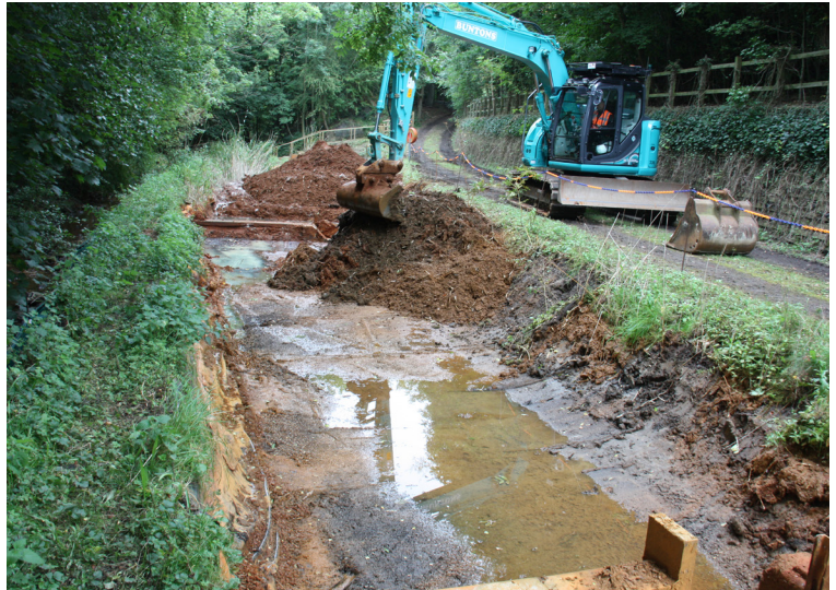
The channel was excavated to remove all ochre traces
