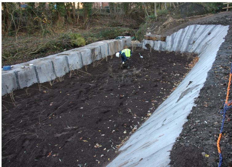
Following hydration, soil was laid and reeds planted
