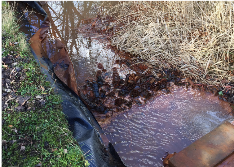
The original HDPE lining had disintegrated and come away
