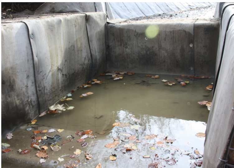
Flexibility of CC allowed for easy covering of complex sections
