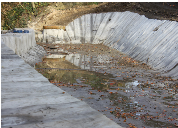
The material was laid transversely across the full width of the channel
