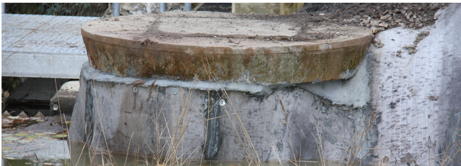
Termination detail around existing infrastructure
