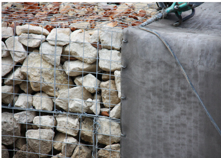
CC was attached to the gabion baskets using hog rings
