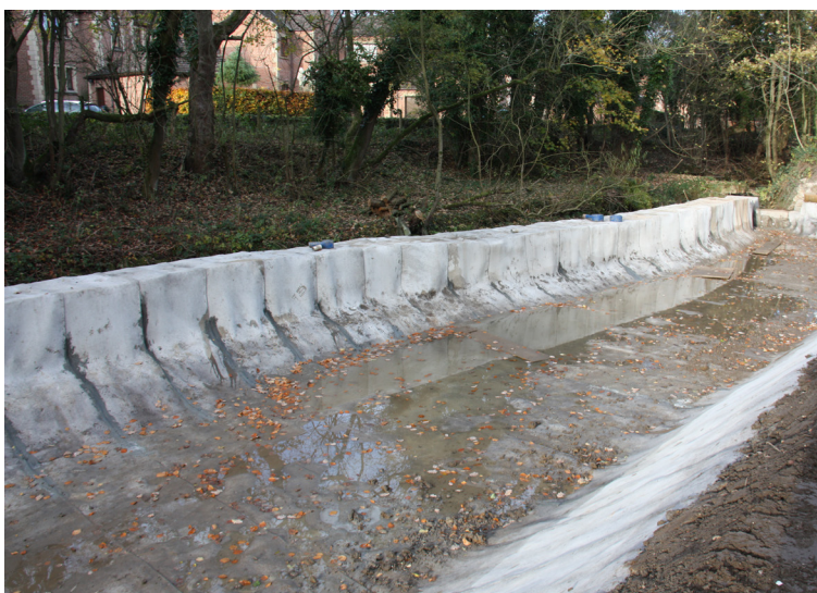
The joints were then sealed to further prevent ingress
