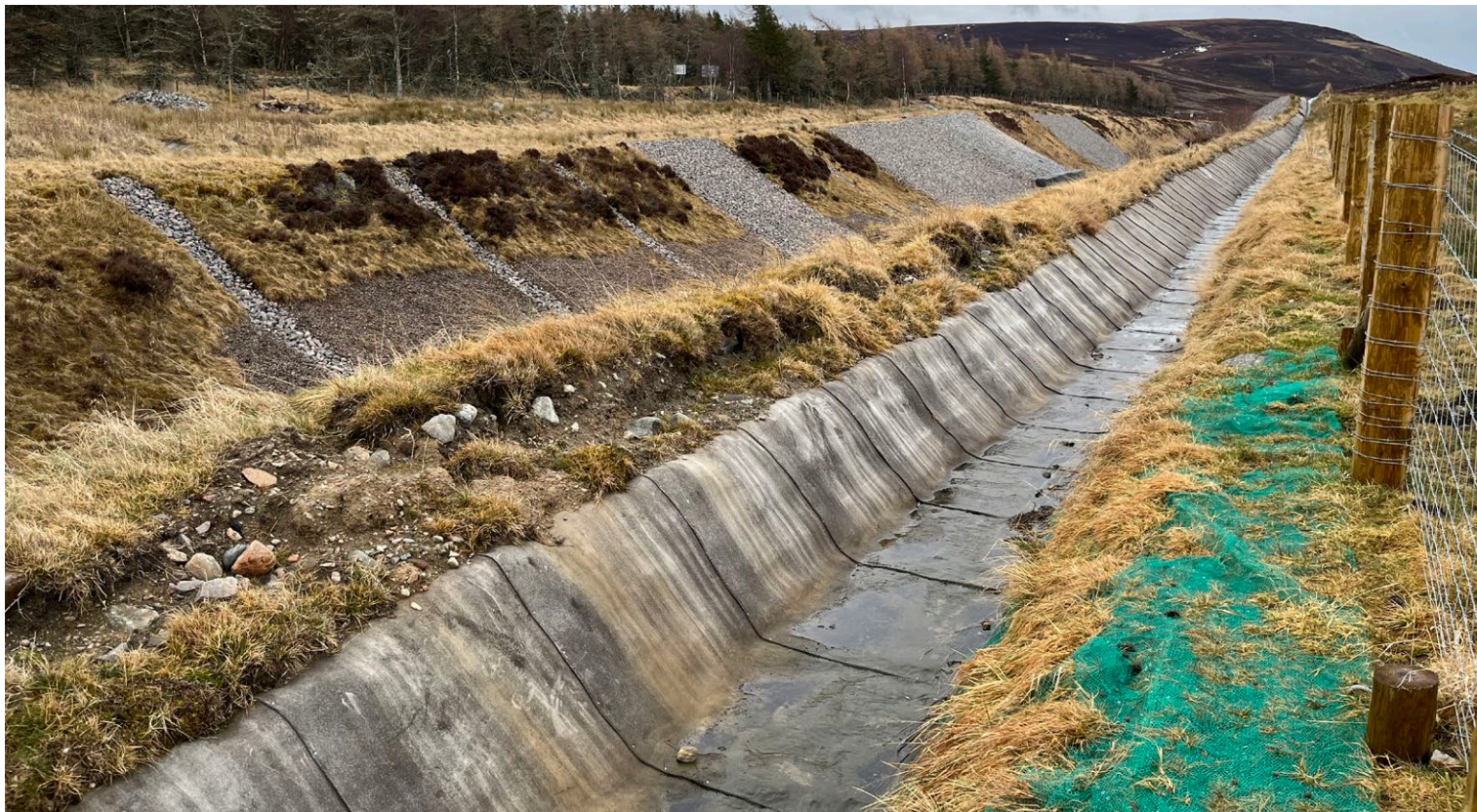
Completed channel lining works
