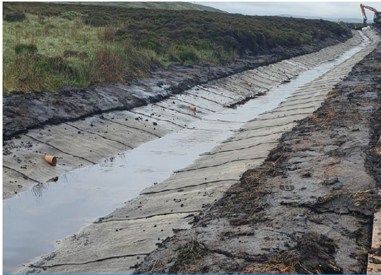
CC8™ (Type II GCCM) cut to length on site & laid transversely across channel
