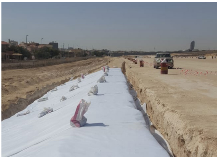
A geotextile was laid prior to installing CC
