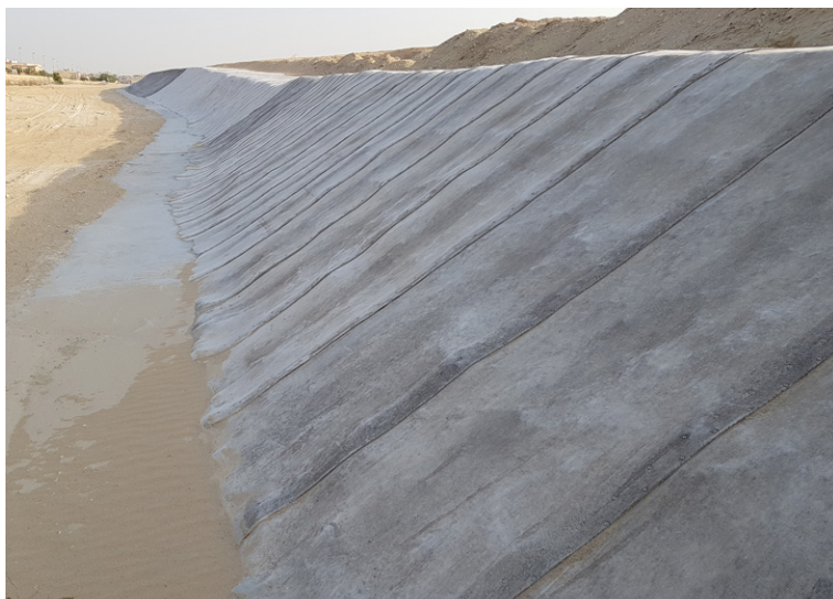
Completed slope protection installation following backfilling of anchor trenches
