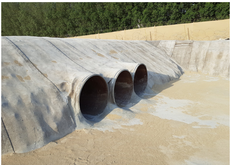
Completed installation around outflow pipes
