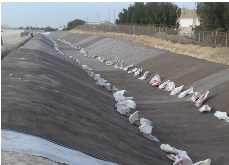
Channel lining installation in progress
