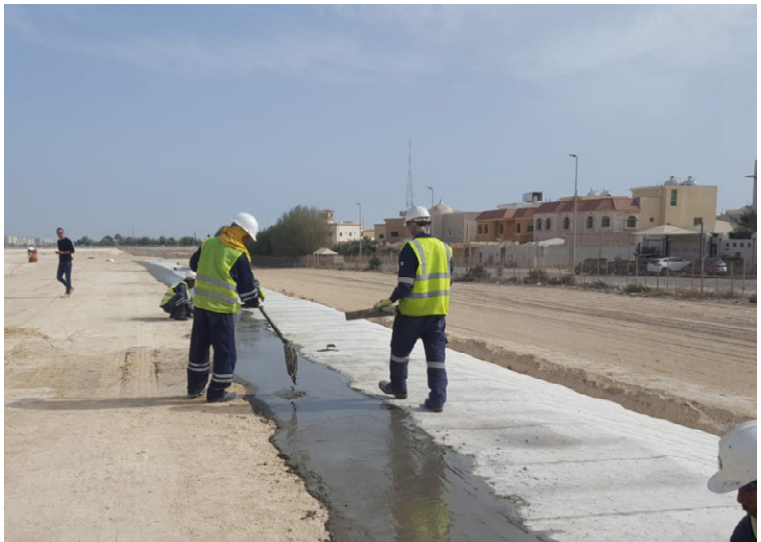
Filling anchor trenches with poured concrete
