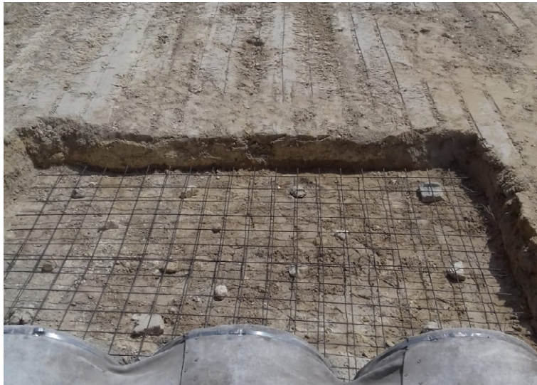
Formwork put in place for capturing CC in anchor trenches
