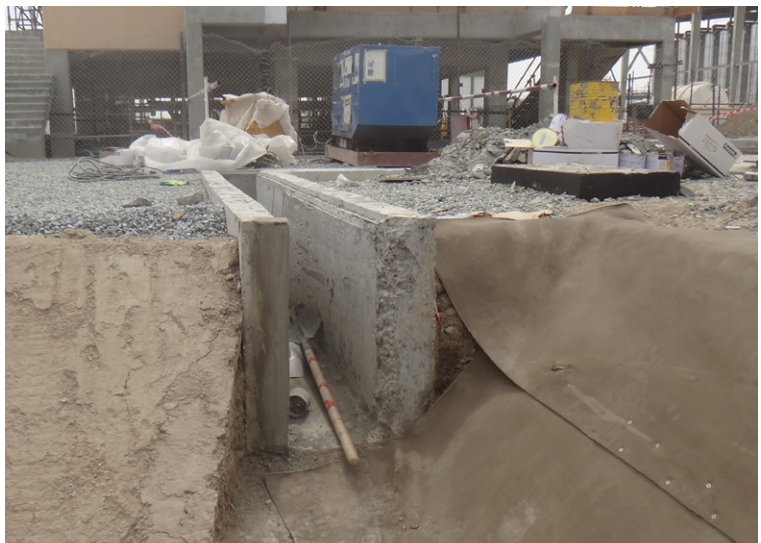
Installation of CC around drain inlet
