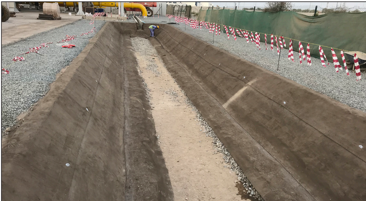
Completed installation prior to hydration
