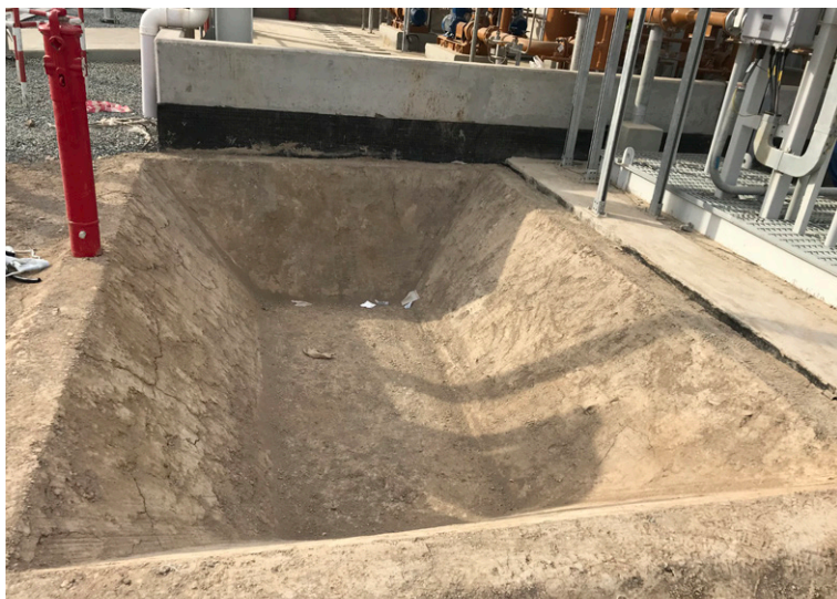
Smaller French drain prior to works
