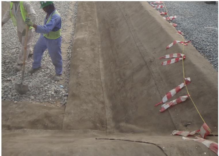
Completed installation of three CC layers
