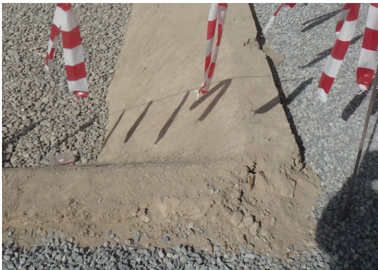
Soil-based substrate showing signs of erosion
