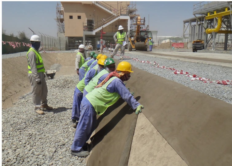
Installation of first CC layers
