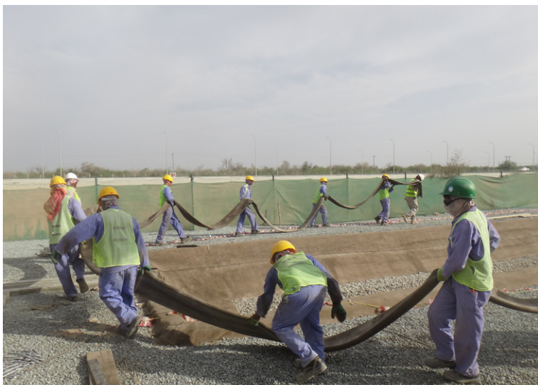
CC lengths manually transported
