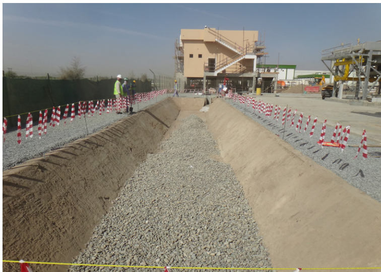
French drain prior to works
