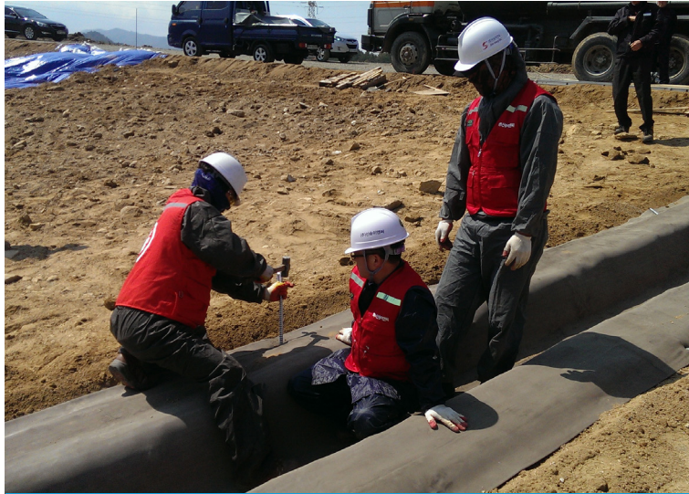
Fixing to substrate with ground pegs
