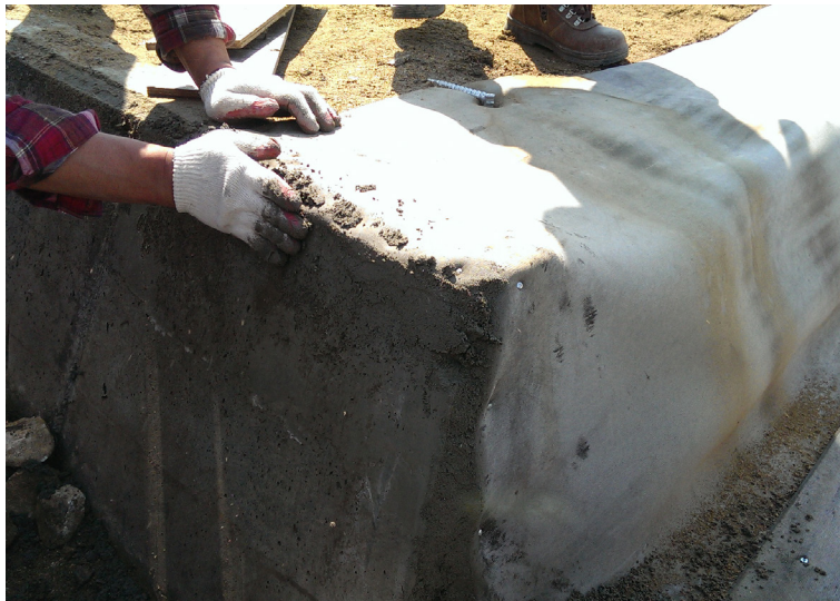
Concrete grout used to join CC to existing poured concrete channel
