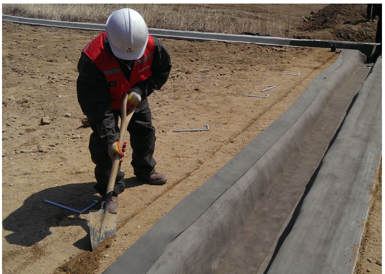
Cutting anchor trench into shoulder
