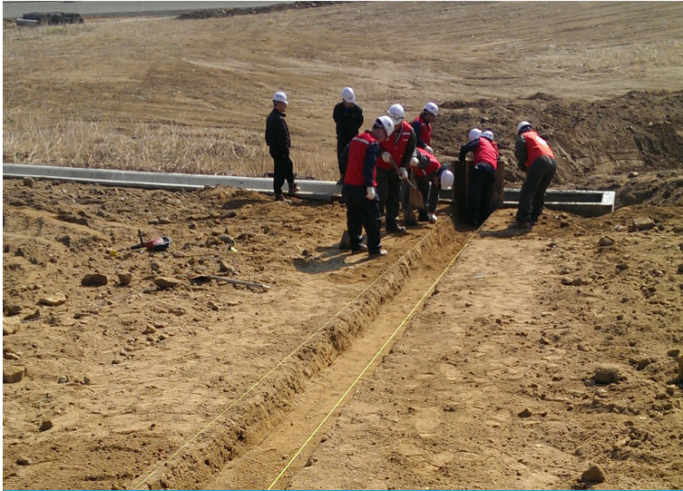
Excavation to profile
