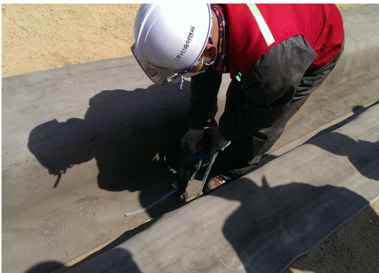
Screwing joints at 200mm intervals
