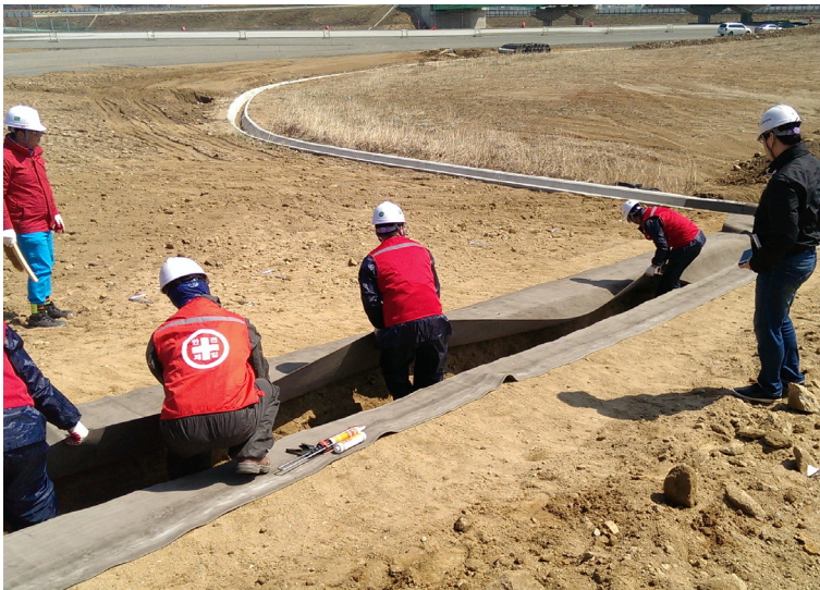
Positioning CC in channel with 100mm overlap
