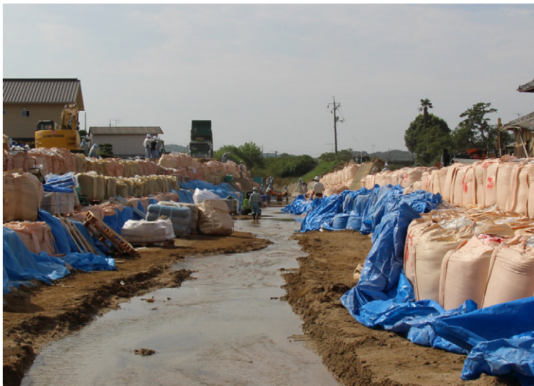
Sand bags in place prior to CC installation
