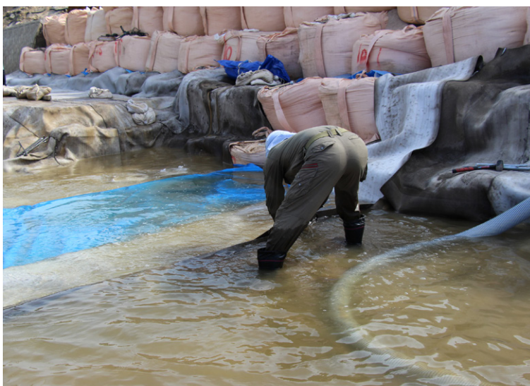
Placing CC below water
