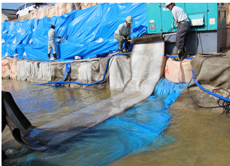
Deployment of CC batched rolls
