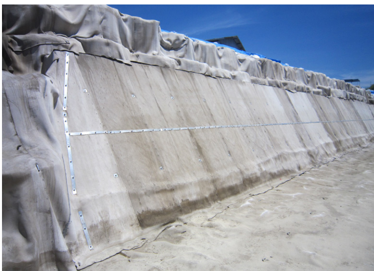
CC fixed to remaining concrete blocks using masonry nails & termination bars
