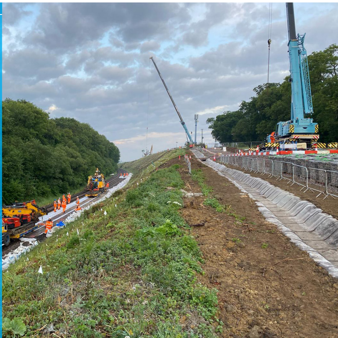
Completed channel lining installation on site in Templecombe; works ongoing on the rail line
