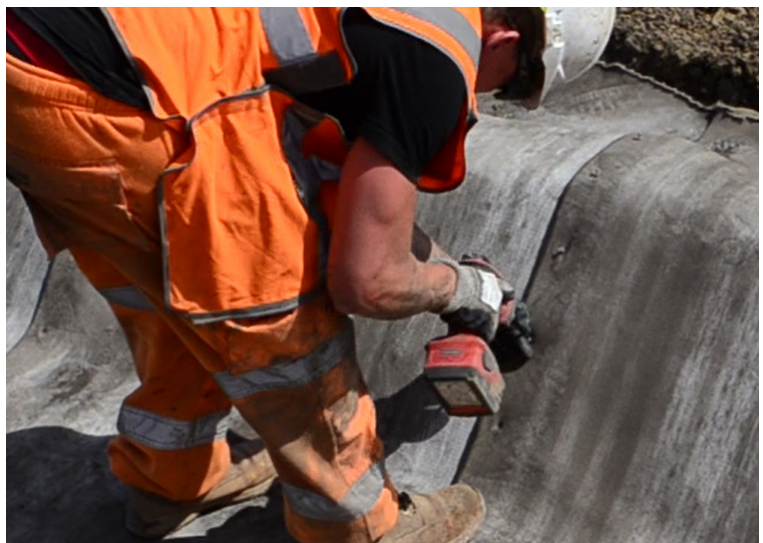
Jointing overlaps with stainless steel screws
