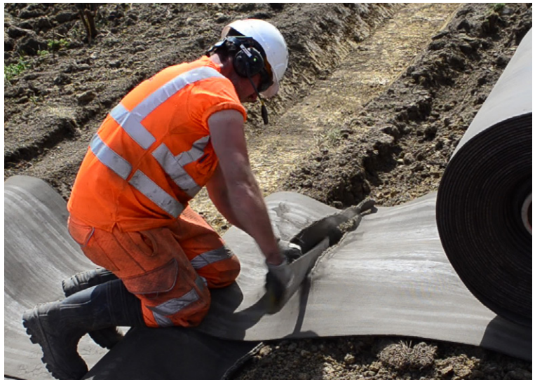
CC cut to required length in-situ using hand saw
