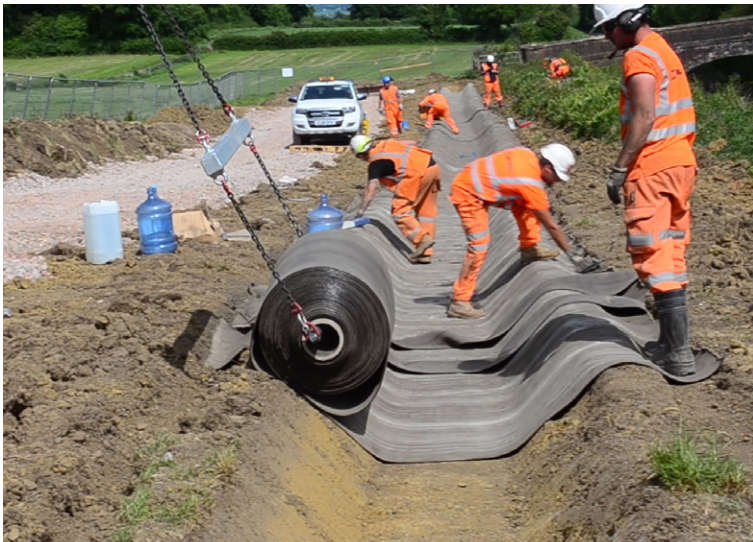
Deployment of the CC bulk rolls
