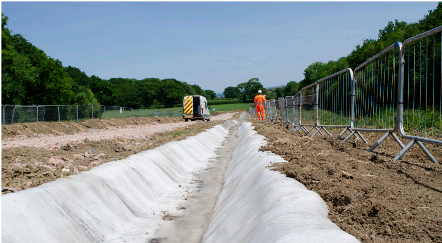
Completed Concrete Canvas® crest drainage channel lining installation
