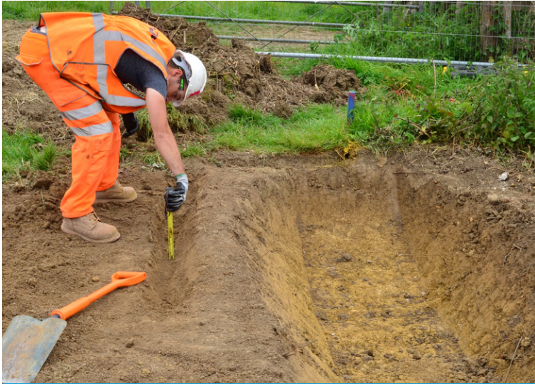
Measuring and creating anchor trenches
