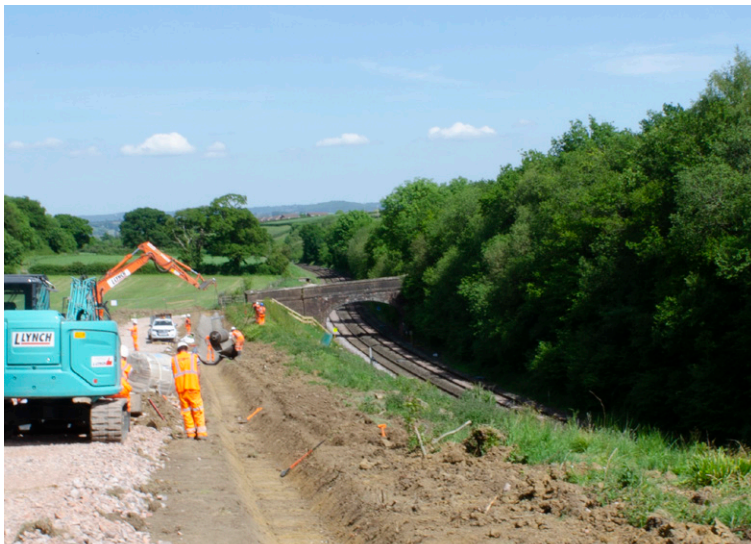
Proximity of crest drainage channel to rail line
