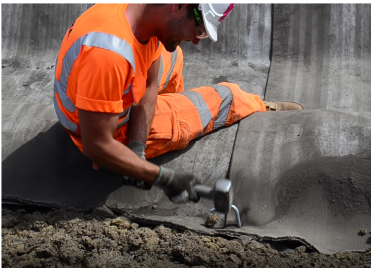
Securing CC within anchor trenches using ground pegs
