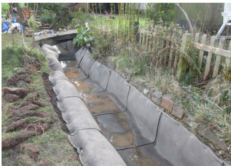
CC installed prior to backfilling anchor trenches
