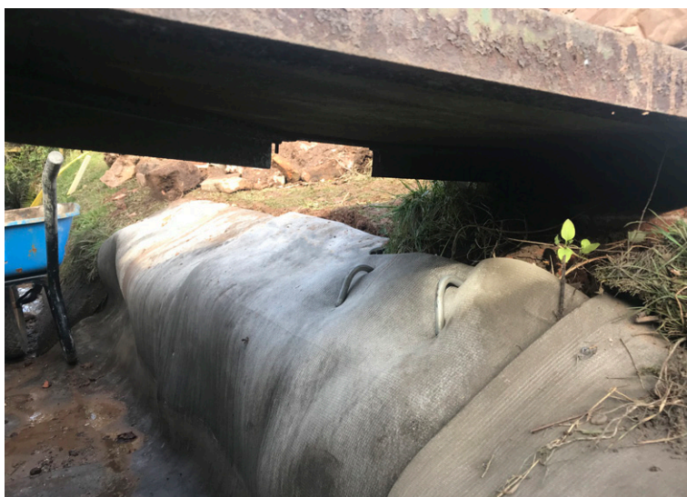
CC pinned under bridge structure
