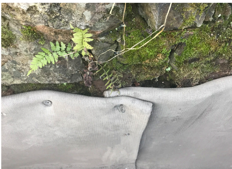
CC secured to masonry with anchors
