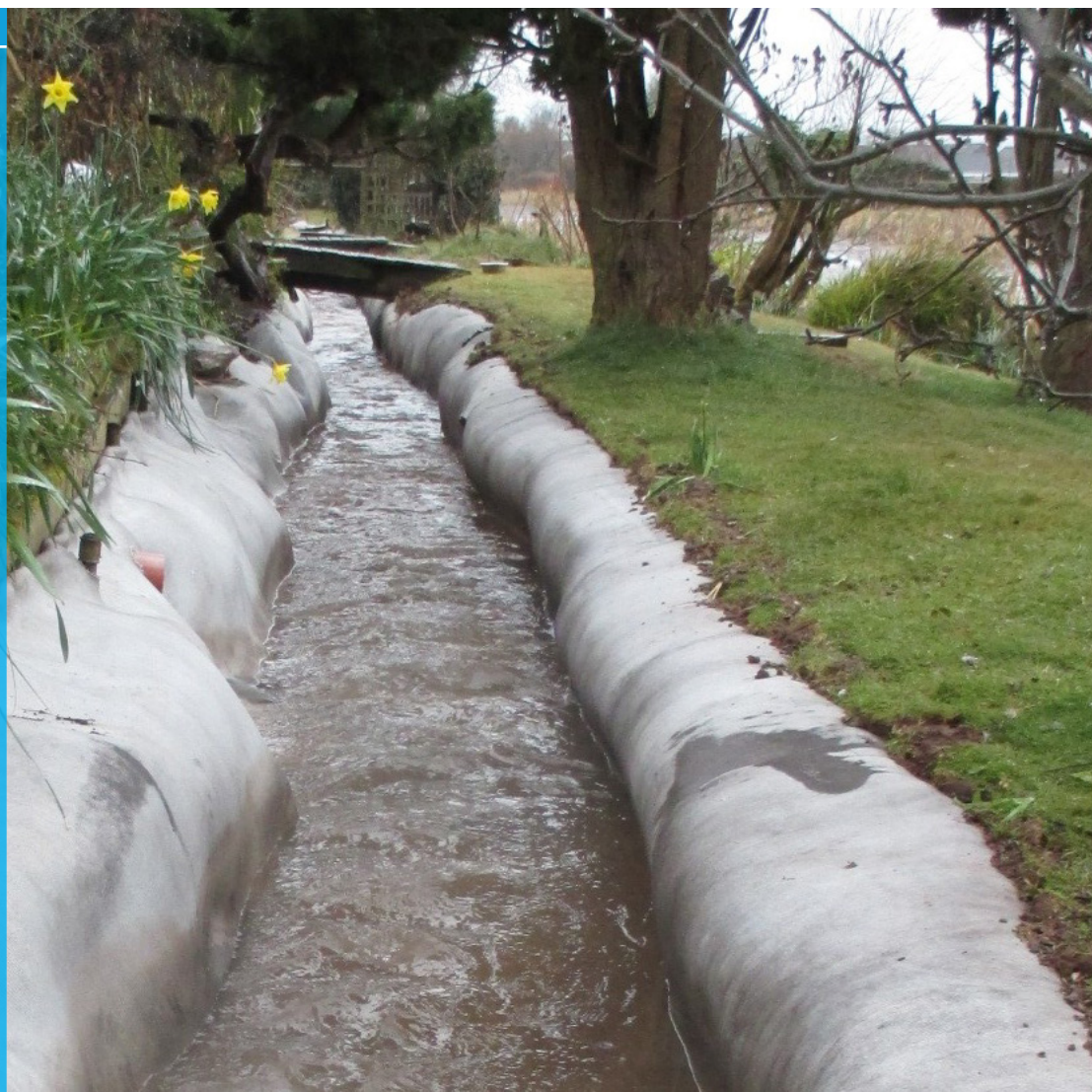
Completed CC lined channel
