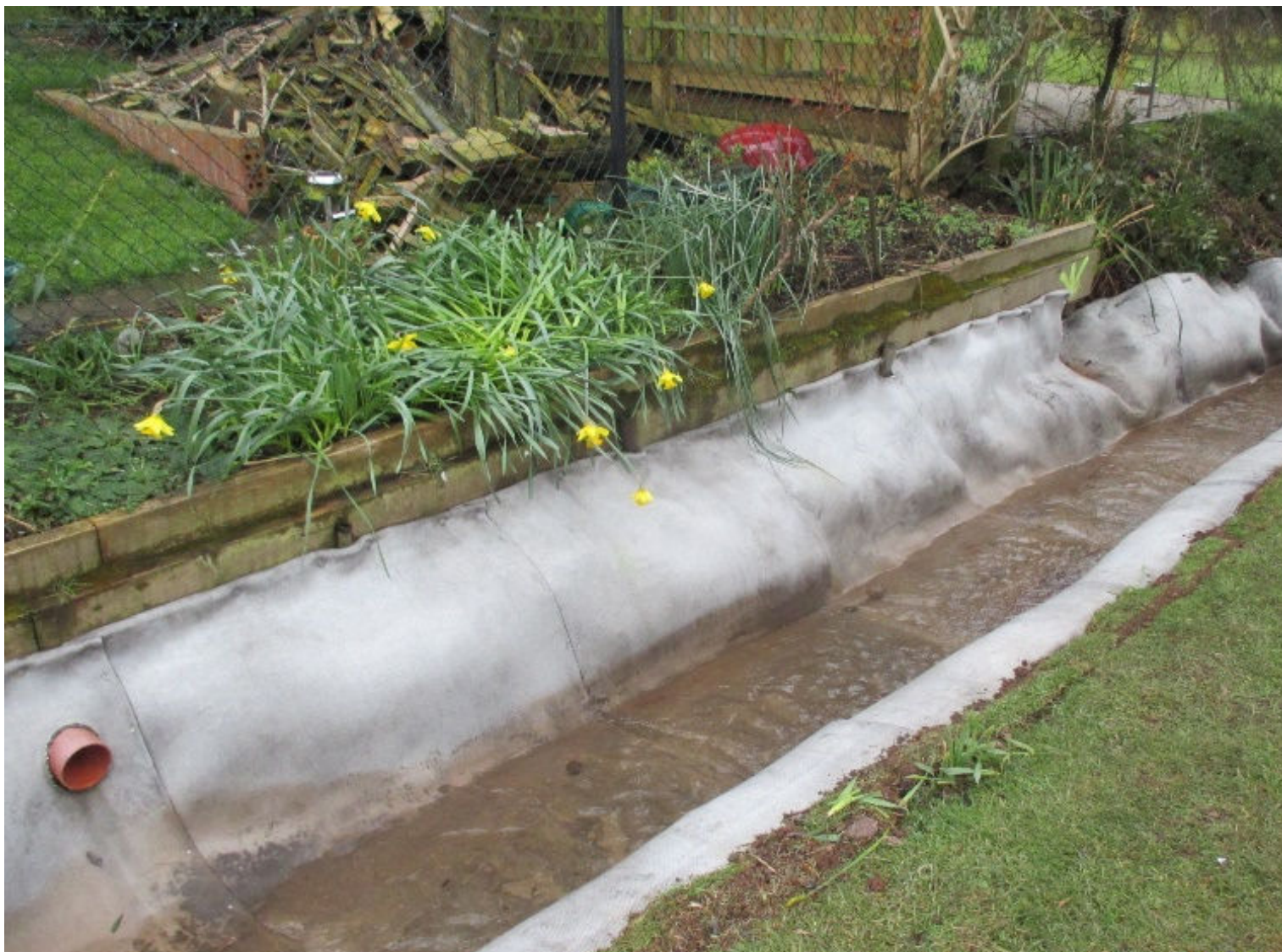
Completed channel with variety of anchor fixings and pipe penetrations
