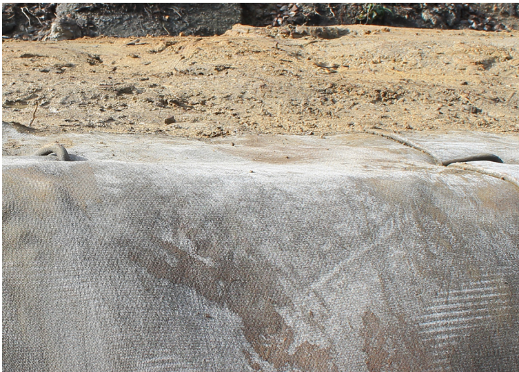
Ground pegs used to fix material in anchor trenches
