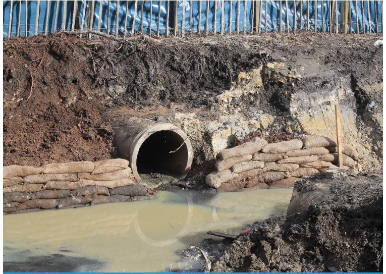
Sandbag retaining wall
