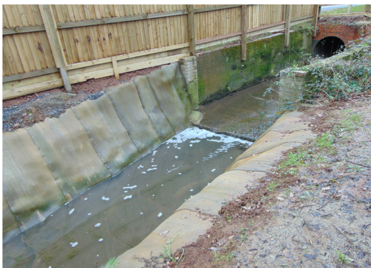
Interface with existing brickwork
