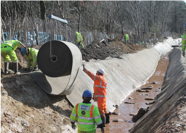
CC deployed from spreader beam and plant
