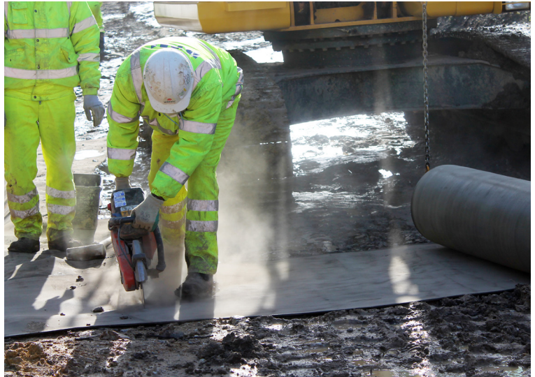
CC cut to length using disc cutter
