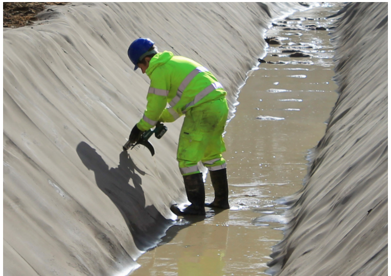
CC jointed with screws
