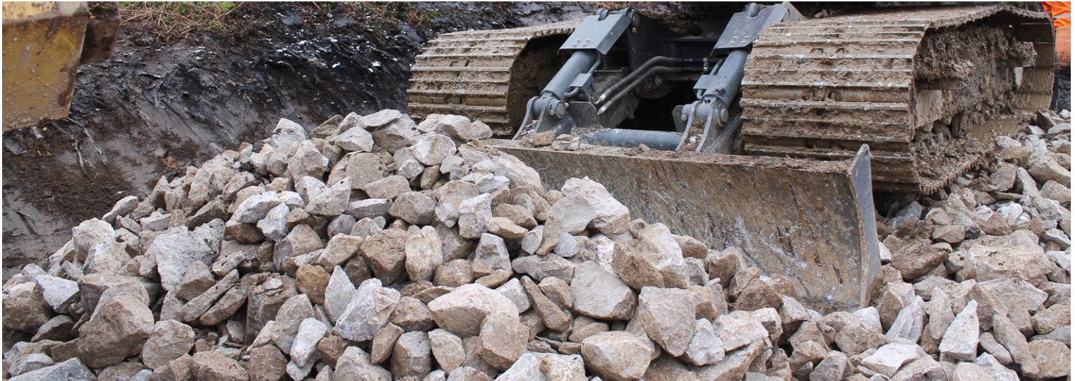
Applying top surface aggregate layer
