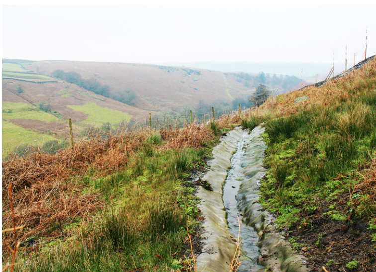
Adjacent CC lined open channel minor works originally installed in 2014
