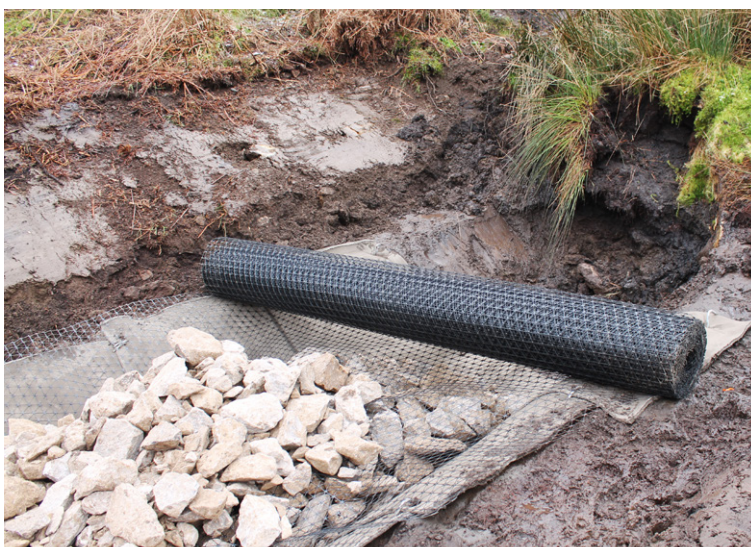
Second aggregate layer applied on top of geogrid
