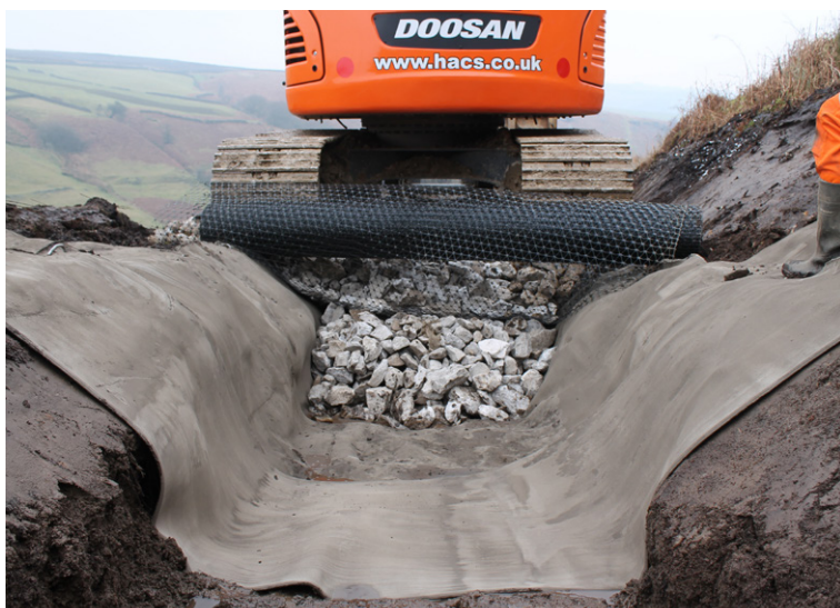
Transverse layers of CC13 deployed in conjunction with aggregate and grid
