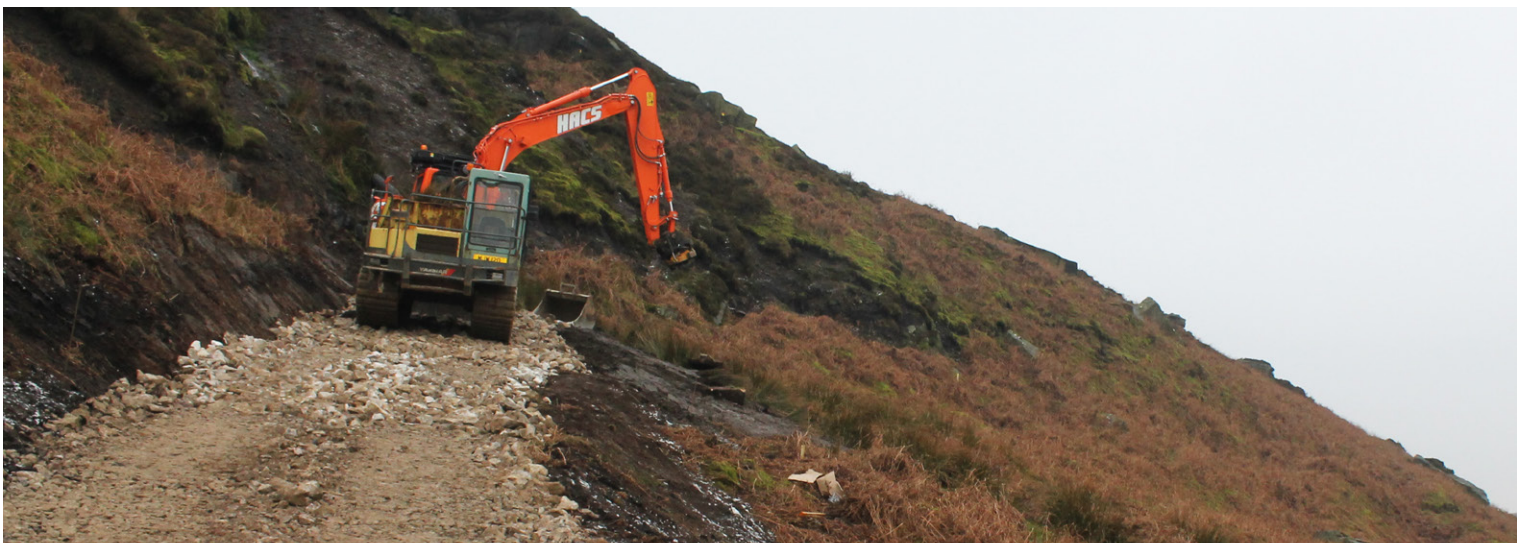
Applying top surface layers and compacting access road
