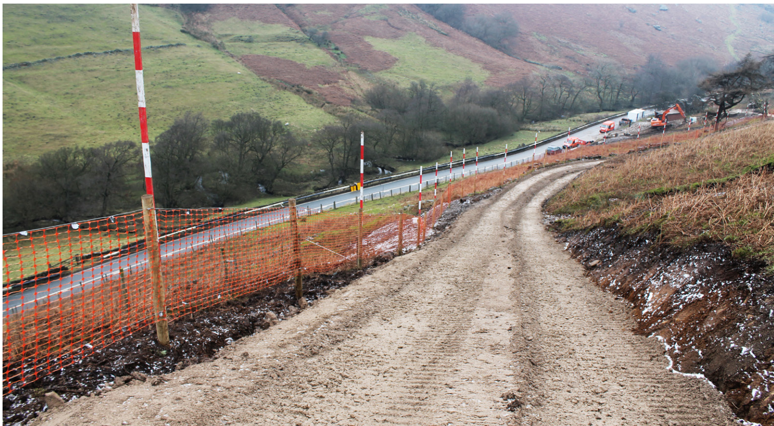
Completed aggregate drainage channel overtopped with temporary access road
