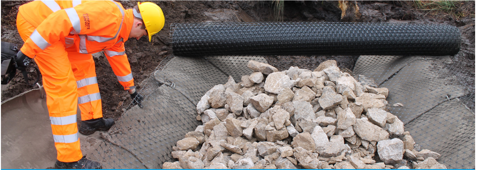
Inspecting second layer aggregate layer and geogrid
