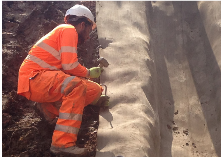
Pegging into anchor trench
