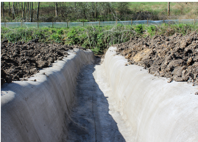
Backfilled anchor trench
