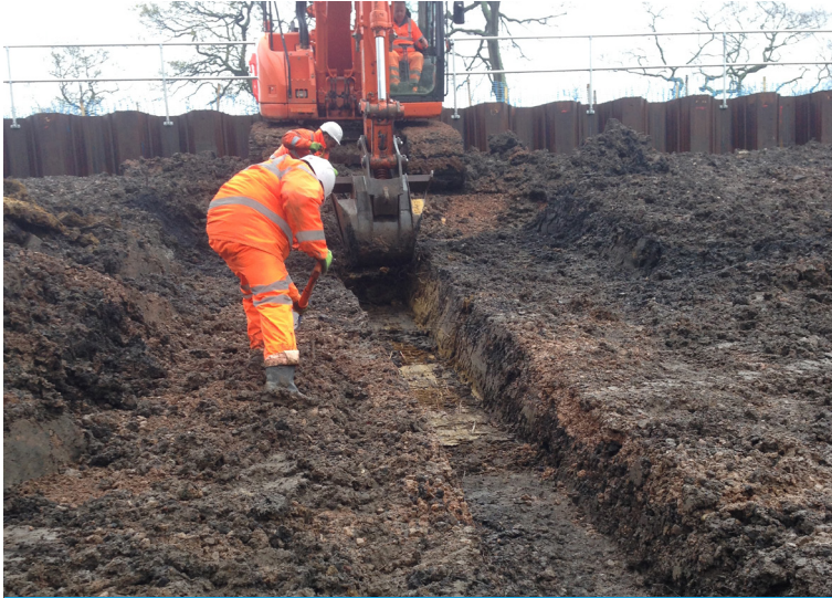
Excavating channel and creating anchor trenches
