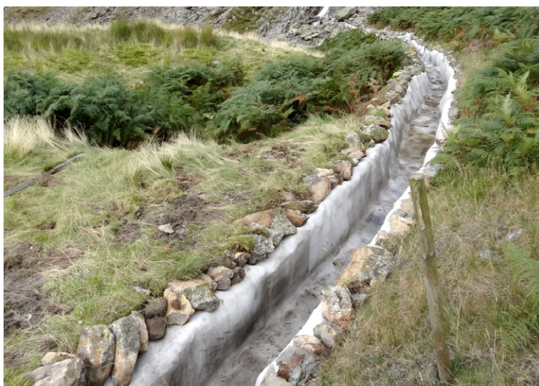
The completed lined channel at Glenridding, Ullswater
