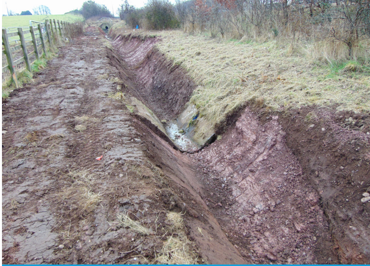
Channel excavated to profile
