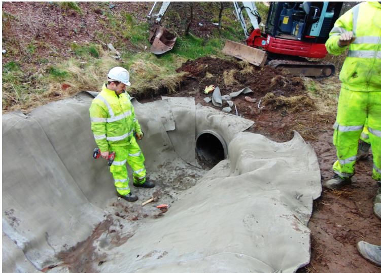
Termination at sandbag headwall
