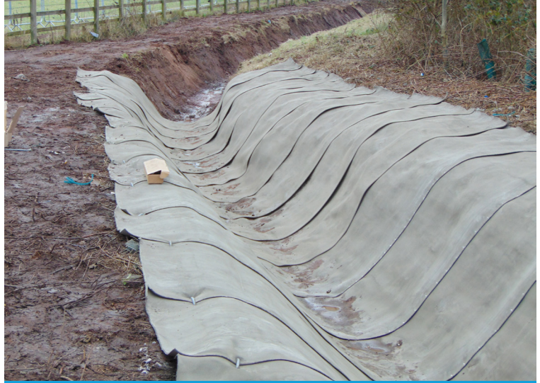
Batched rolls of CC8™ were laid transversely across channel
