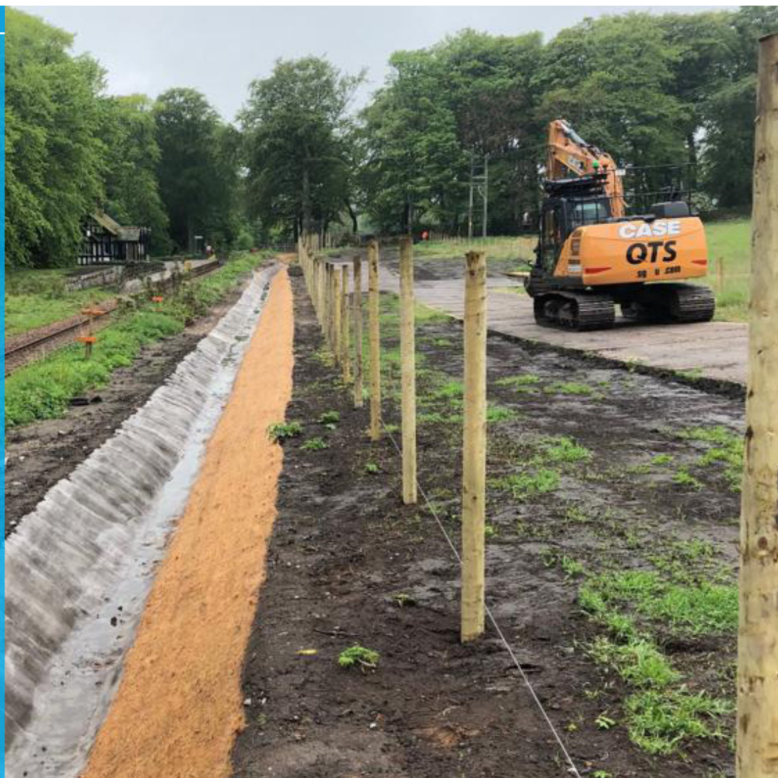
Completed channel lining installation in Sutherland
