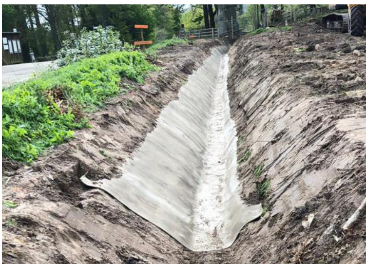
CC terminated into anchor trenches
