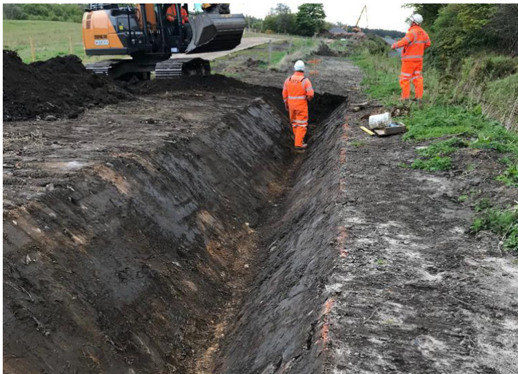
Excavation of the channel profile
