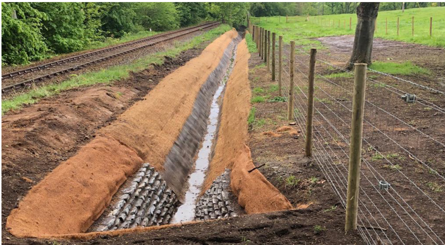
Completed CC lined channel
