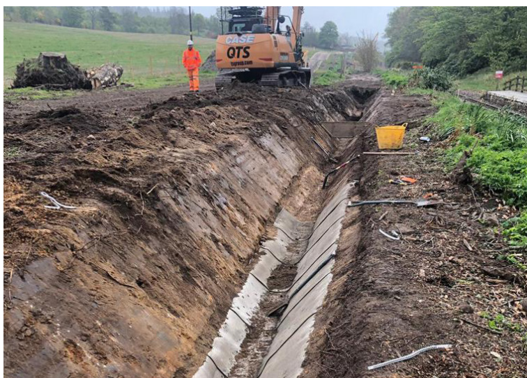
CC laid transversely across the channel
