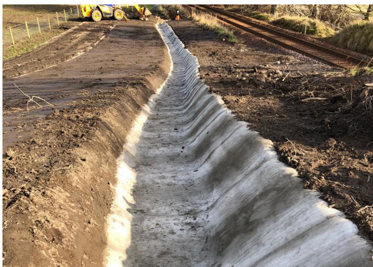
Anchor trenches backfilled prior to erosion mat installation
