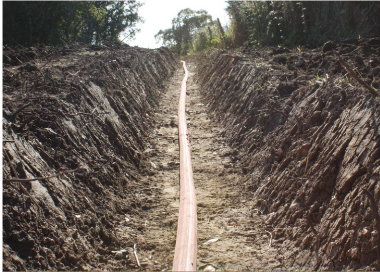
Trapezoidal ditch profile cut prior to install
