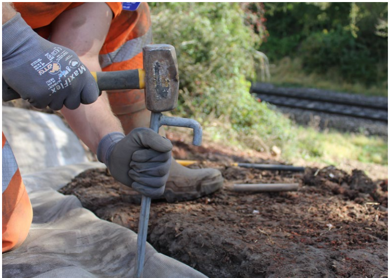
CC8™ Pegged in anchor trench
