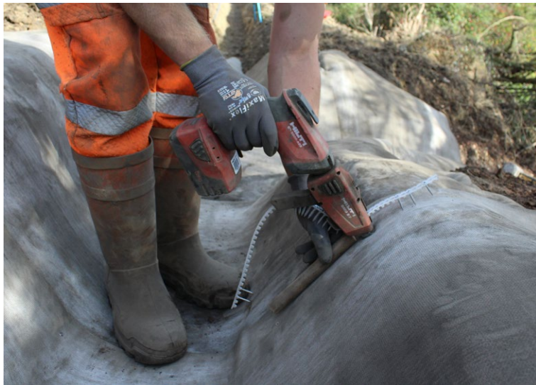
CC8™ Laid transversely & secured with 30mm stainless steel screws
