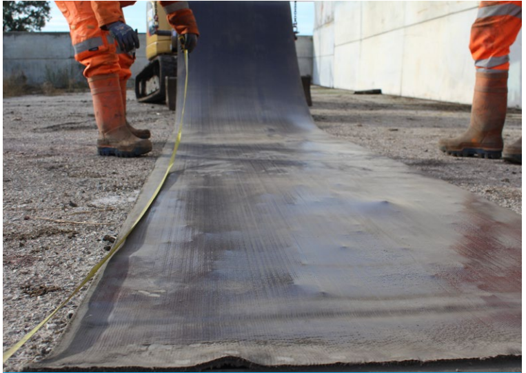
CC8™ measured & cut into 3.5m lengths
