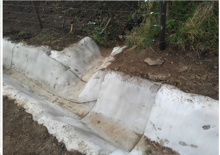
Junction detail to collect water from natural drainage paths
