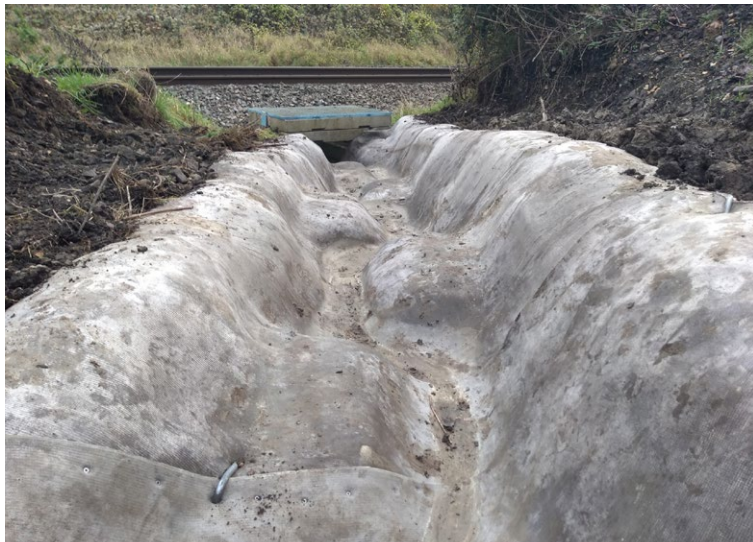
Baffled cascade formed with concrete sandbags lined in CC™
