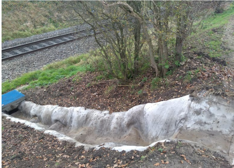
Cascade connection to the track drainage
