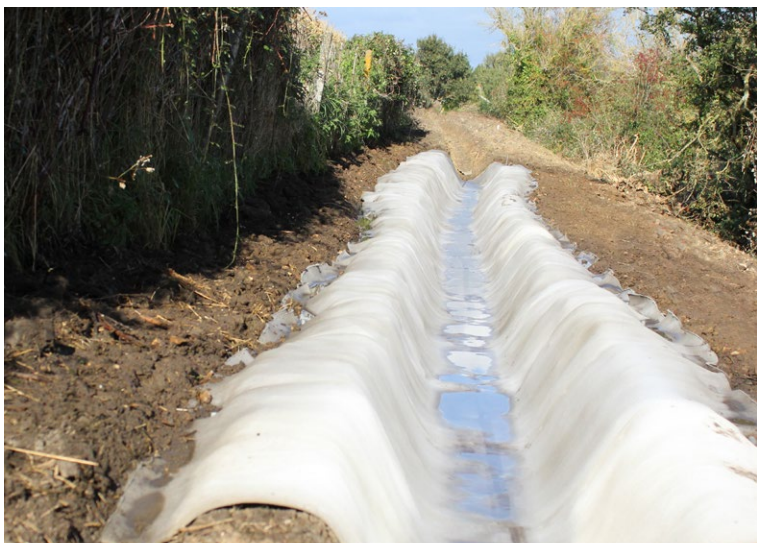
Section of new channel with hydrated CC8™
