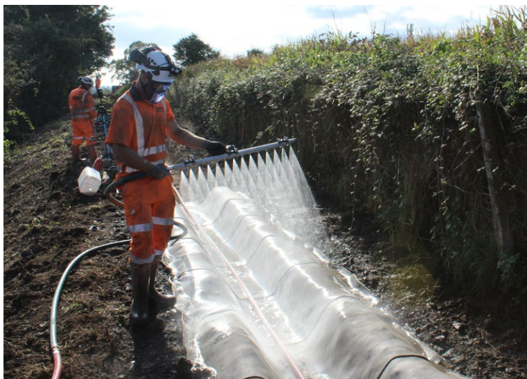
Sprinkler used to give CC8™ even hydration
