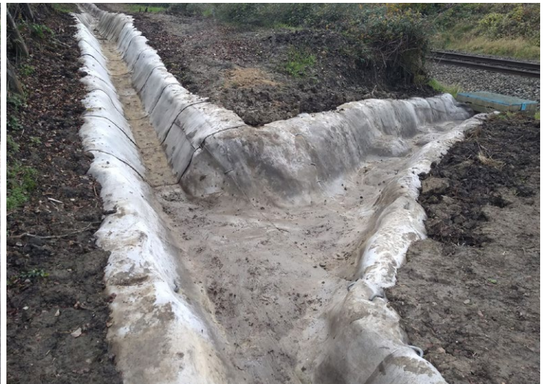
Channel/cascade junction detail
