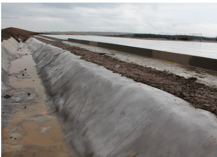
Anchor trenches were backfilled to prevent ingress
