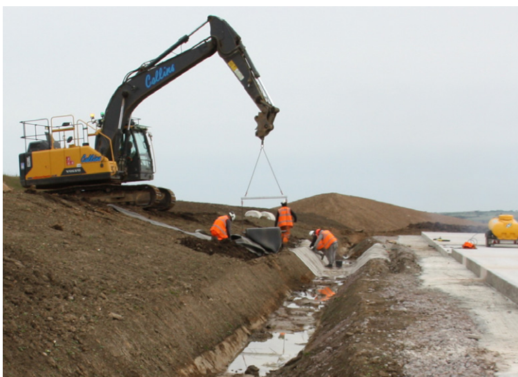
Bulk rolls of CC were mounted onto a spreader beam for installation
