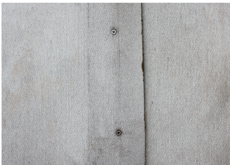
Stainless steel screws were used to fix overlaps
