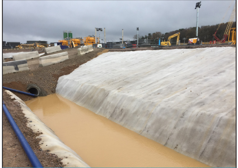
South pad termination detail
