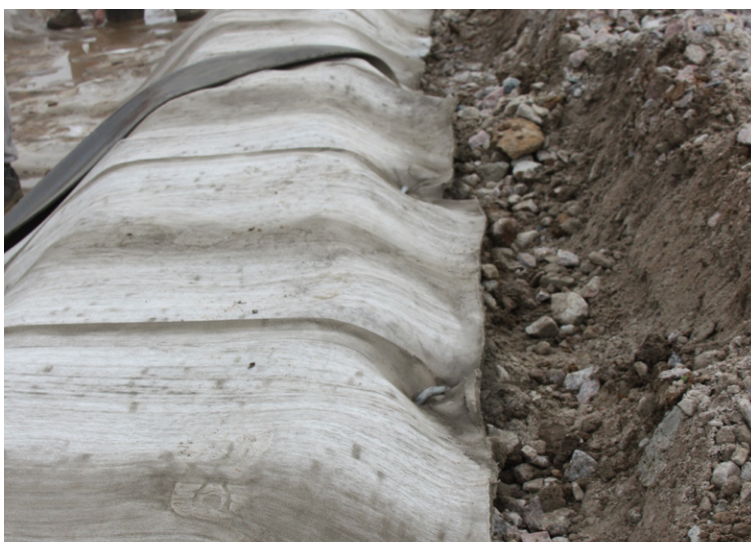
Edges of CC were secured in anchor trenches using ground
