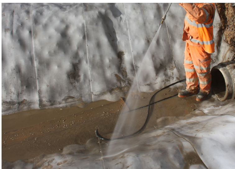
CC was hydrated following installation
