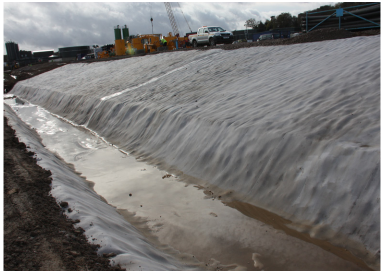
CC installed on slope and channel between North and Lower pads
