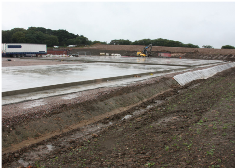
CC was laid transversely
