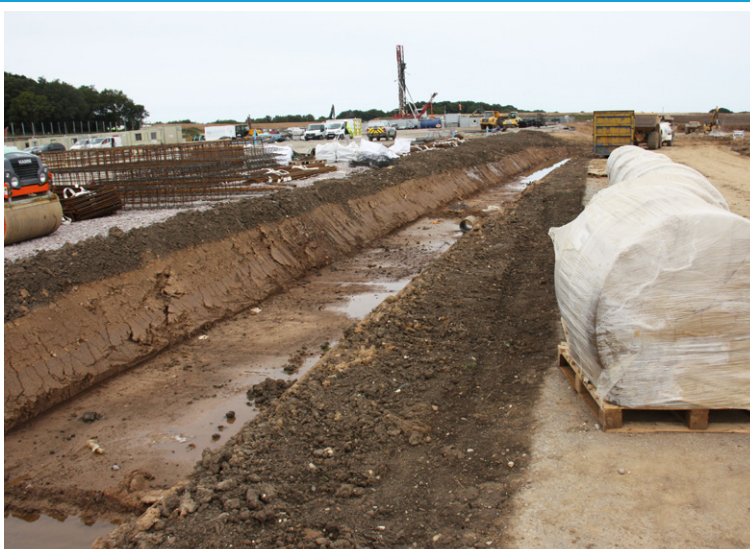
Bulk rolls of CC8™ were delivered to site prior to installation
