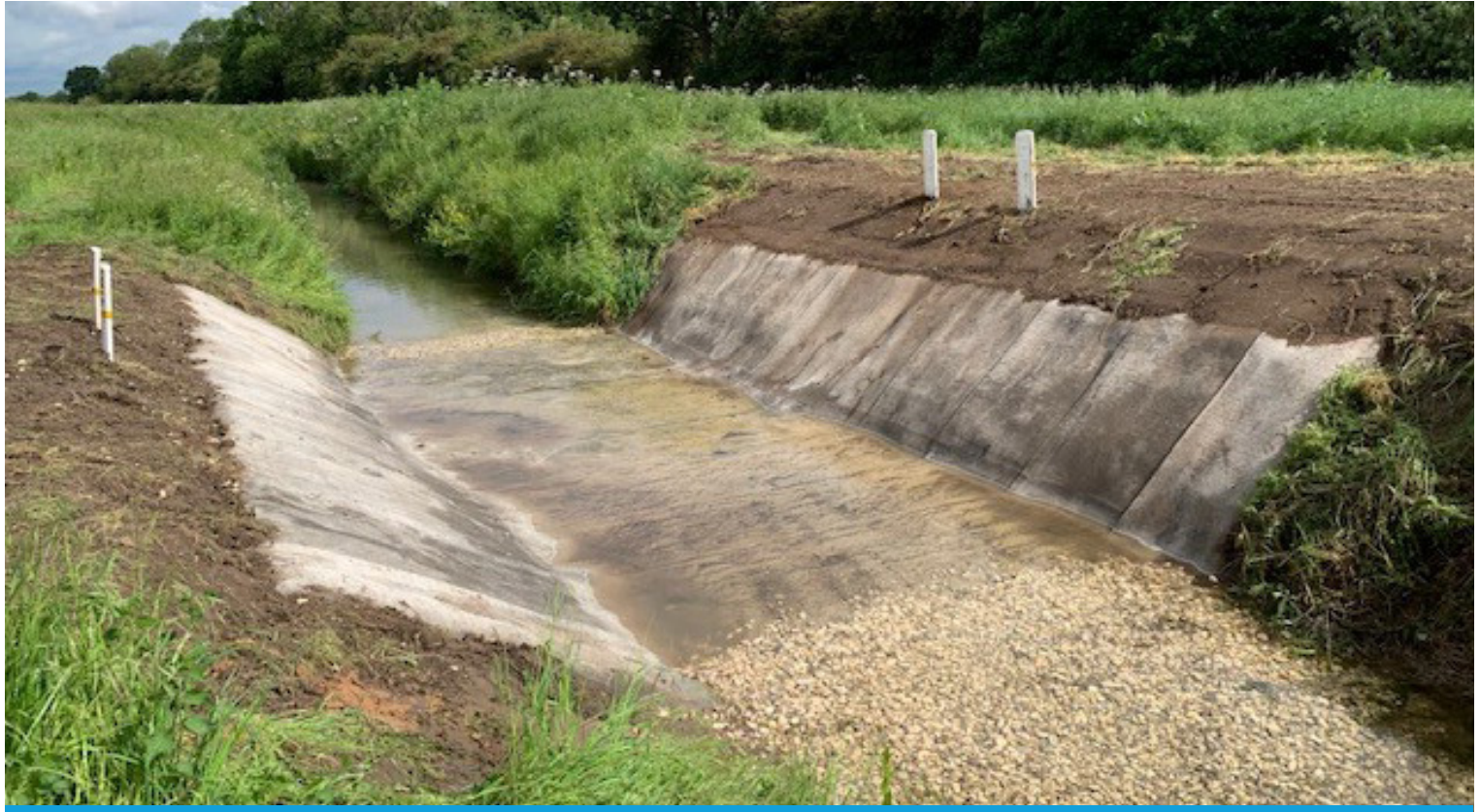
Completed channel lining installation for pipe protection
