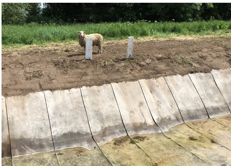
Anchor trenches backfilled following hydration
