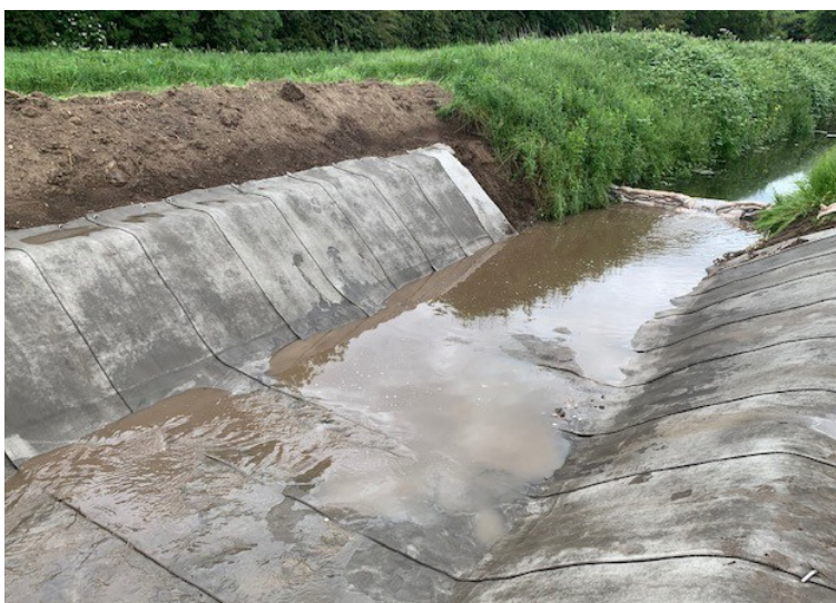
CC edges pinned within anchor trenches half way up the slopes
