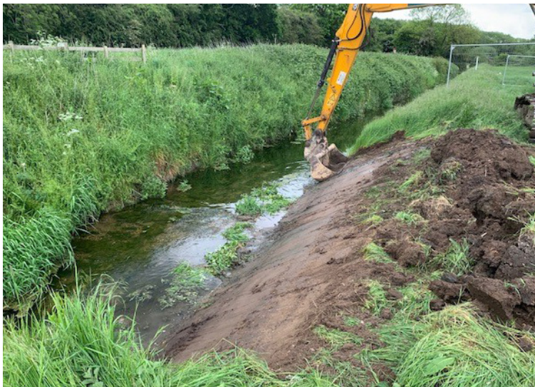
Grading of the channel banks
