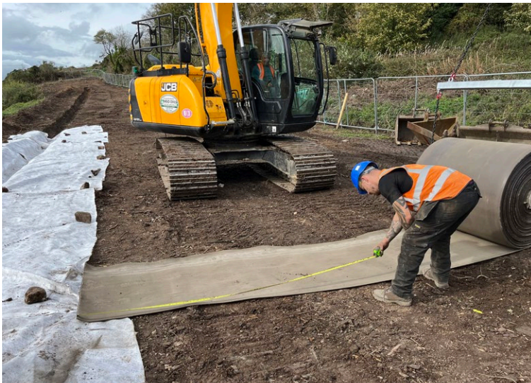
CCT2™ Measured prior to cutting
