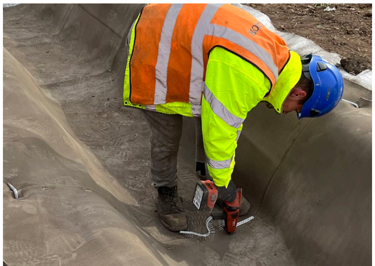
CCT2™ laid transversely & secured with 30mm stainless steel screws
