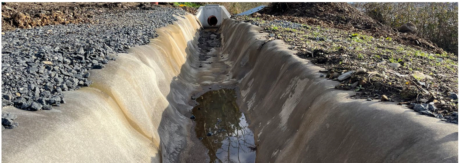
Channel terminated into precast headwall with 300mm pipe
