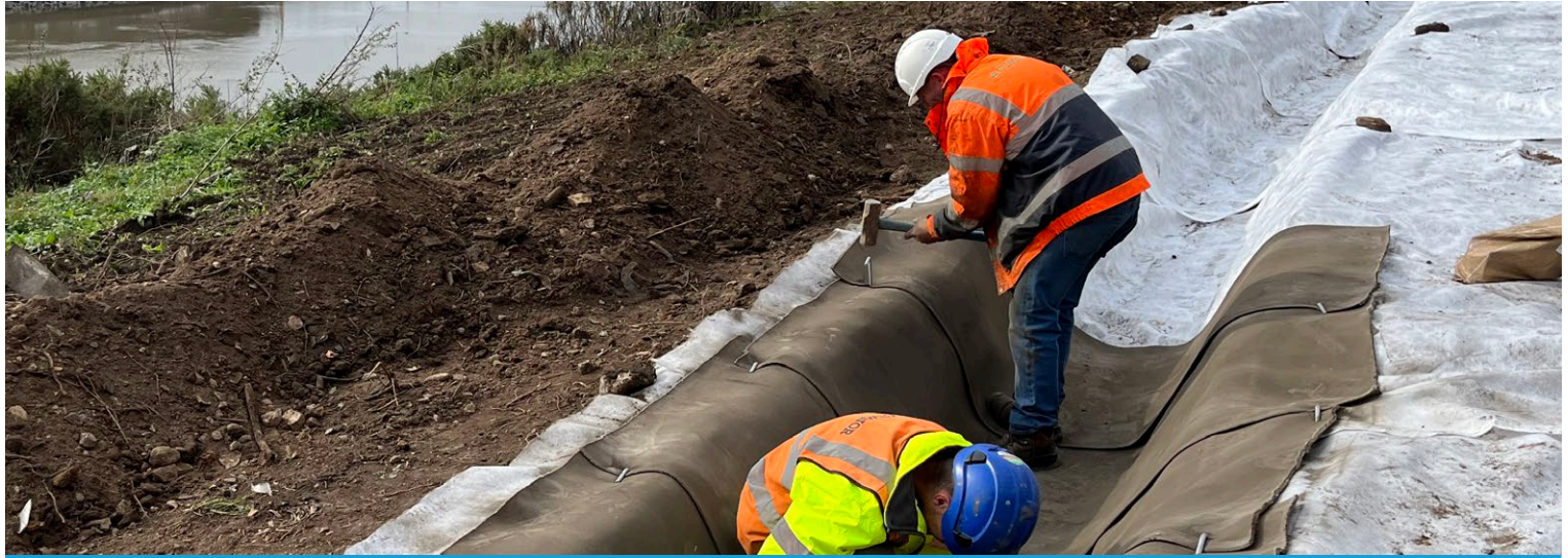
CCT2™ pegged into anchor trenches
