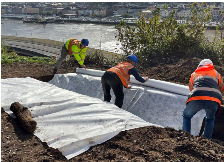
Non-woven geotextile laid into channel
