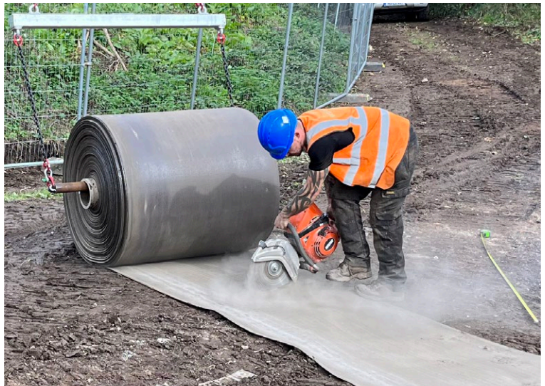
CCT2™ cut to desired length
