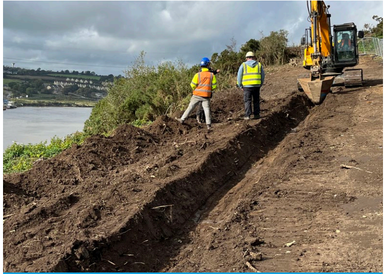
V-Bucket excavation
