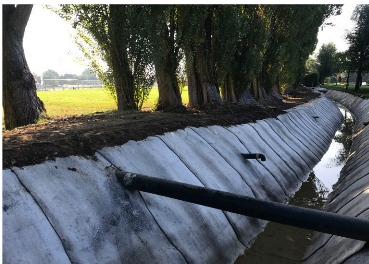
CC was cut to accomodate pipes and outfalls
