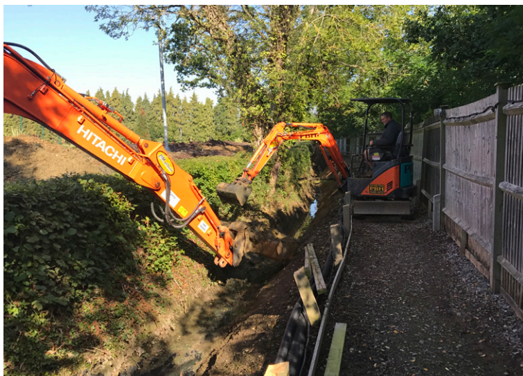
Excavators regraded the channel prior to installation
