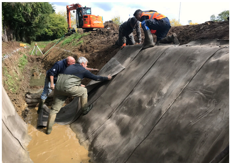
CC8 was laid transversely across the channel
