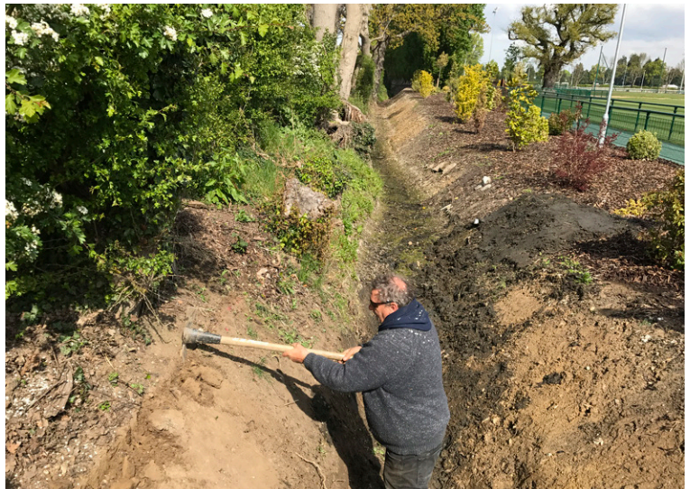
A pick-axe and shovel were used to regrade in restricted areas
