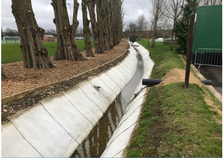
Outfall pipe and section of completed channel
