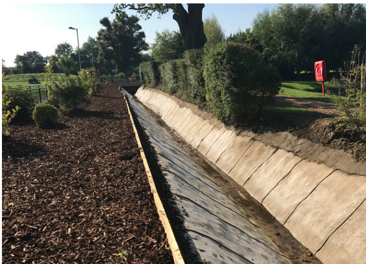
Edges were buried in soil anchor trenches or timber edging & bark chippings
