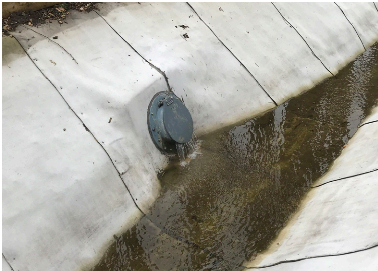
Capped outfall pipe covered with CC
