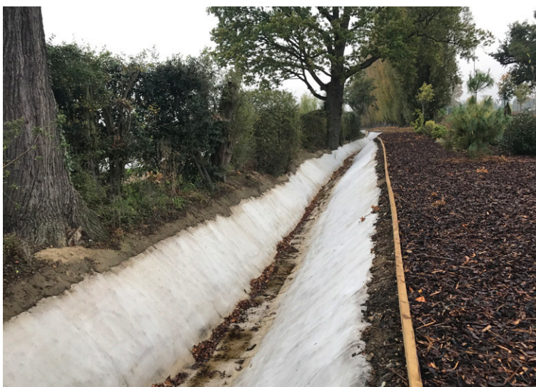
CC was jet washed after hydration to remove mud stains on surface
