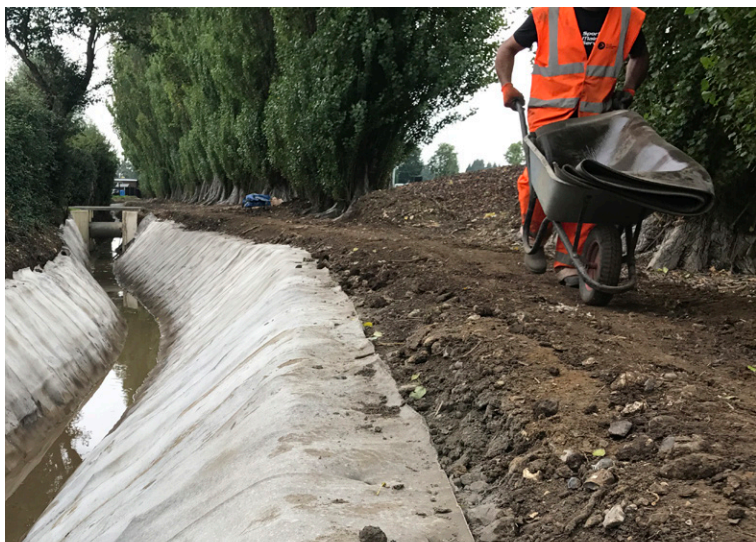
CC was batched and transported by wheelbarrow
