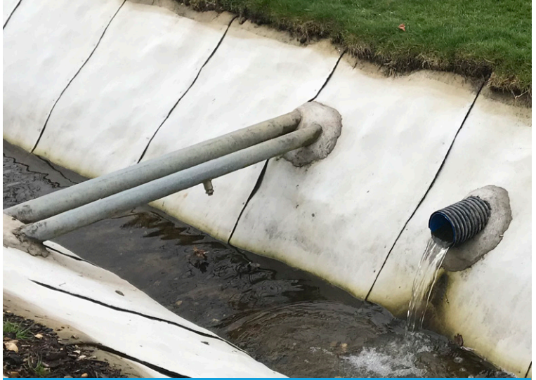
Sealed pipe detail, 9 months after installation
