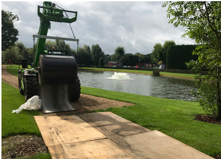
CC8 and CC13 Bulk rolls were batched on site
