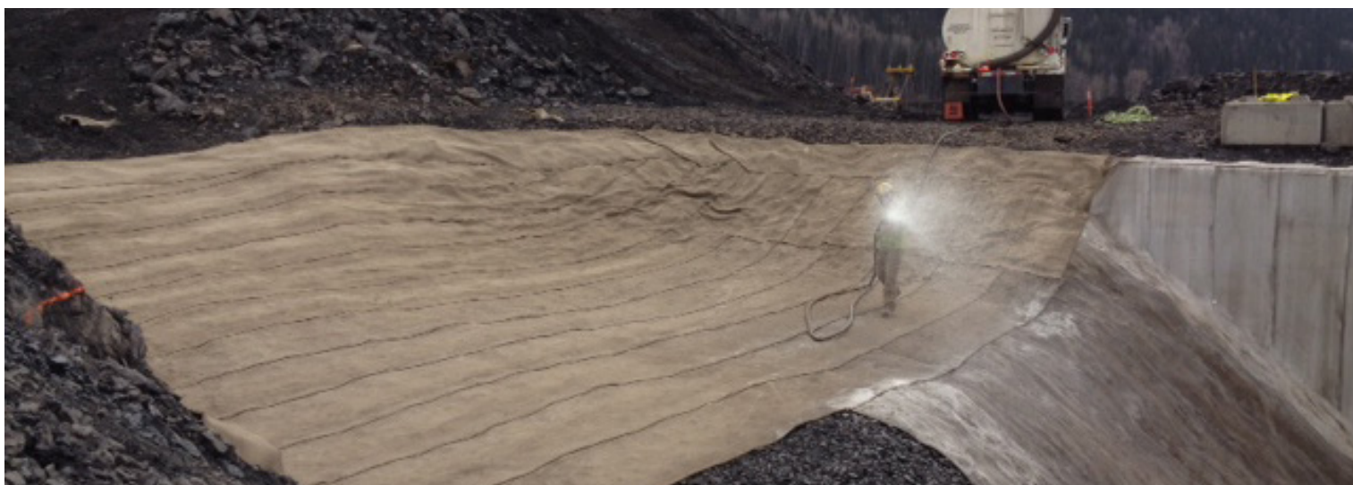
Hydration of top section of carrier channel
