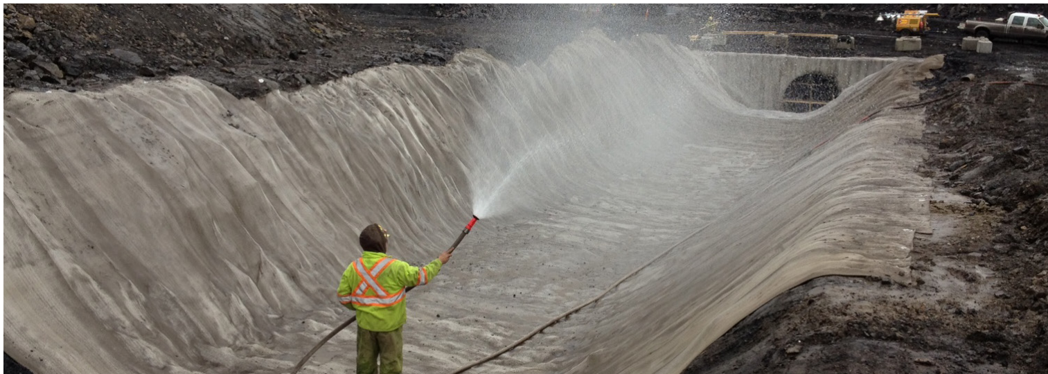
Hydration of lower channel section
