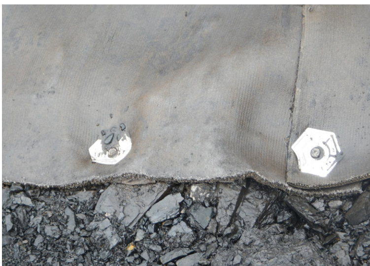
6" steel anchor nails with 1" hex head washers
