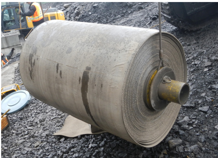
CC bulk rolls dispensed using spreader beam and plant
