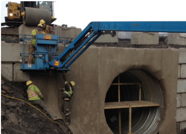
Lining culvert with CC8™
