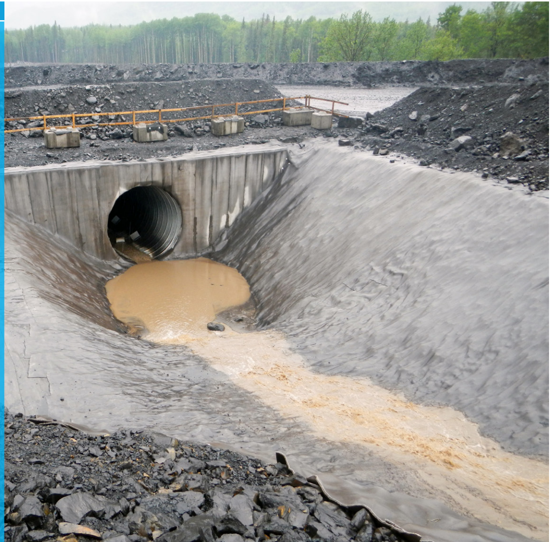
Completed lined channel and culvert
