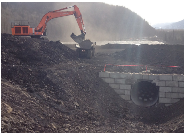
Excavating sump and constructing culvert
