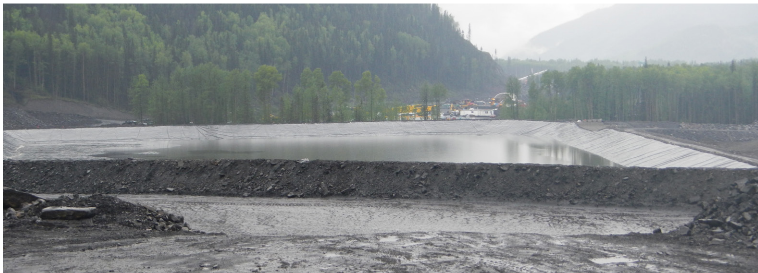
Large settling pond collecting effluent from nearby Willow Creek mine
