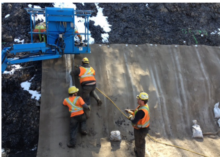
Applying SikaFlex beading to joints
