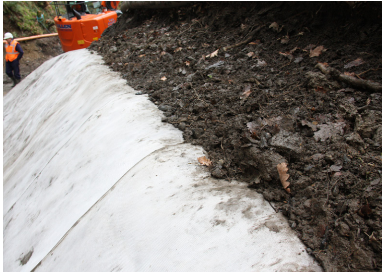
Backfilled anchor trench
