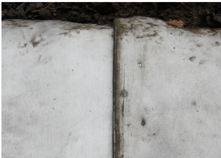
Stainless steel screws were used to joint CC overlaps
