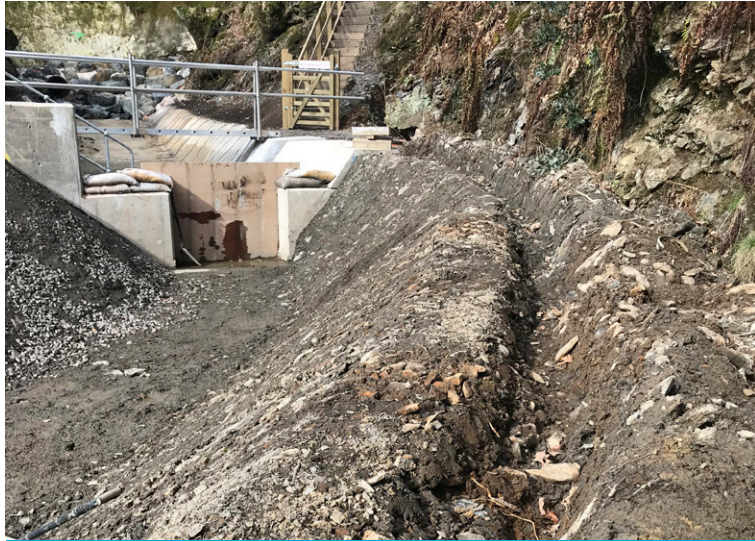
Channel following regrading, profiling and creation of anchor
