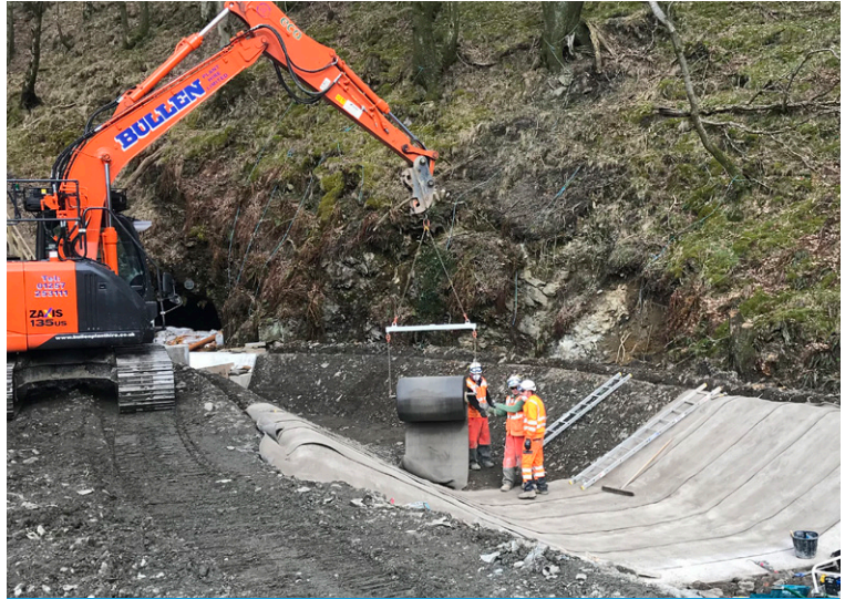
CC was deployed from a spreader beam and digger and laid transversely
