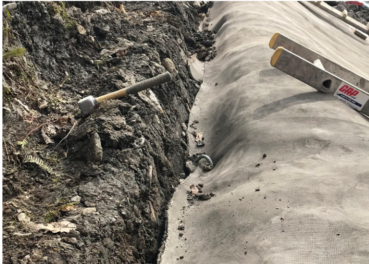
Ground pegs were used to secure CC edges in anchor trenches
