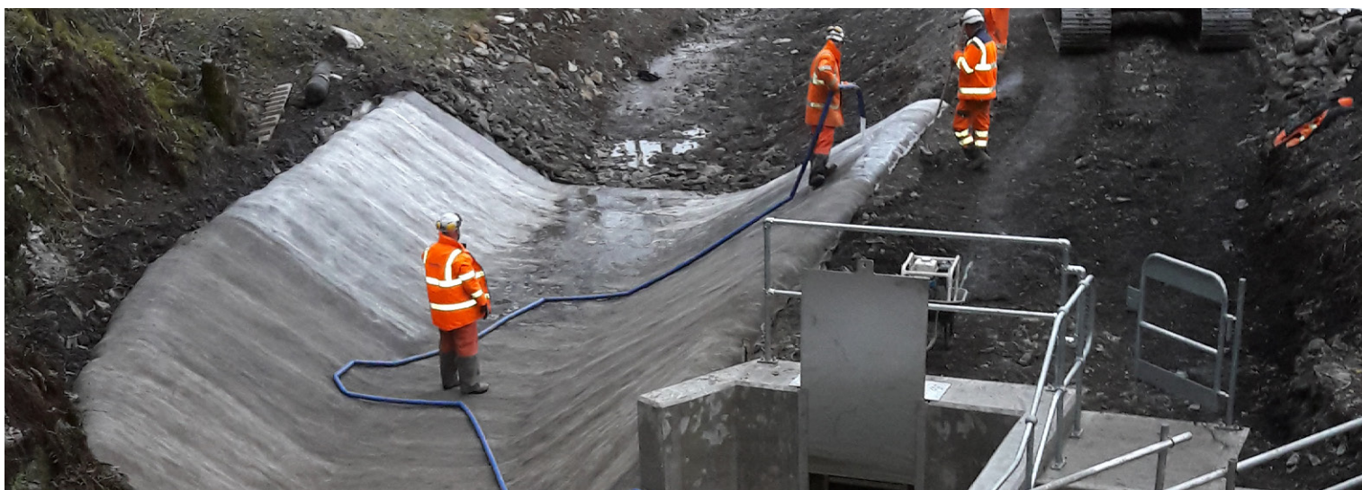
Hydration was given at the end of each day using water from the dam
