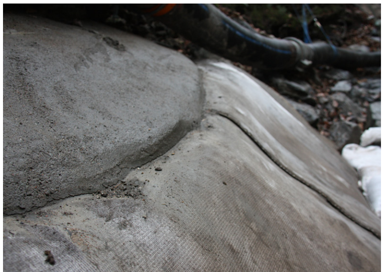
CC edges sealed using poured concrete instead of anchor trenches
