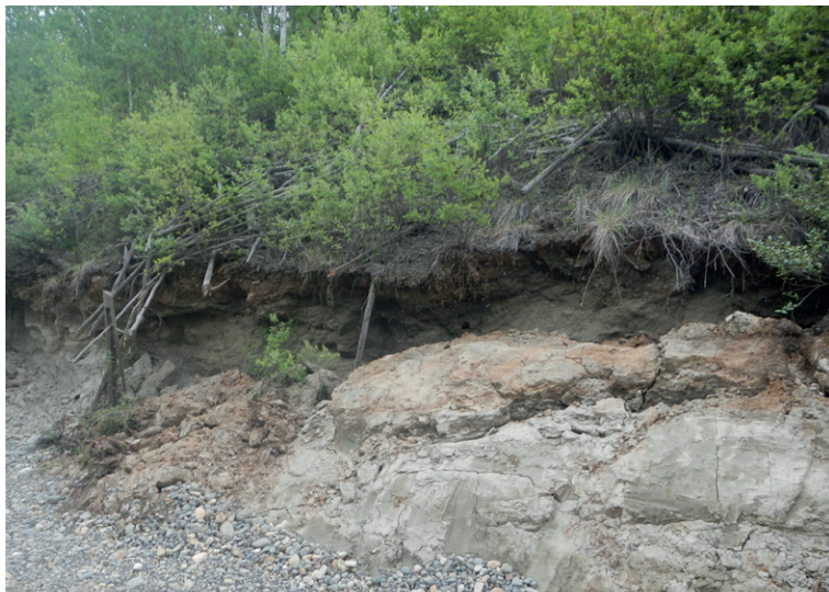
Condition of slope prior to installation
