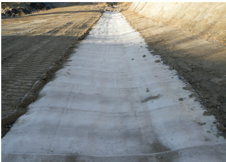
Completed channel trial installation
