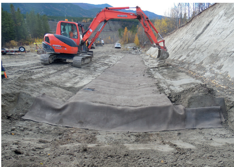
CC edges were captured in a large anchor trench which was later backfilled
