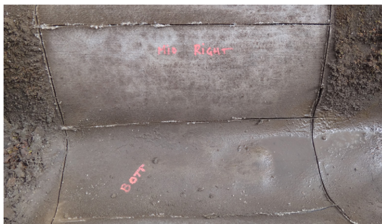
Fig. 4: Channel section after cutting
