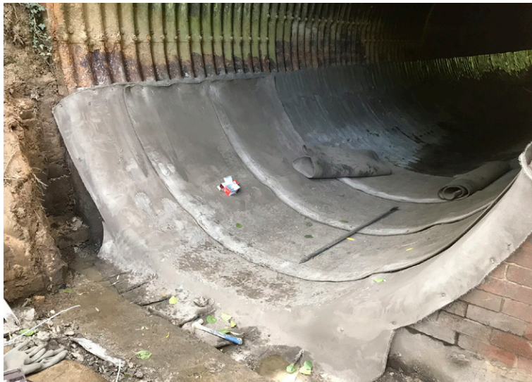
Installing first layers of CC
