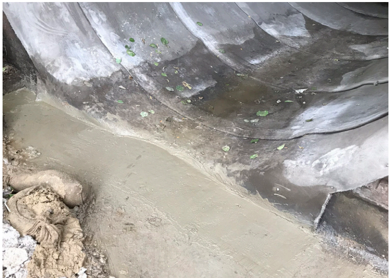
Edge of CC secured to archway and buried with poured concrete
