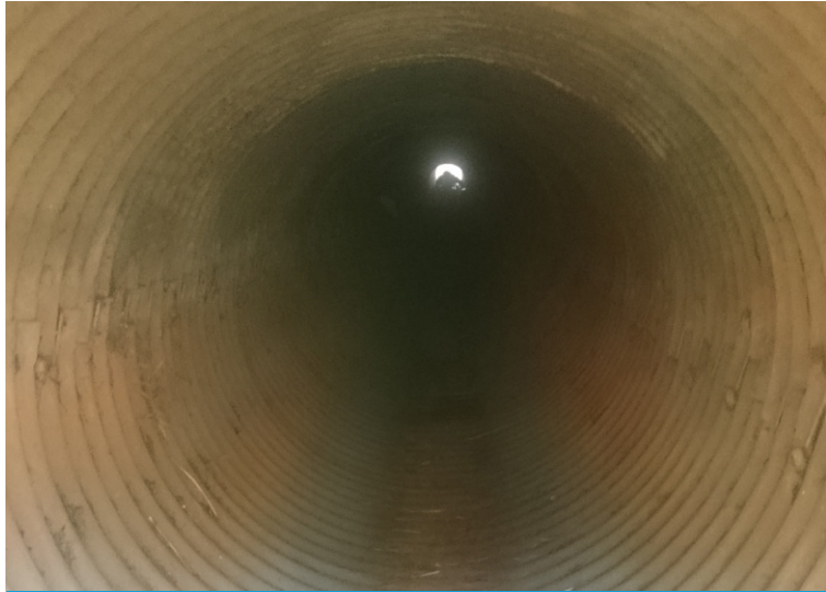
Existing corrugated steel culvert
