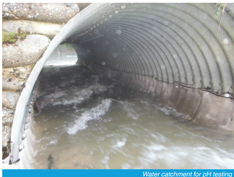
CC post-installation, prior to trimming and sealing of edges
