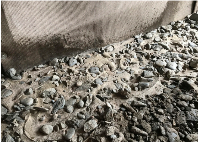
Grout & stones applied to CC floor to provide rocky surface for fish
