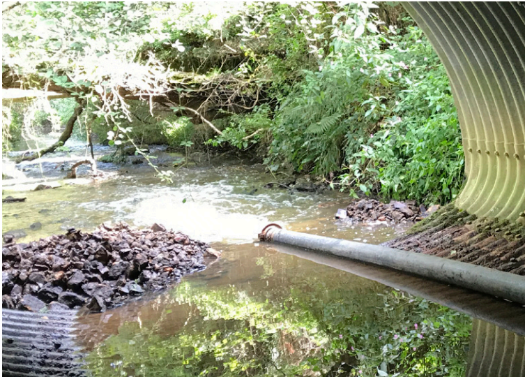
Water redirected using overpumping
