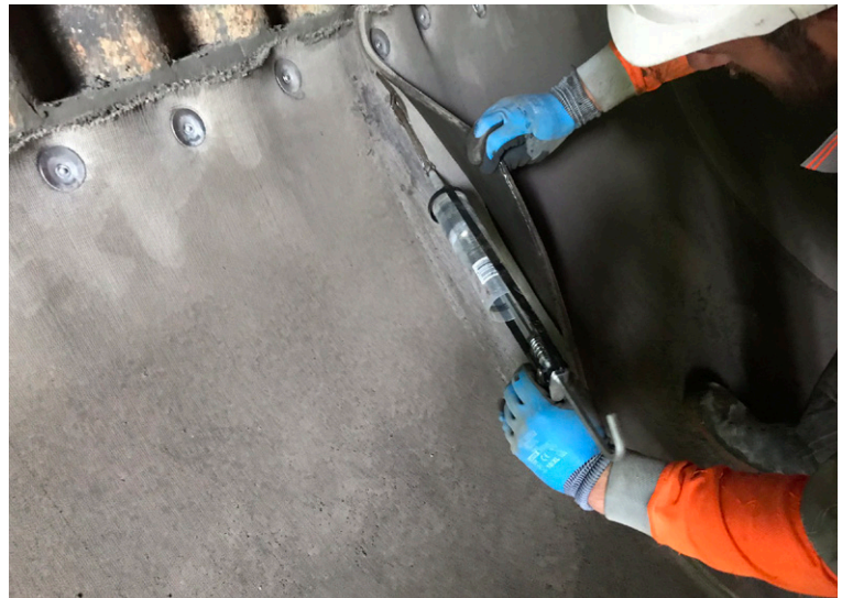
Hilti shot-fired nails used to fix CC to culvert before sealing joints
