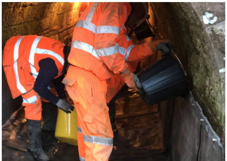
Hydration of CC on walls
