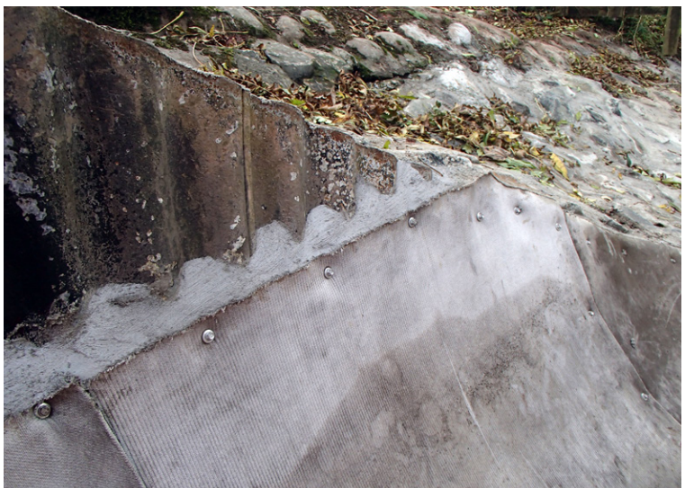
CC was fixed with tech screws & grout applied to prevent water ingress
