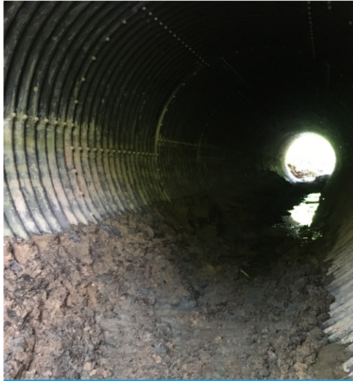
Thick silt build up in culvert 1
