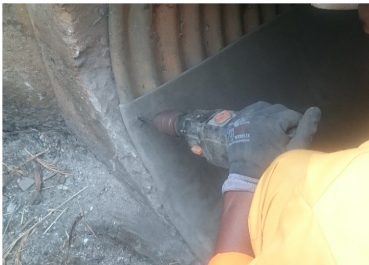
Fixing with pop rivets
