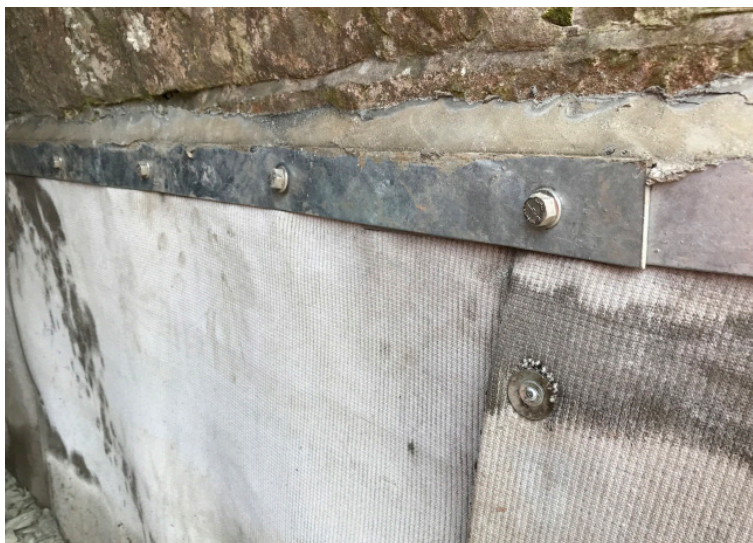
Shot-fired nails, steel bars and grout used for fixing and termination
