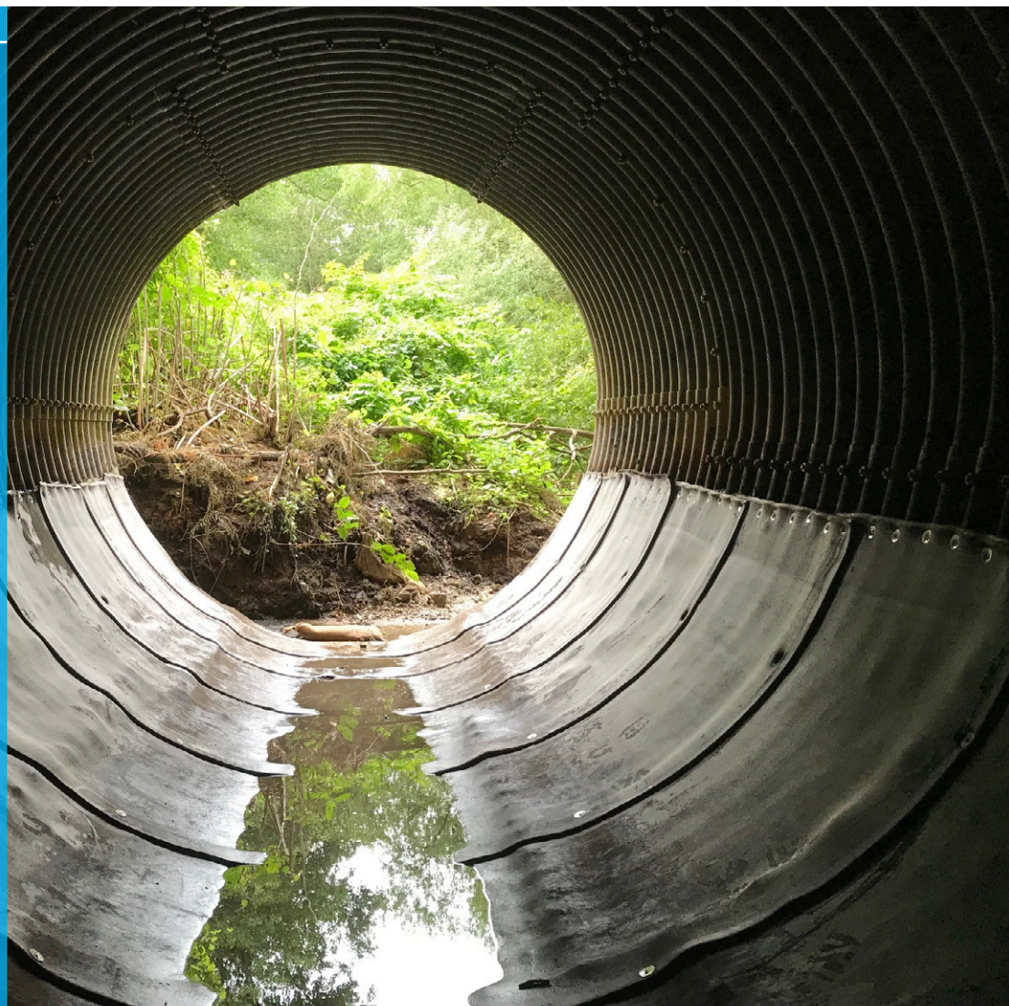
Completed CC culvert lining installation
