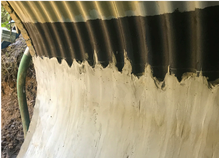
Inverts filled with concrete mortar following cleaning
