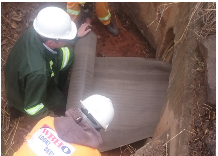
Laying CC5™ lengths in culvert
