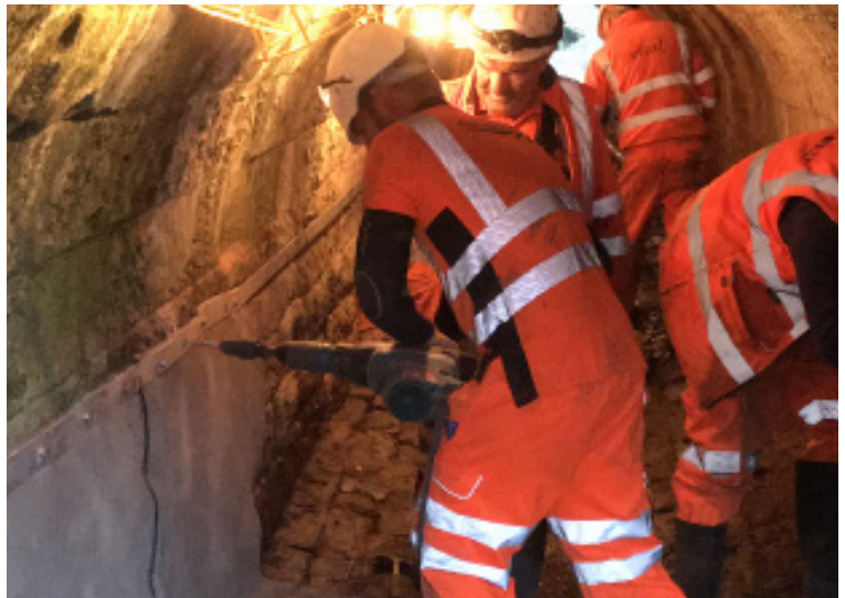
Fixing CC to masonry wall
