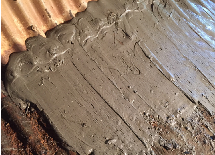
The grout provided a flat surface to lay the CC on top of
