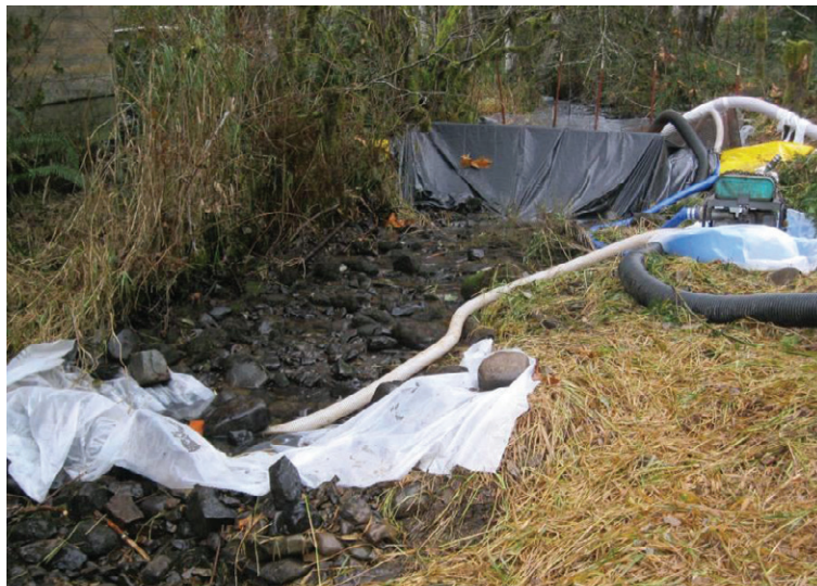
Isolating with cofferdams and de-watering the site
