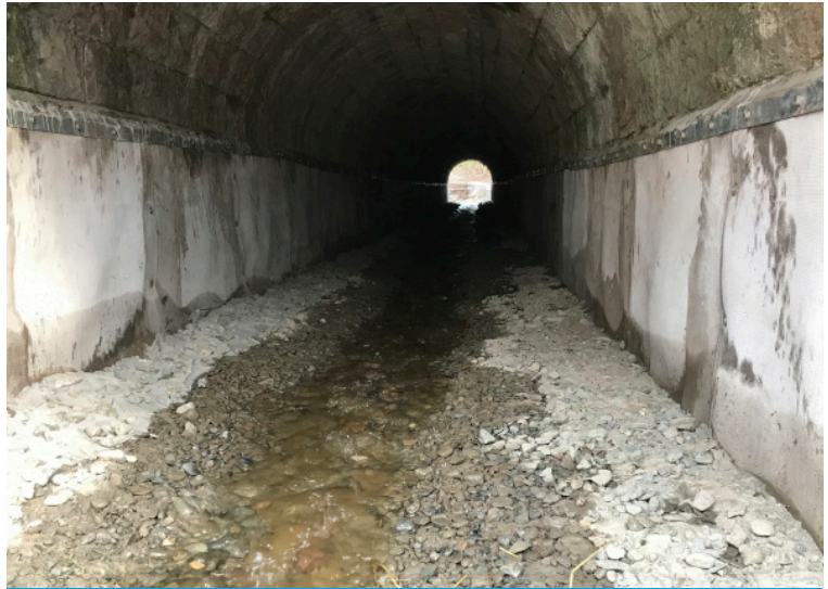
Completed installation, with additional stone floor
