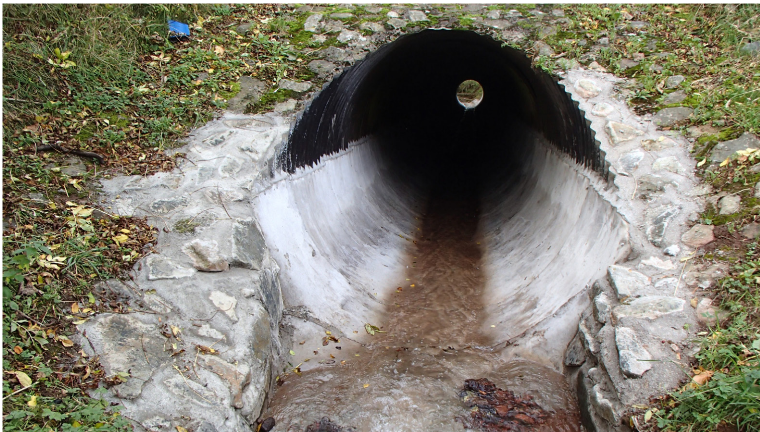
Completed relined culvert on upstream side
