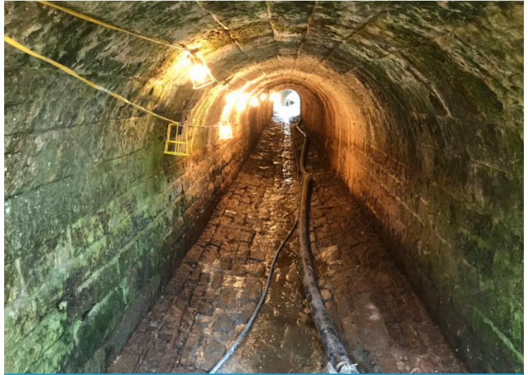
Culvert prior to works - water overpumped to allow installation
