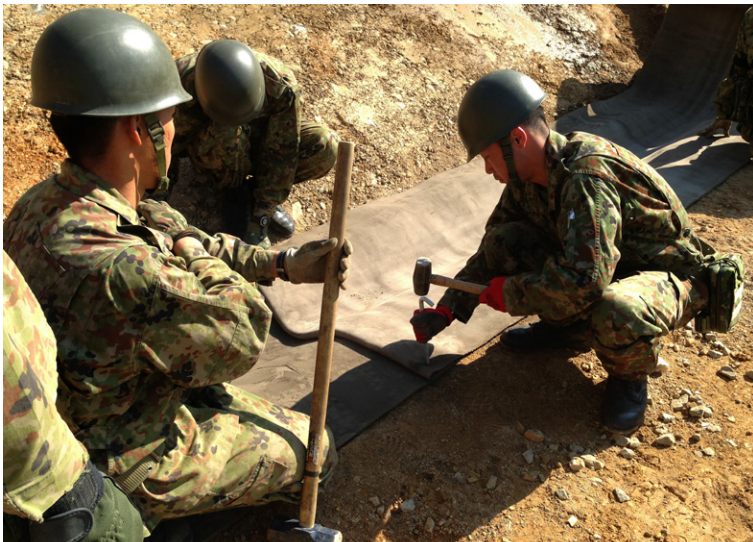
Ground pegs were inserted through knuckle joints
