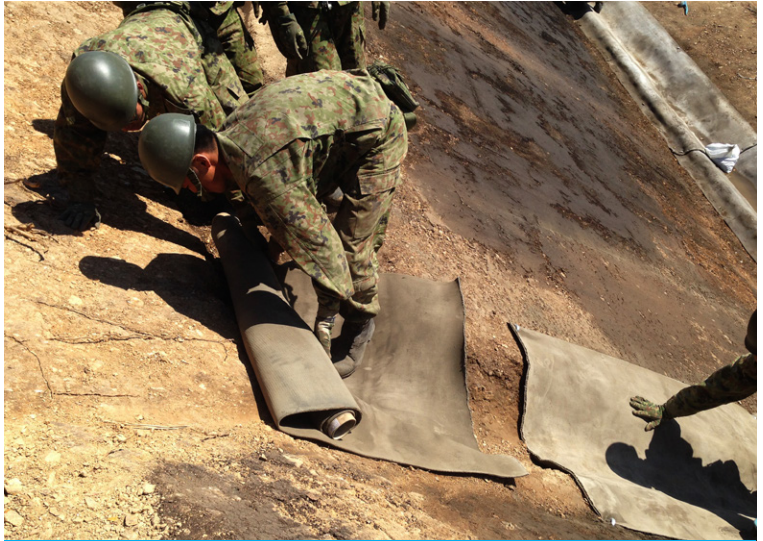
The CC was laid longitudinally
