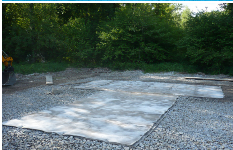
Hydrated CC allowed to set for 2 hours
