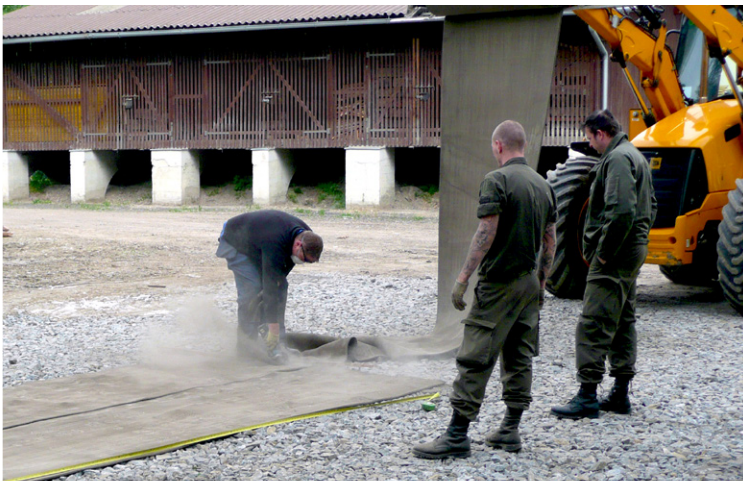
Cutting CC onsite using powered disc cutter
