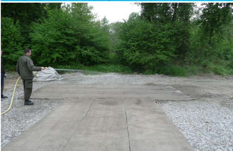
Hydrating the first CC layer, prior to installing the second
