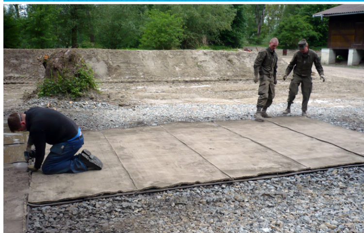
CC layers were screwed together using standard wood screws
