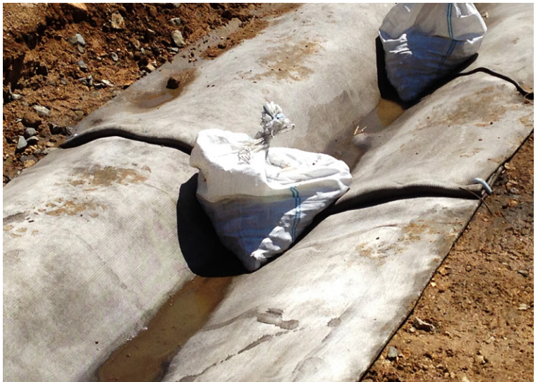
A knuckle joint pegged, screwed and weighed down whilst setting
