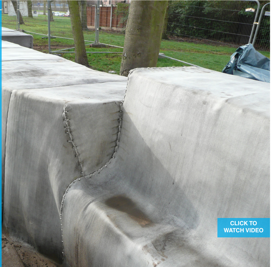
Completed CC-lined gabion
