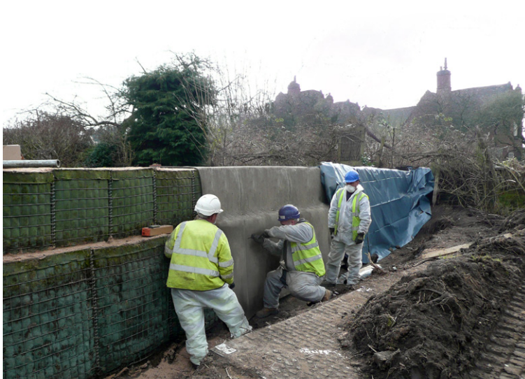
Fixing CC to gabion structures using re-bar staples
