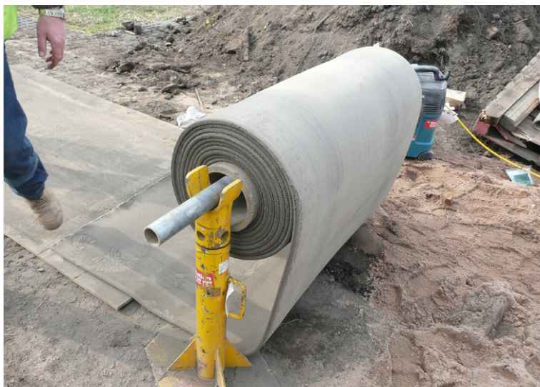
Dispensing 20m pre-cut rolls of CC13 on site before cutting to length
