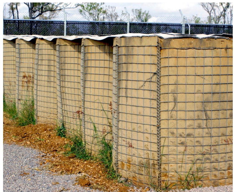
CC cap provides protection from inclement weather and high winds
