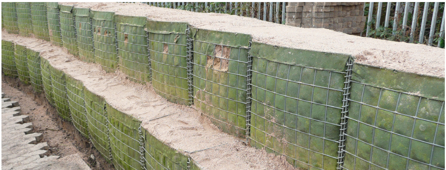
Degraded gabion flood defences, damaged from weathering and vandalism
