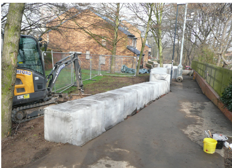
Completed CC lined gabion section
