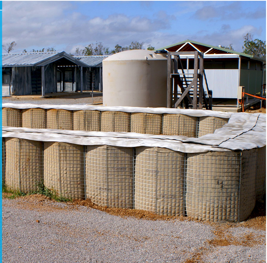
Completed gabion capping
