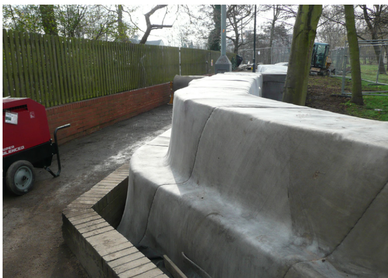
Hydrated CC prior to backfilling toe anchor trench
