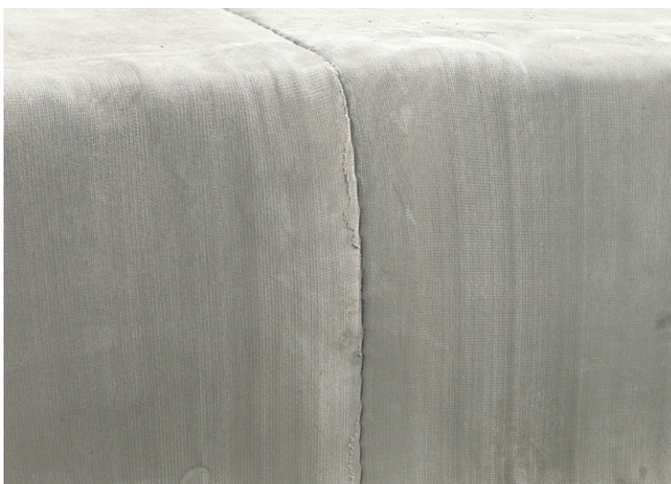
Flush seamed joints between hog ringed CC layers
